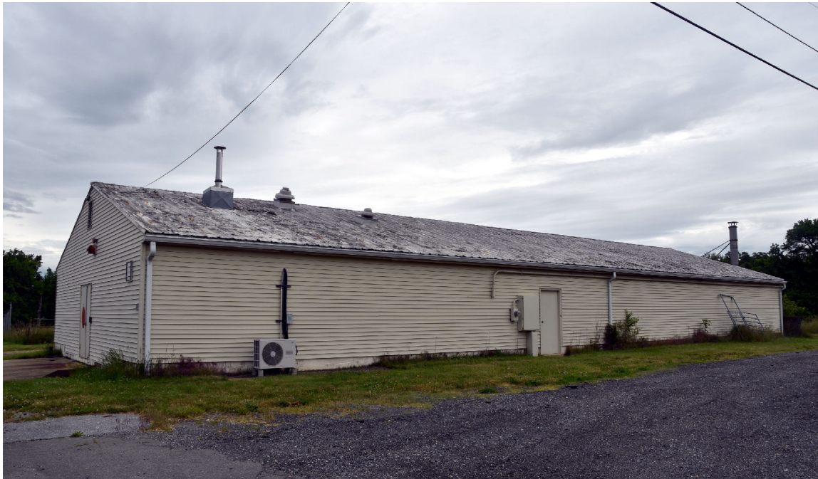
Photo 2 - Building 204B, Central Farm, View of South Elevation, Looking Northeast
