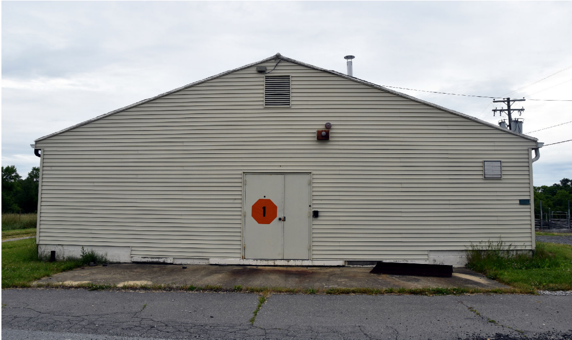
Photo 1 - Building 204B, Central Farm, View of West Elevation, Looking East
