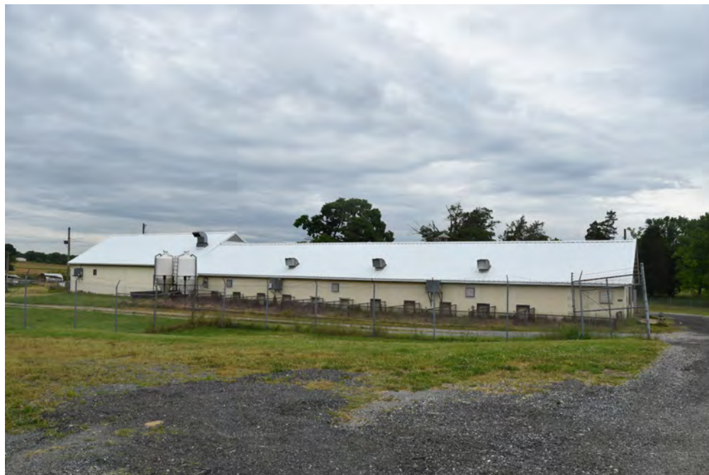
Photo 1 - Building 208, Swine Feed Barn & Farrowing Facility, Central Farm, View of South Elevation, Looking North
