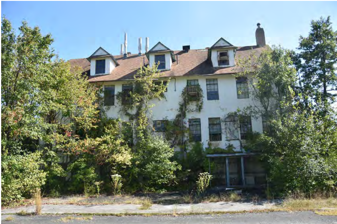
Photo 3 – Building 264, Poultry Laboratory Building, Central Farm, View of West Elevation, Looking East
