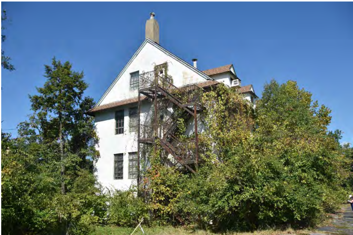
Photo 2 – Building 264, Poultry Laboratory Building, Central Farm, View of South Elevation, Looking Northwest
