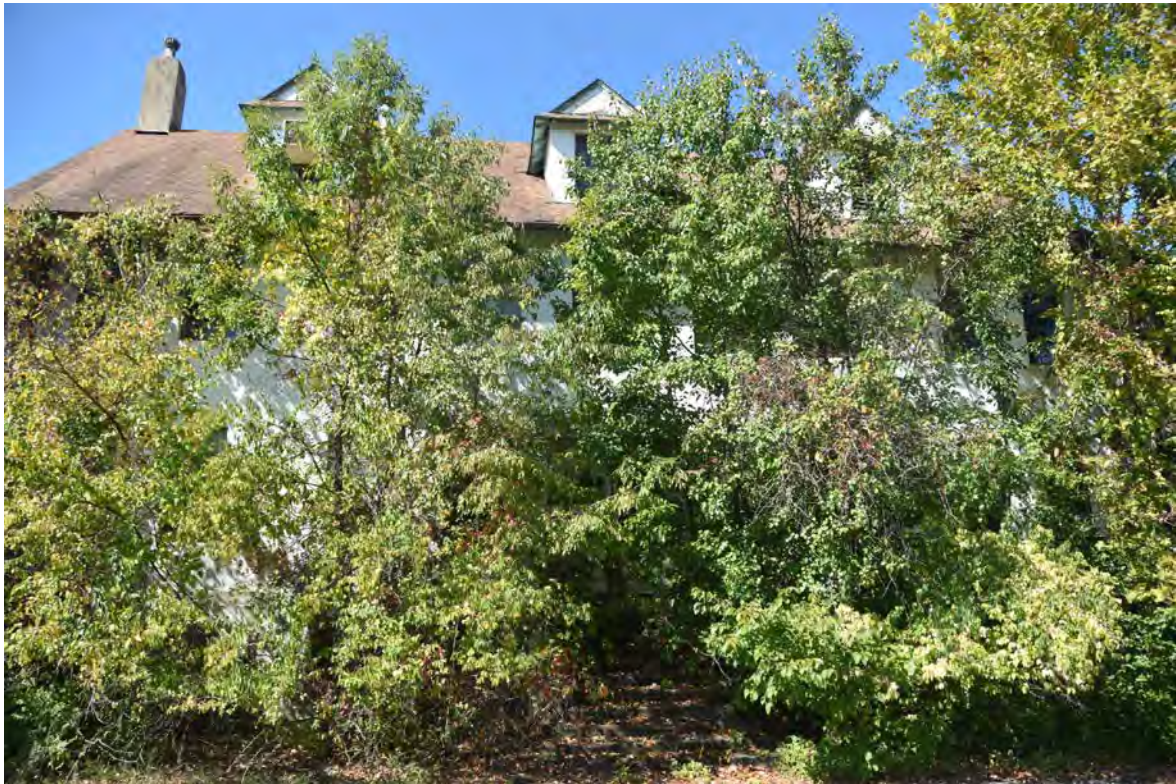
Photo 1 – Building 264, Poultry Laboratory Building, Central Farm, View of East Elevation, Looking West
