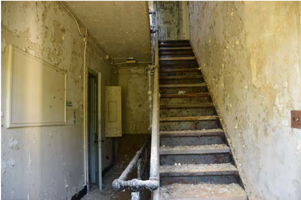
Photo 4 – Building 265, Biological Poultry Lab, Central Farm, View of First Floor Hall, Looking West
