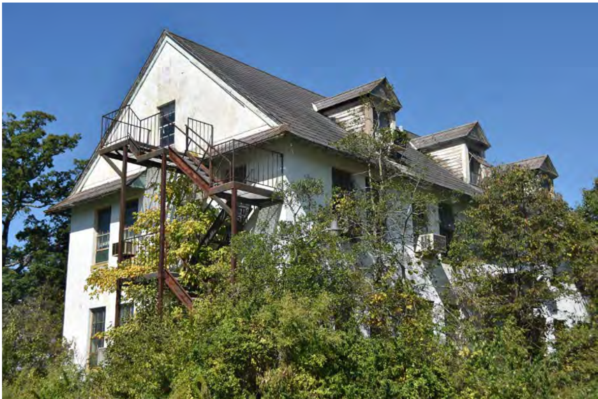
Photo 2 – Building 265, Biological Poultry Lab, Central Farm, View of East and South Elevations, Looking Northwest
