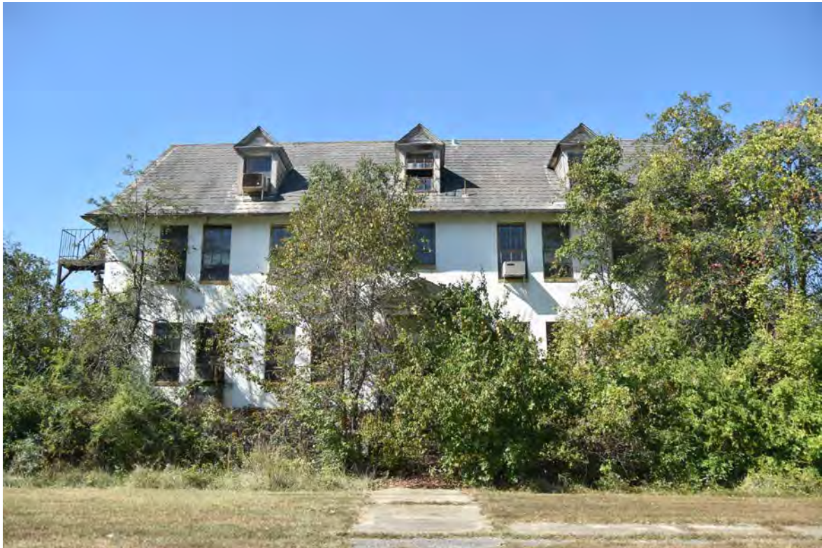
Photo 1 – Building 265, Biological Poultry Lab, Central Farm, View of East Elevation, Looking West
