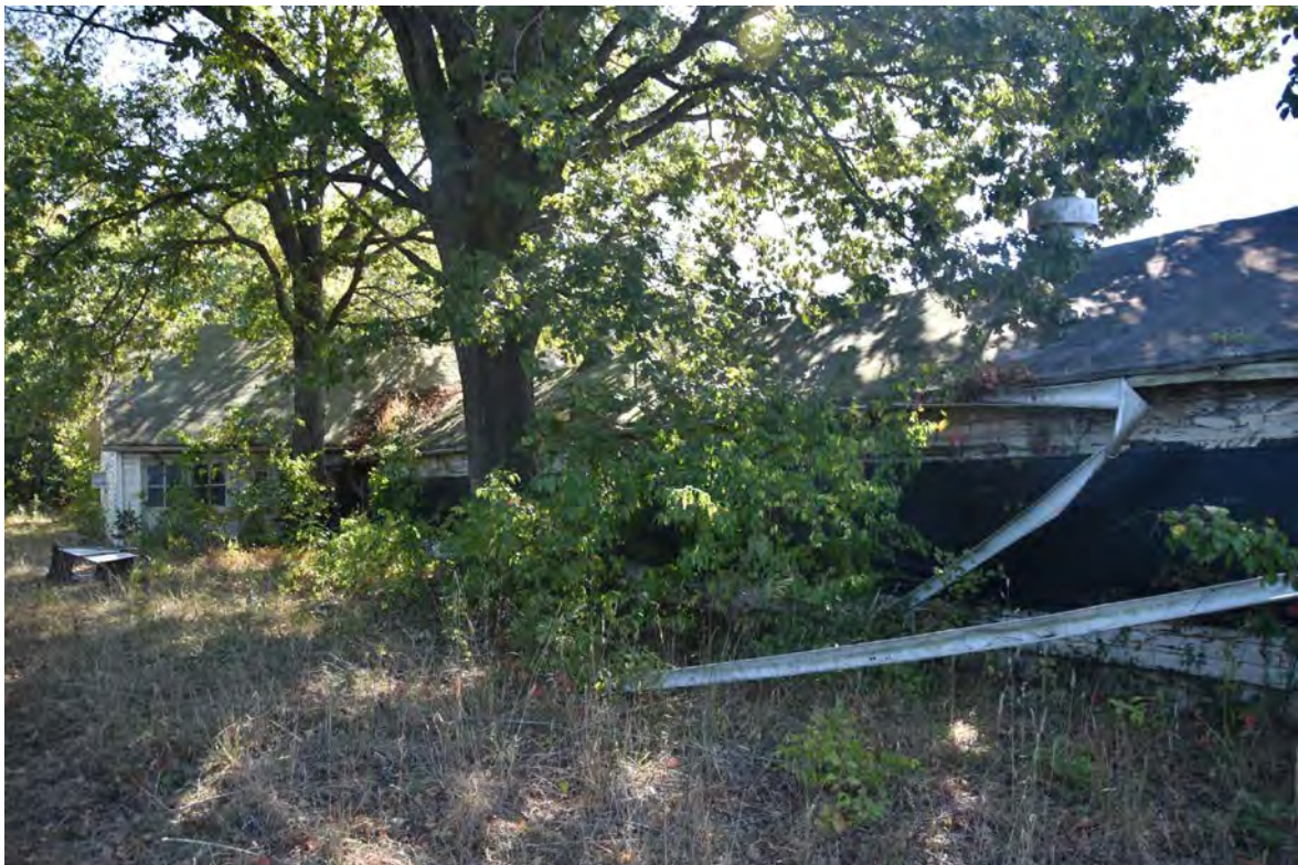
Photo 4 – Building 267, Turkey Brooder and Feed House, Central Farm, View of North Elevation, Looking Southeast
