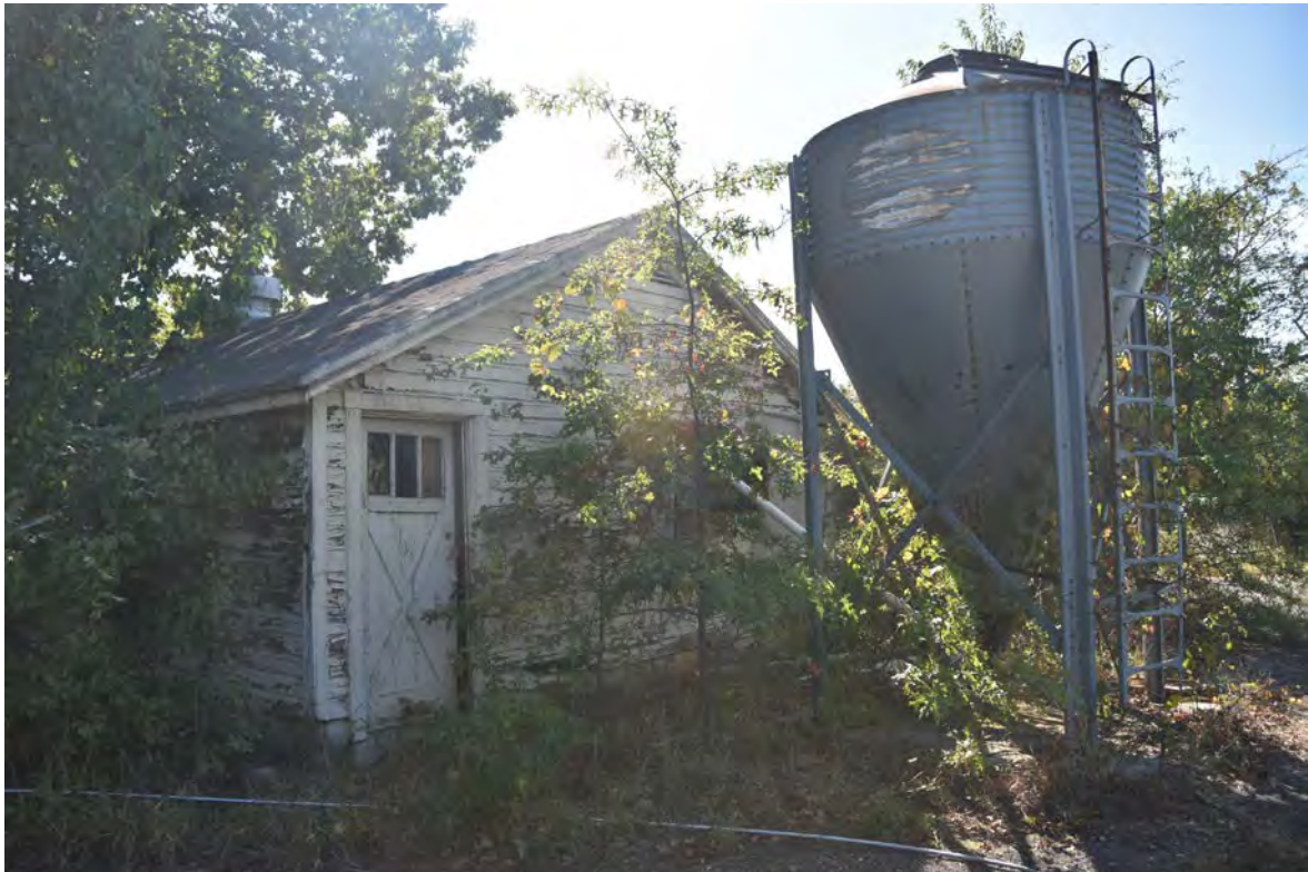
Photo 3 – Building 267, Turkey Brooder and Feed House, Central Farm, View of West Elevation, Looking Southeast
