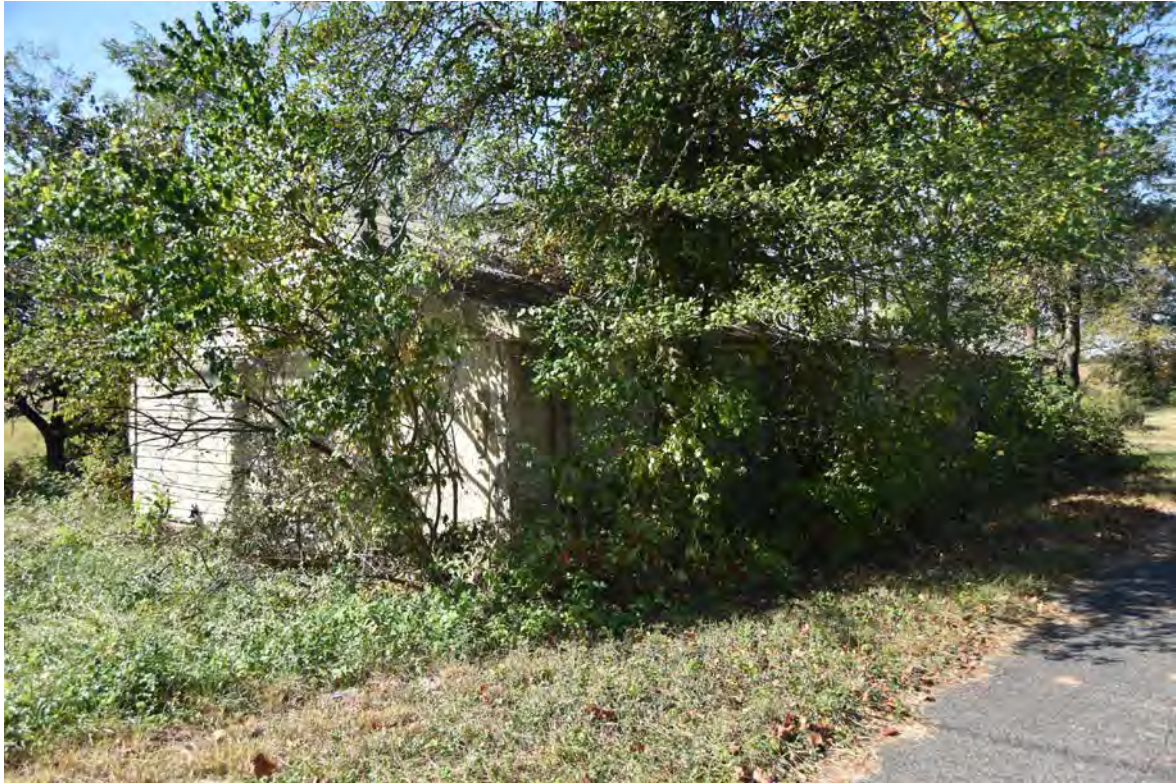
Photo 1 – Building 270, Turkey Mating and Breeding House, Central Farm, View of East and North Elevations, Looking Southwest
