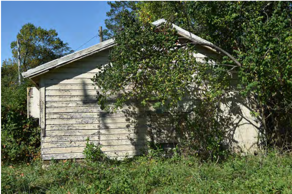
Photo 2 – Building 270, Turkey Mating and Breeding House, Central Farm, View of East Elevation, Looking West
