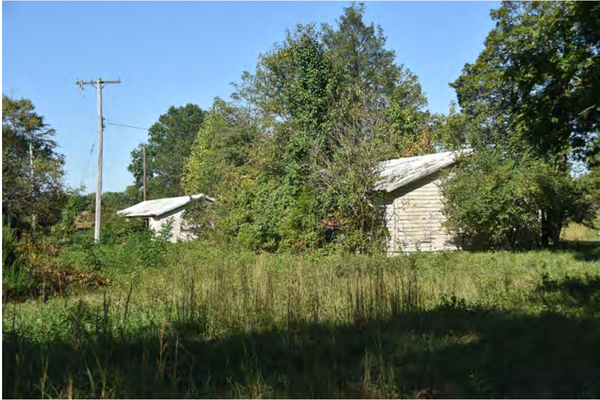
Photo 3 – Building 271, Turkey Mating and Breeding House, Central Farm, View of South and East Elevations, Looking Northwest
