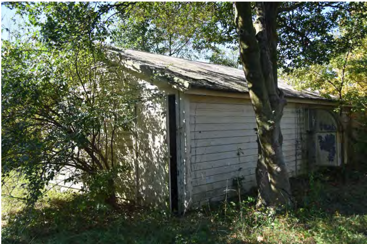
Photo 2 – Building 271, Turkey Mating and Breeding House, Central Farm, View of East and North Elevations, Looking Southwest
