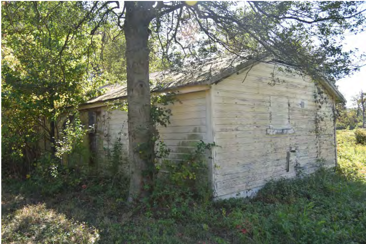
Photo 1 – Building 271, Turkey Mating and Breeding House, Central Farm, View of North and West Elevations, Looking Southeast
