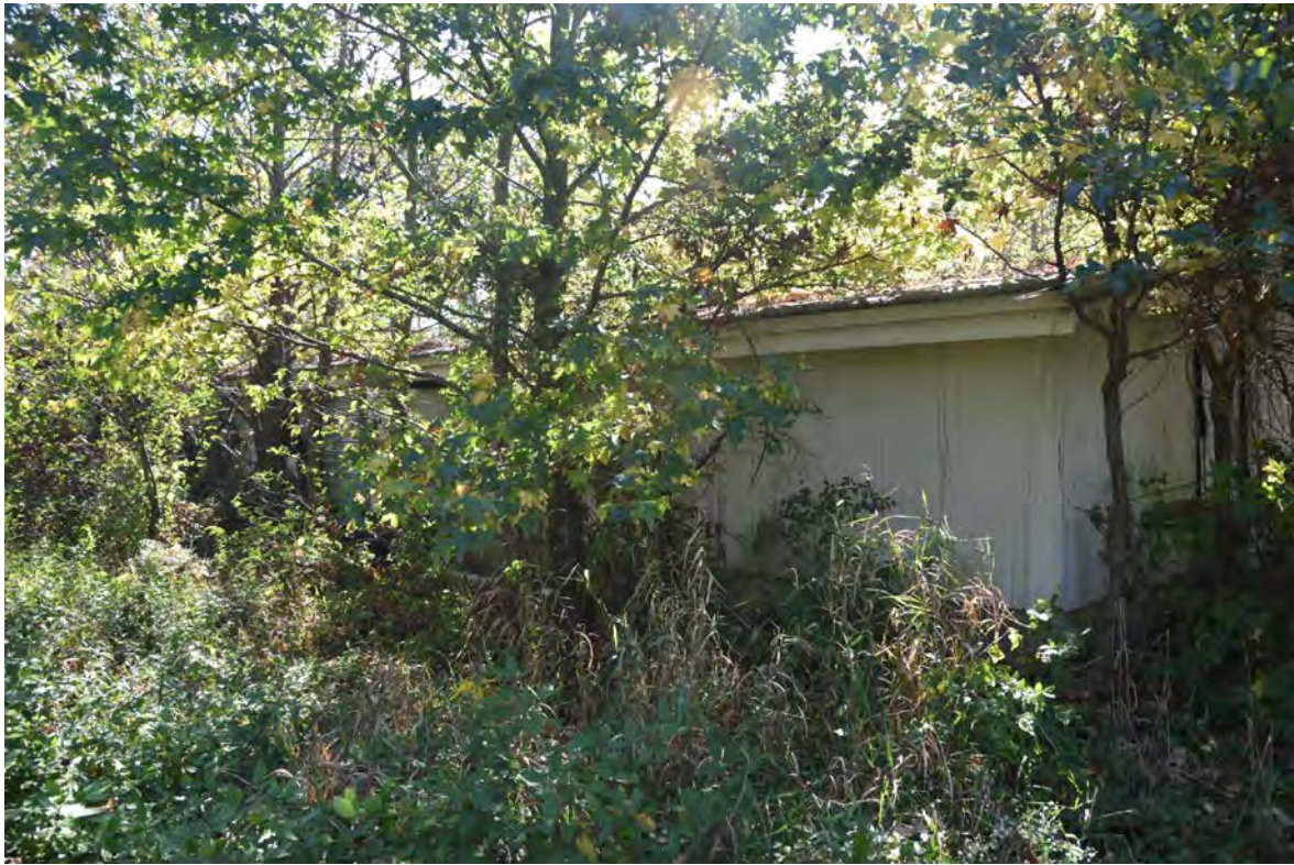
Photo 3 – Building 273, Experimental Laying House for Breeding, Central Farm, View of West and North Elevations, Looking Southeast
