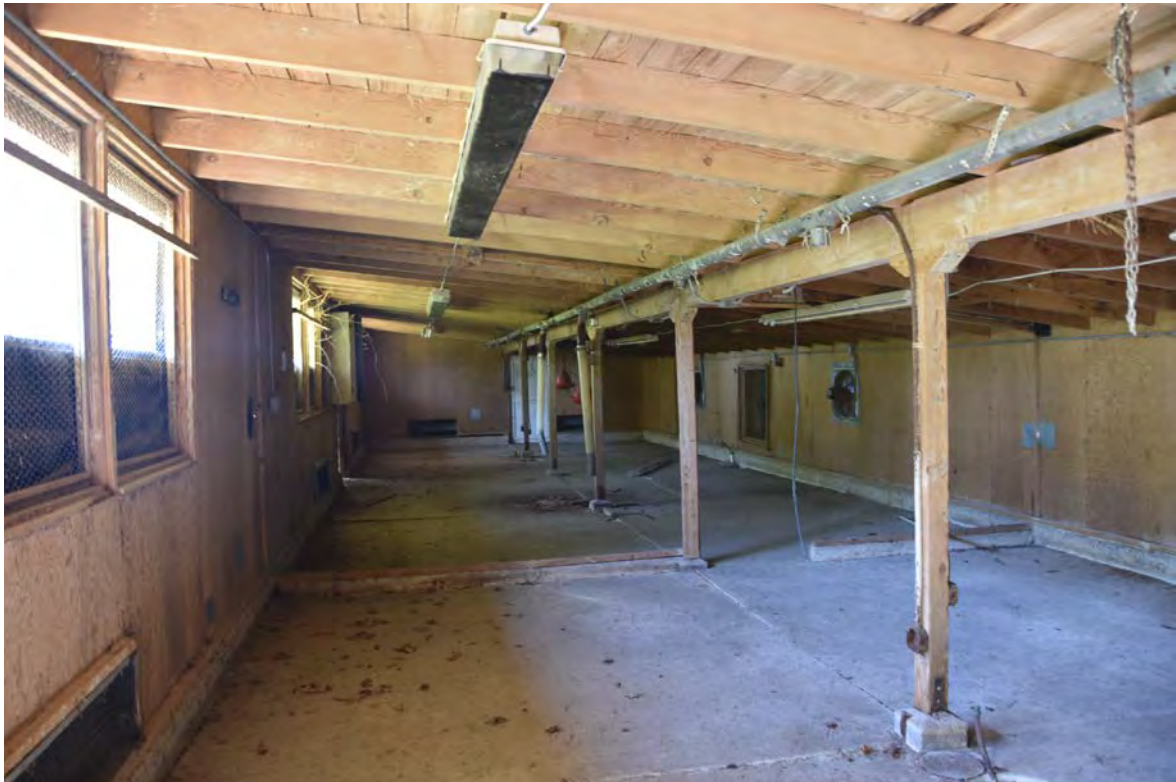
Photo 4 – Building 273, Experimental Laying House for Breeding, Central Farm, Overview of the Interior, Looking West
