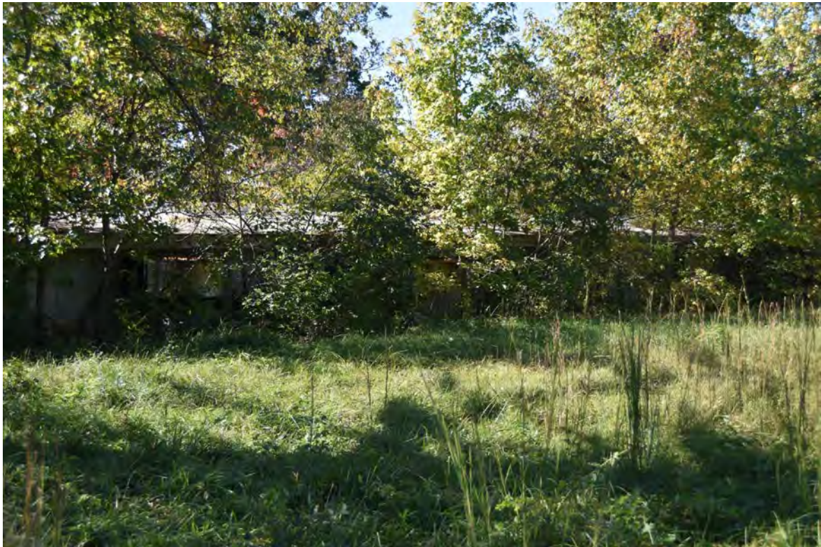
Photo 3 – Building 274, Experiment Laying House for Breeding, Central Farm, View of North Elevation, Looking Southwest
