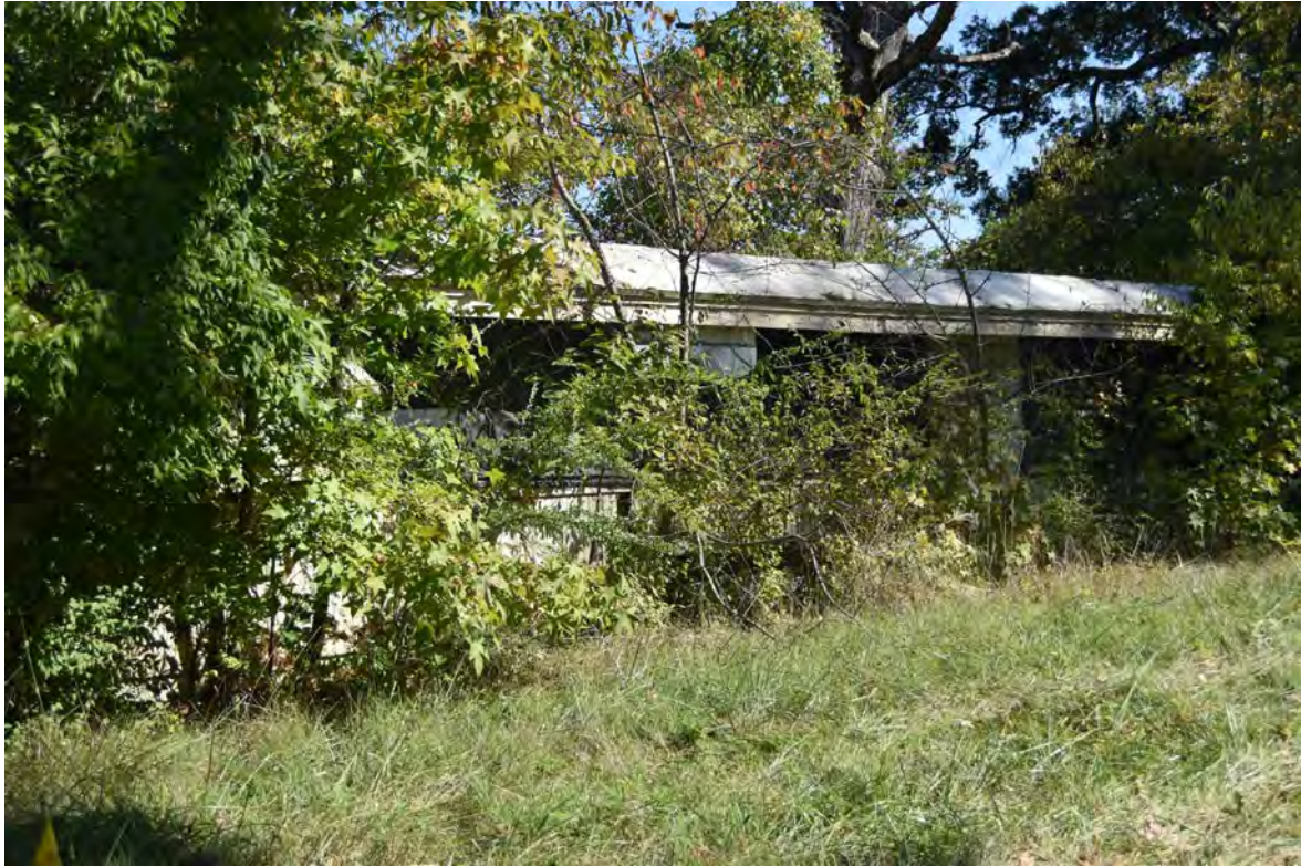
Photo 1 – Building 274, Experimental Laying House for Breeding, Central Farm, View of South Elevation, Looking Northeast
