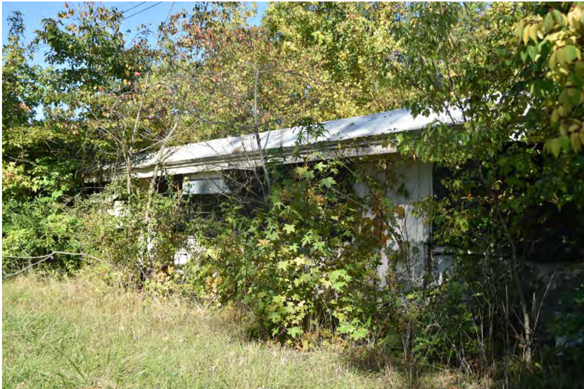
Photo 2 – Building 274, Experimental Laying House for Breeding, Central Farm, View of South Elevation, Looking Northwest
