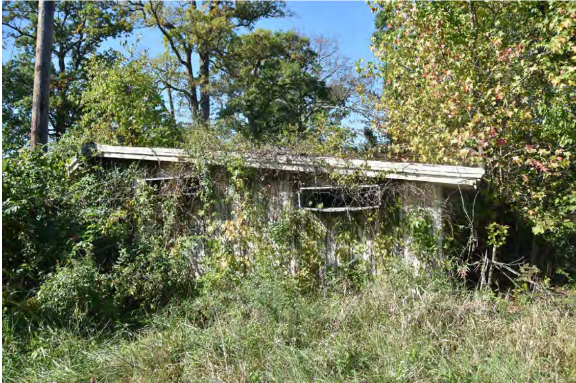
Photo 3 – Building 275, Experiment Laying House for Breeding, Central Farm, View of East Elevation, Looking West
