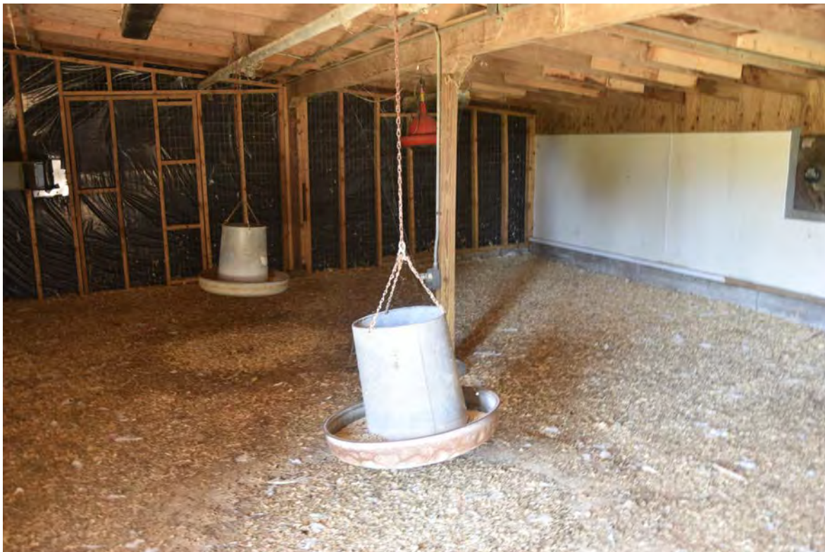
Photo 4 – Building 277, Experimental Laying House for Breeding, Central Farm, Overview of the Interior, Looking Northwest
