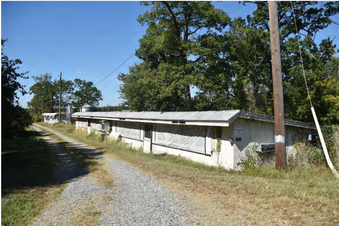
Photo 1 – Building 278, Experimental Laying House for Breeding, Central Farm, View of South and East Elevations, Looking Northwest
