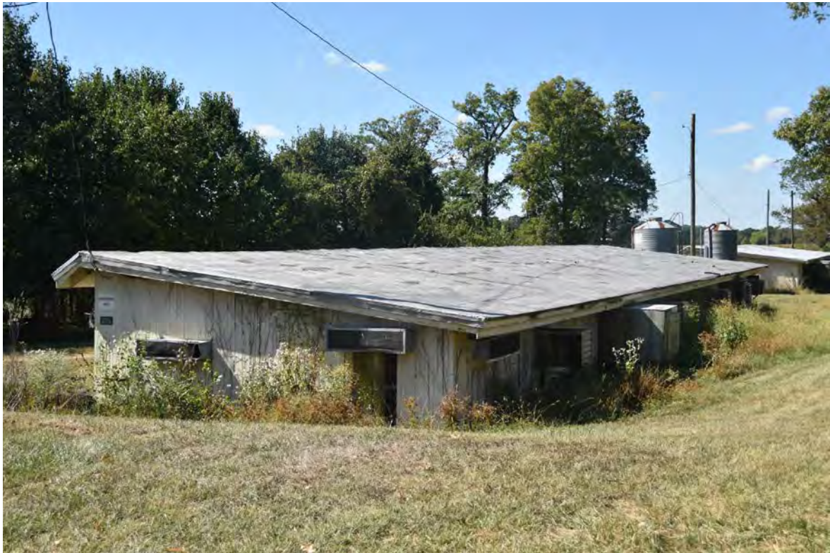
Photo 3 – Building 278, Experiment Laying House for Breeding, Central Farm, View of East and North Elevations, Looking Southwest
