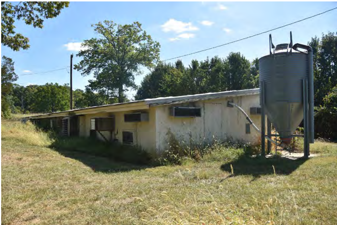
Photo 2 – Building 278, Experimental Laying House for Breeding, Central Farm, View of North and West Elevations, Looking Southeast
