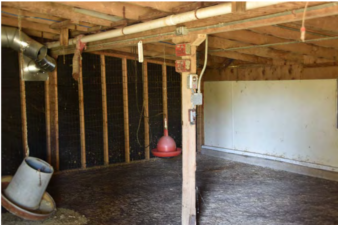
Photo 4 – Building 278, Experimental Laying House for Breeding, Central Farm, Overview of the Interior, Looking Northwest
