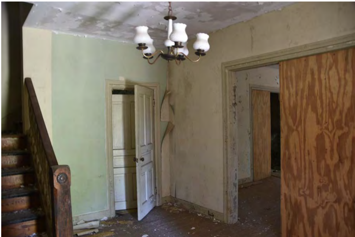
Photo 4 – Building 281, House for Poultryman, Central Farm, View of Hall, Looking Northeast
