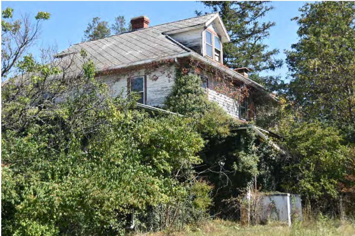
Photo 2 – Building 281, House for Poultryman, Central Farm, View of South and West Elevations, Looking Northeast
