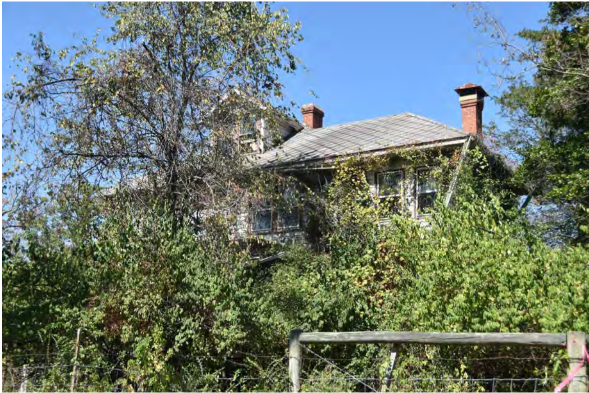
Photo 1 – Building 281, House for Poultryman, Central Farm, View of South Elevation, Looking Northwest
