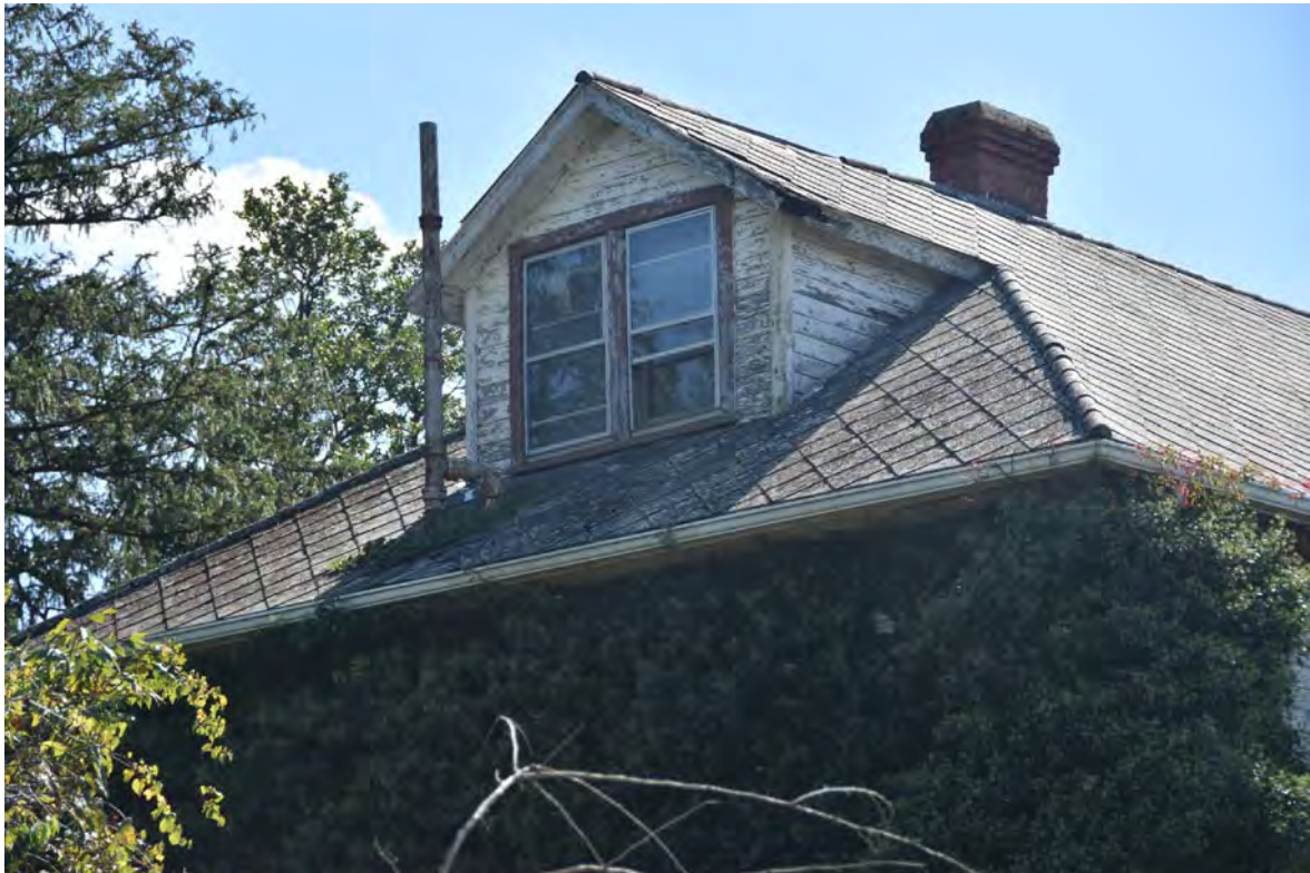
Photo 3 – Building 281, House for Poultryman, Central Farm, View of North Elevation Dormer, Looking Southeast
