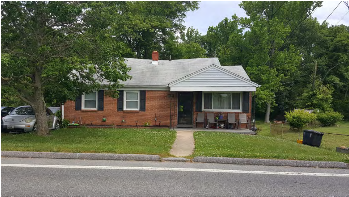
Photo 1 - Primary (south) elevation, 5438 Odell Road, Looking North
