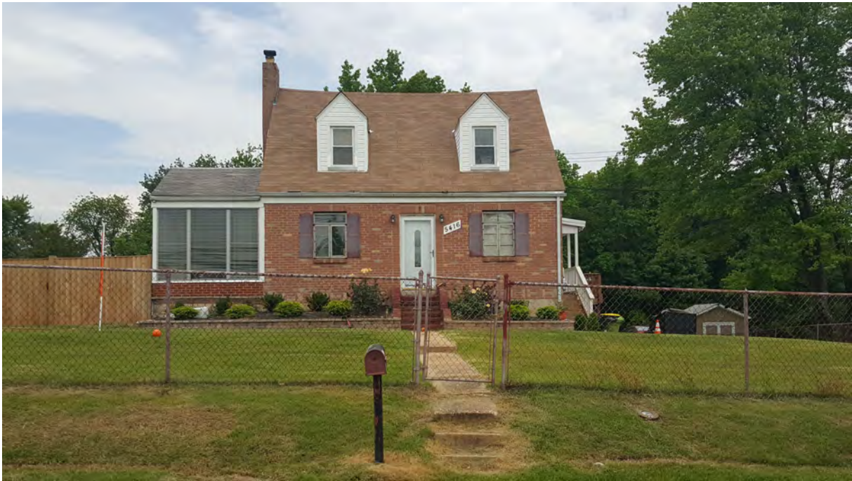
Photo 1 - Primary (south) elevation, 5416 Odell Road, Looking North
