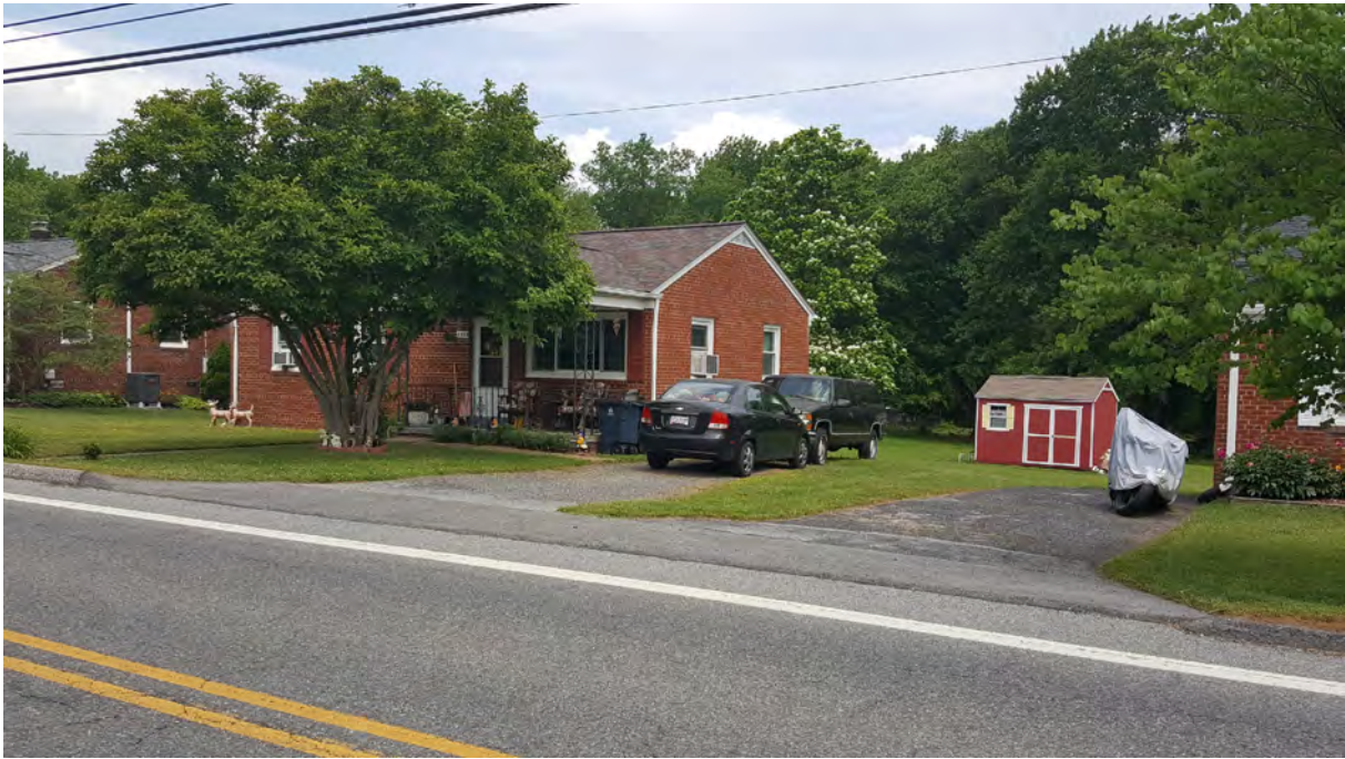
Photo 3 - Oblique view of primary elevation, 5428 Odell Road, Looking Northwest
