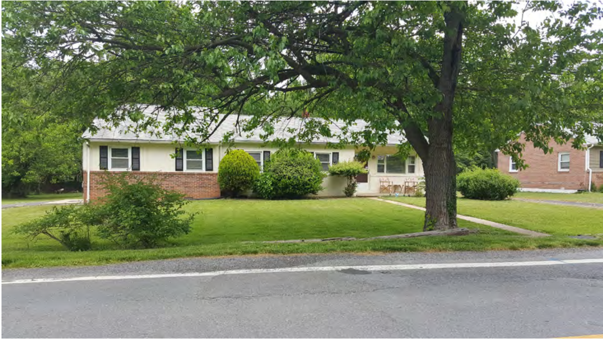
Photo 1 - Primary (south) elevation, 5600 Odell Road, Looking North
