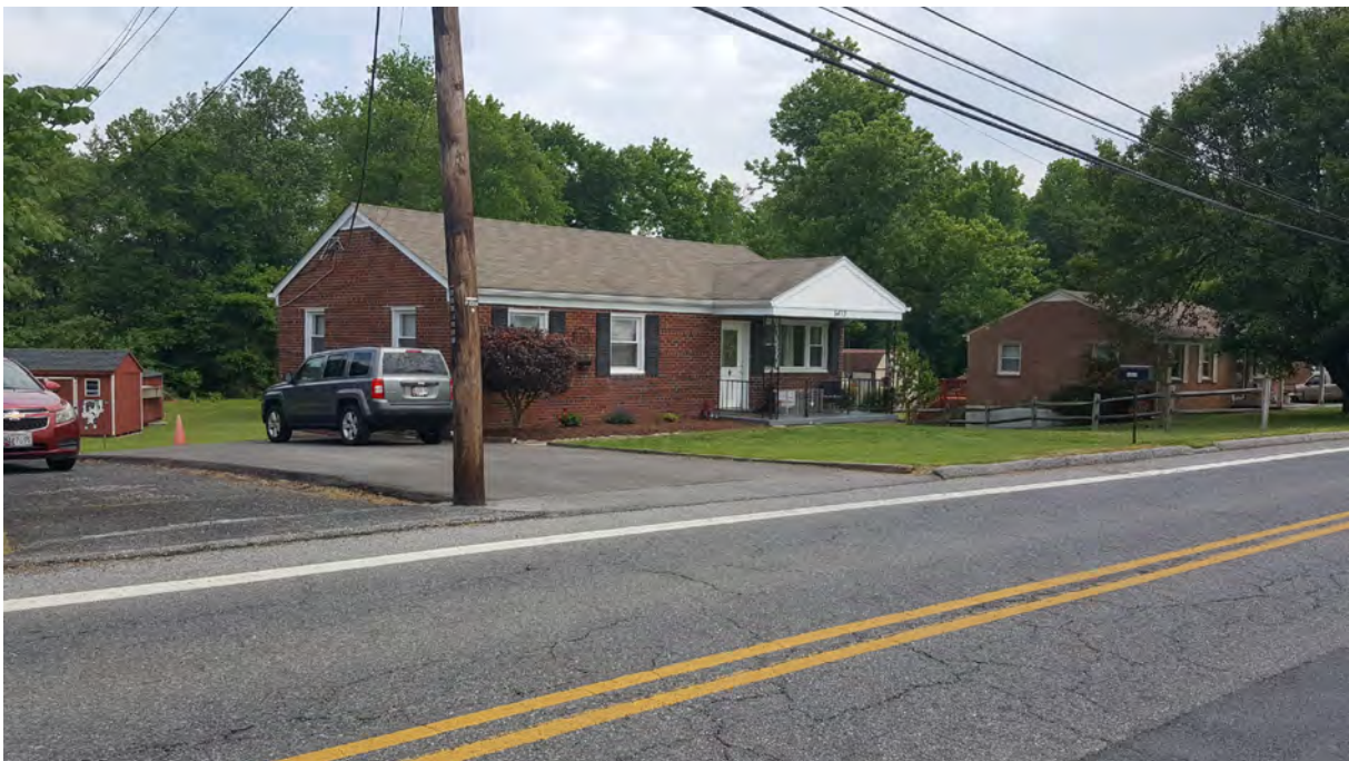
Photo 2 - Oblique view of primary elevation, 5432 Odell Road, Looking Northeast
