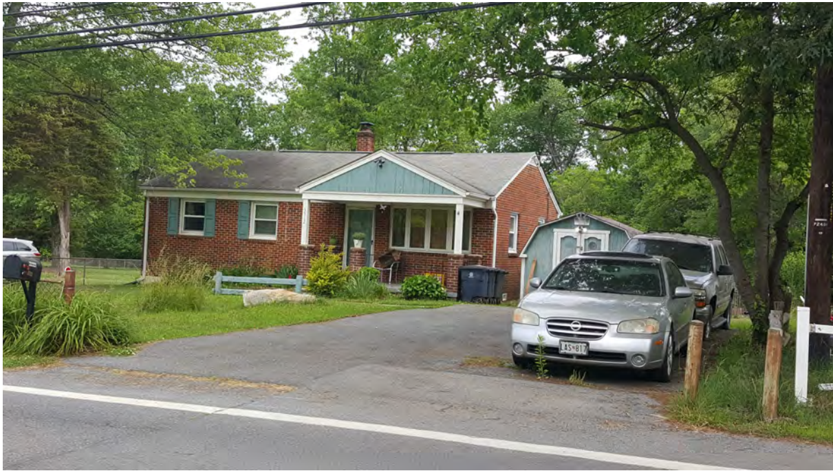
Photo 3 - Oblique view of primary elevation, 5512 Odell Road, Looking Northwest
