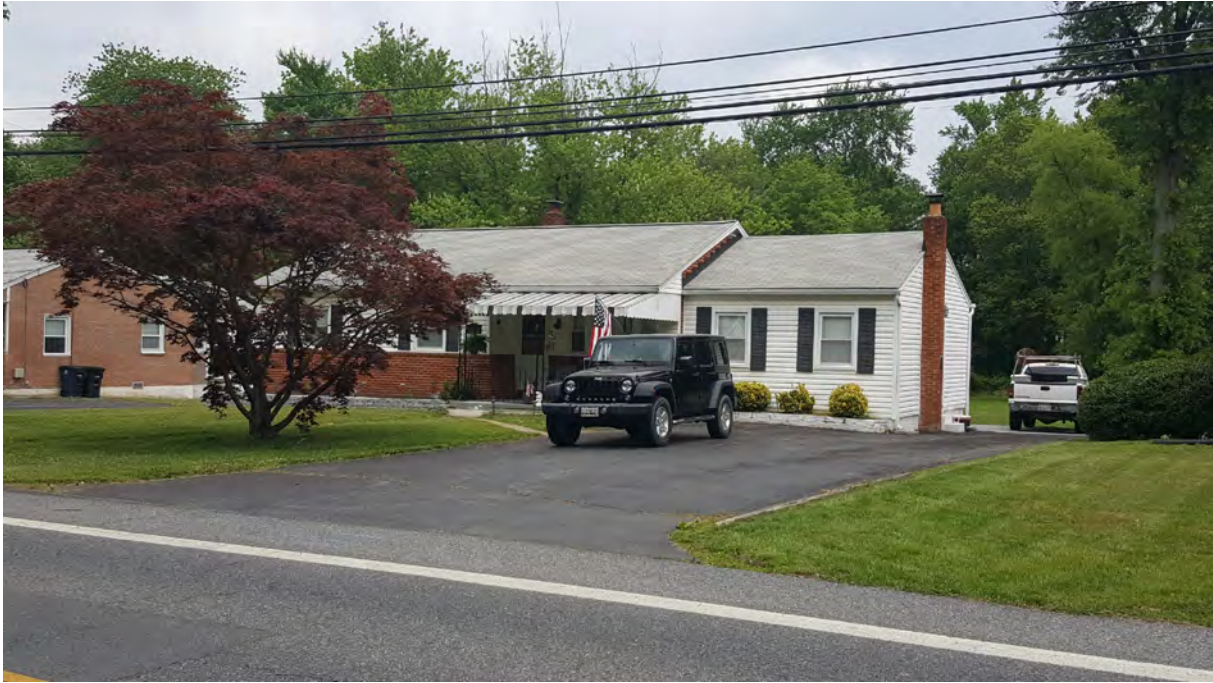
Photo 3 - Oblique view of primary elevation, 5604 Odell Road, Looking Northwest
