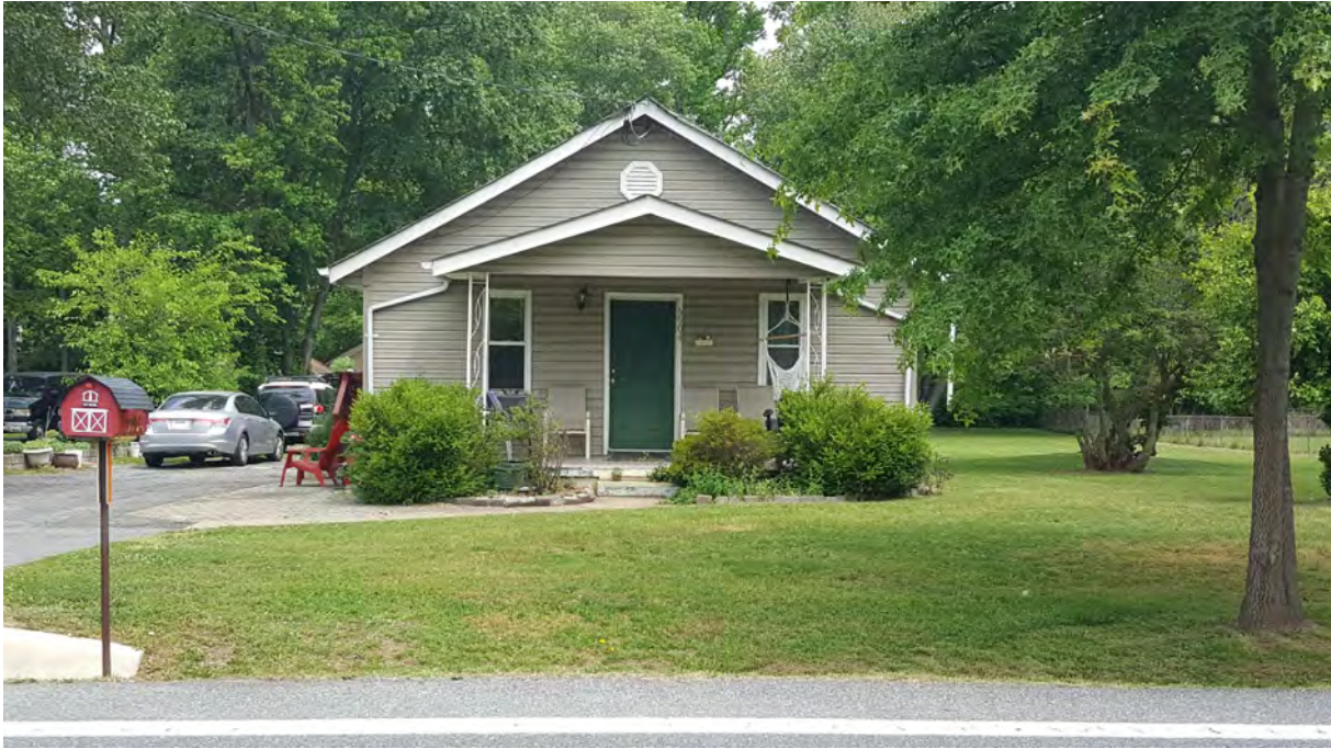
Photo 1 - Primary (south) elevation, 5504 Odell Road, Looking North
