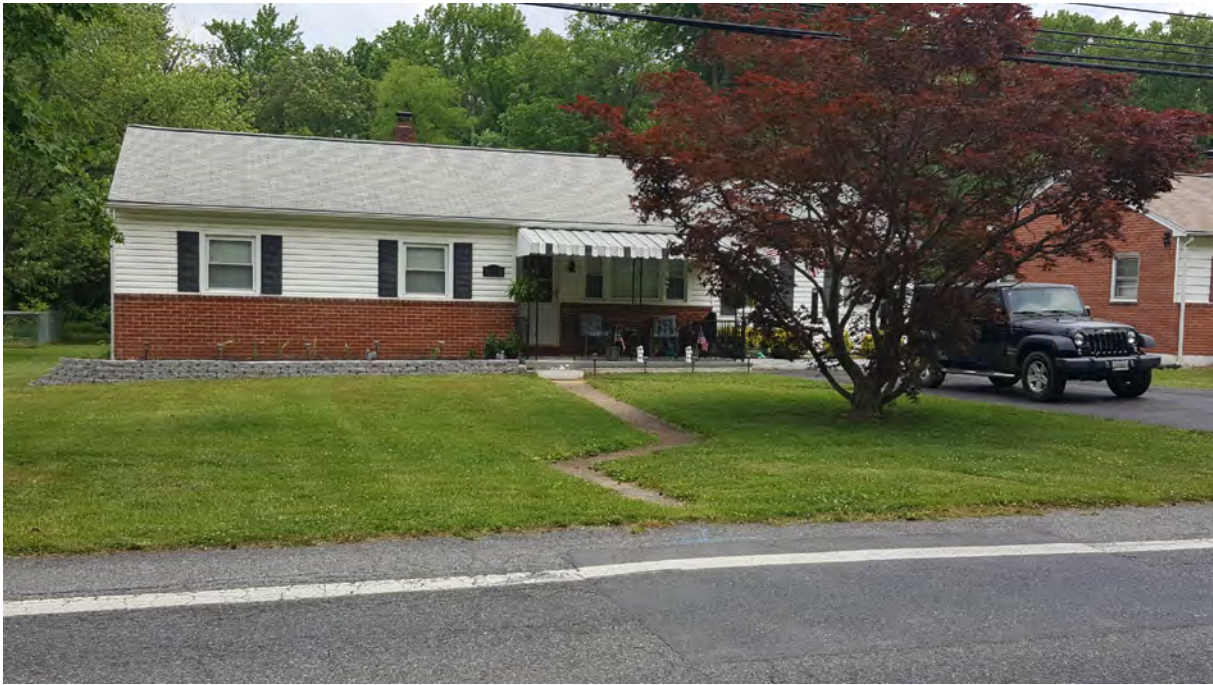
Photo 1 - Primary (south) elevation, 5604 Odell Road, Looking North
