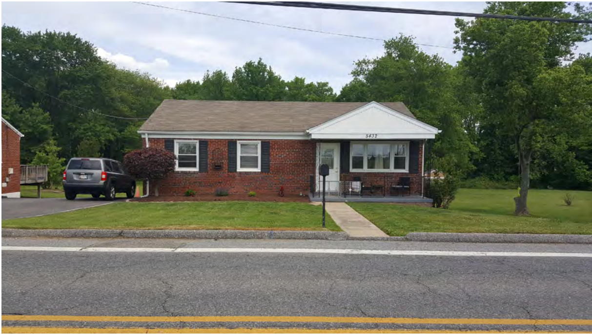
Photo 1 - Primary (south) elevation, 5432 Odell Road, Looking North
