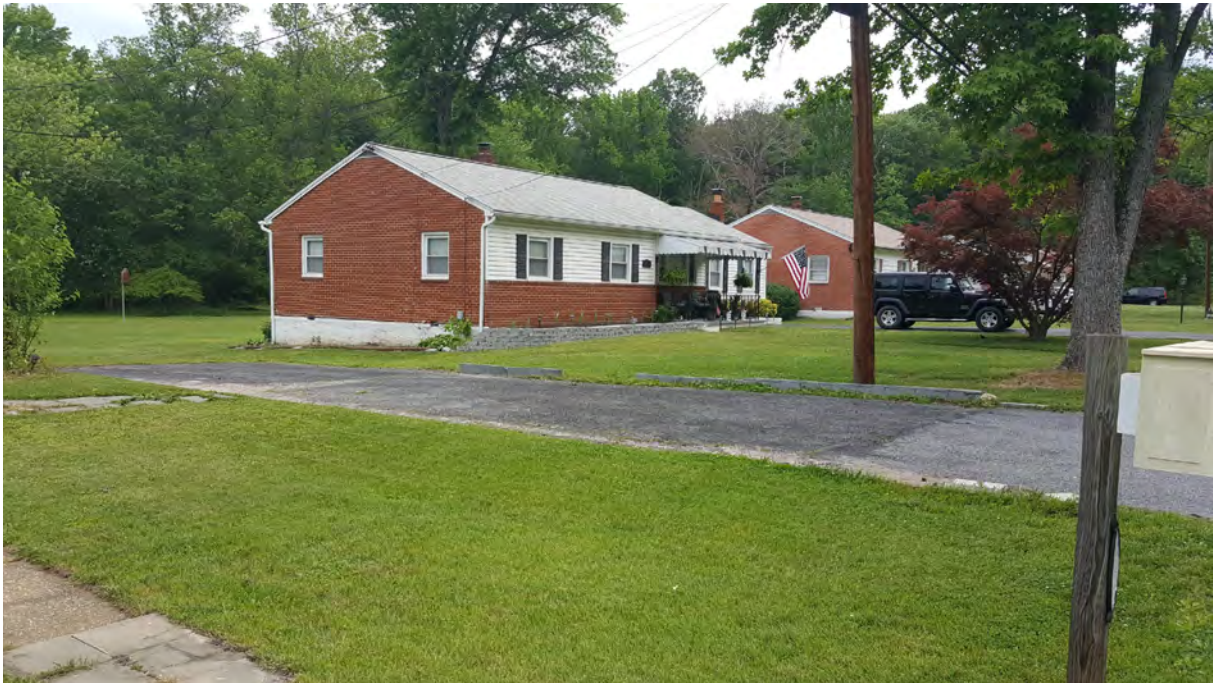
Photo 2 - Oblique view of primary elevation, 5604 Odell Road, Looking Northeast
