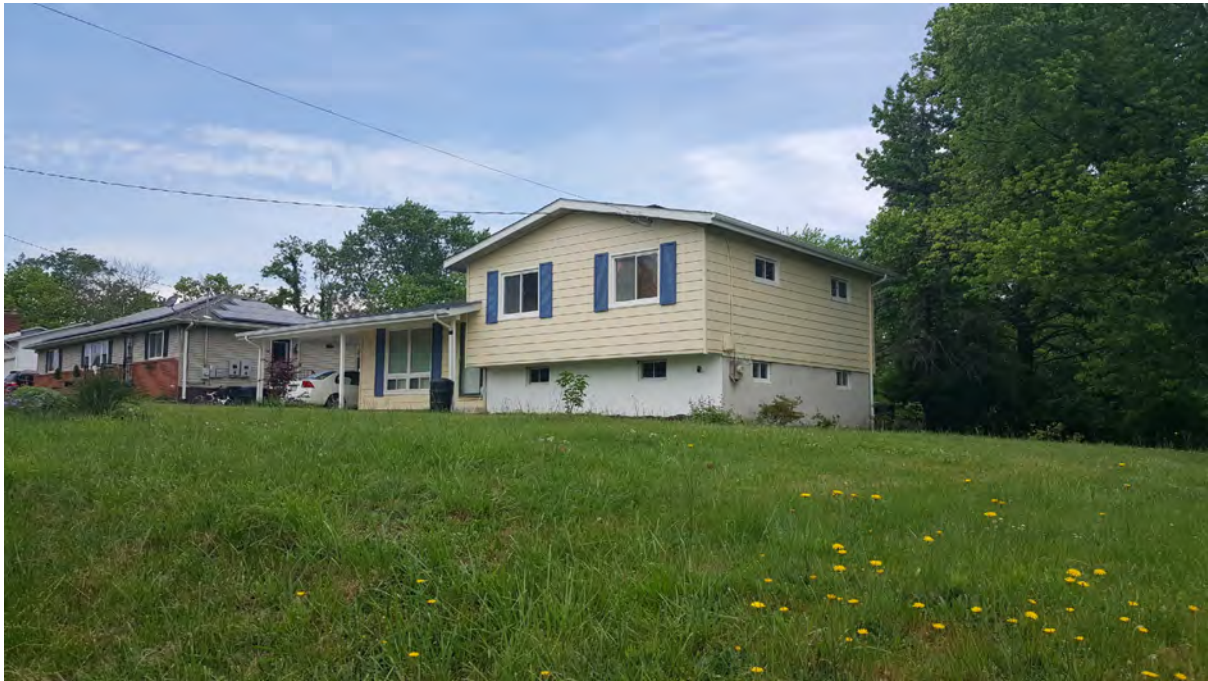
Photo 3 - Oblique view of primary elevation, 5412 Odell Road, Looking Northwest
