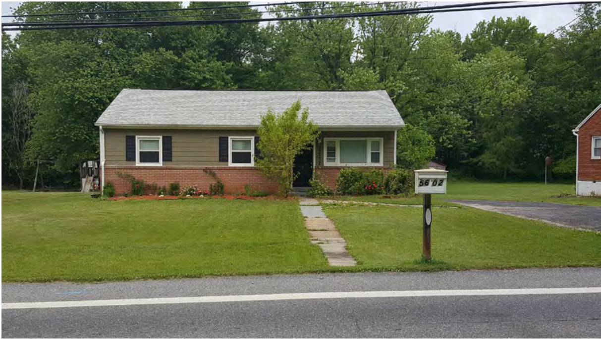
Photo 1 - Primary (south) elevation, 5602 Odell Road, Looking North
