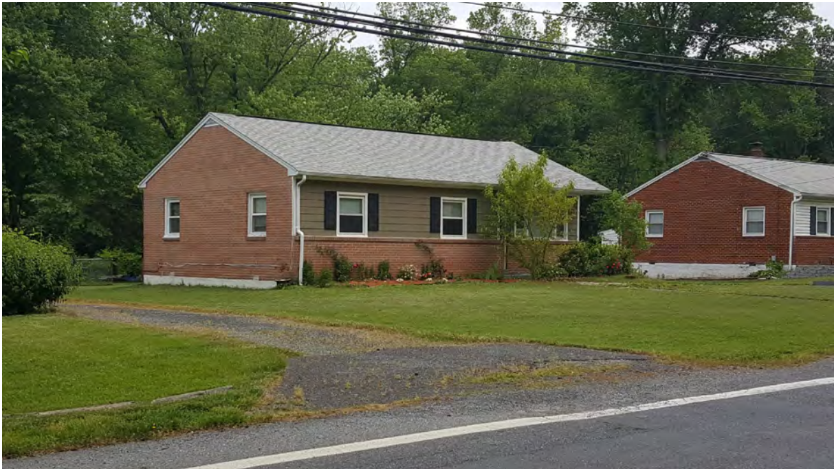
Photo 2 - Oblique view of primary elevation, 5602 Odell Road, Looking Northeast
