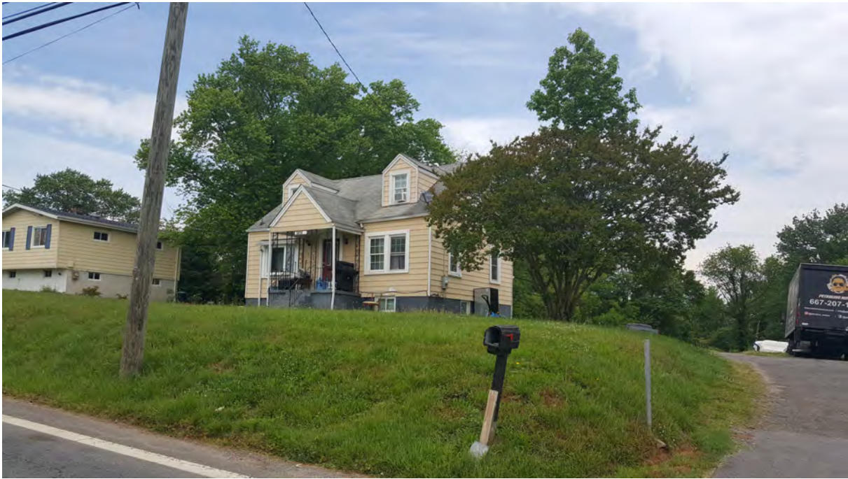
Photo 3 - Oblique view of primary elevation, 5414 Odell Road, Looking Northwest
