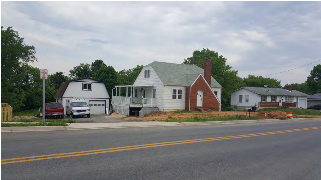
Photo 2 - Oblique view of primary elevation, 5406 Odell Road, Looking Northeast
