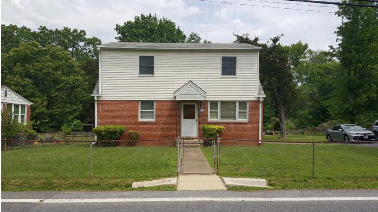
Photo 1 - Primary (south) elevation, 5510 Odell Road, Looking North
