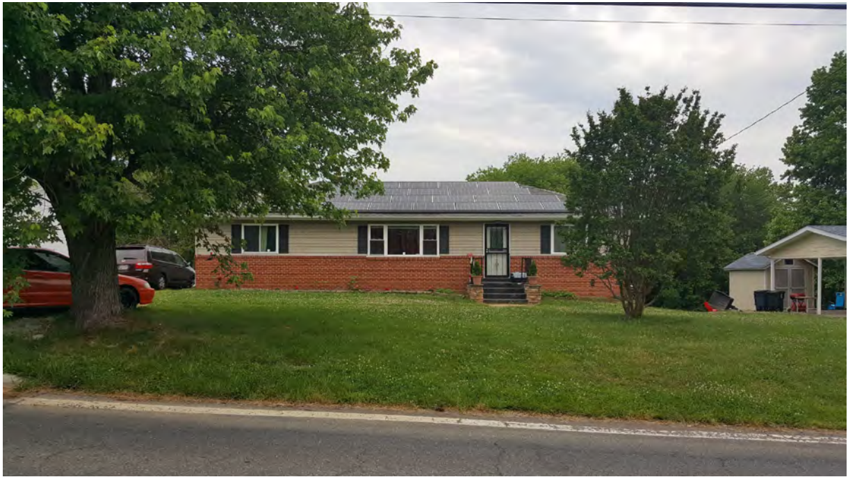
Photo 1 - Primary (south) elevation, 5410 Odell Road, Looking North
