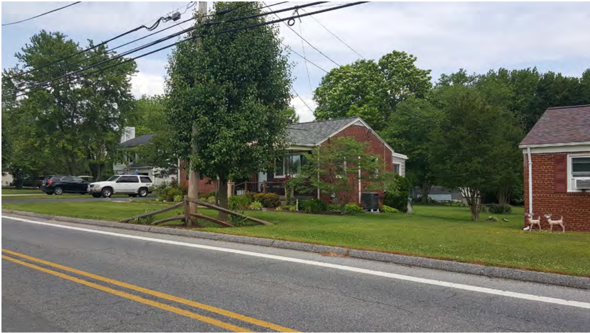
Photo 3 - Oblique view of primary elevation, 5426 Odell Road, Looking Northwest
