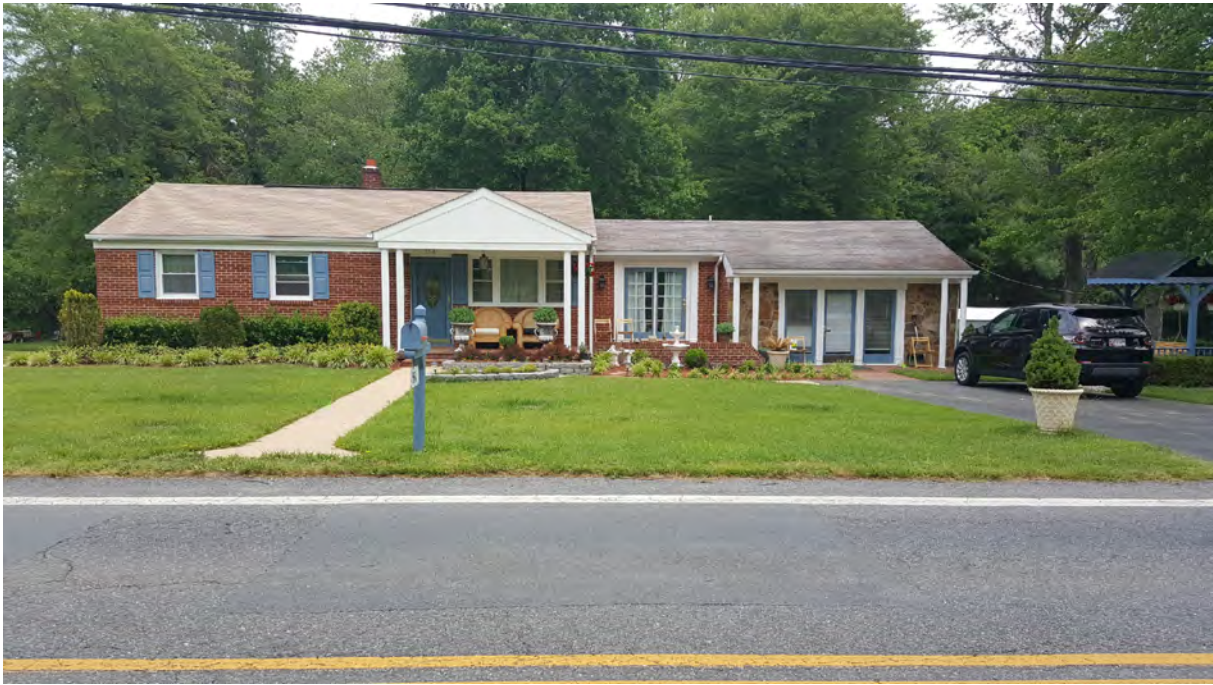
Photo 1 - Primary (south) elevation, 5518 Odell Road, Looking North
