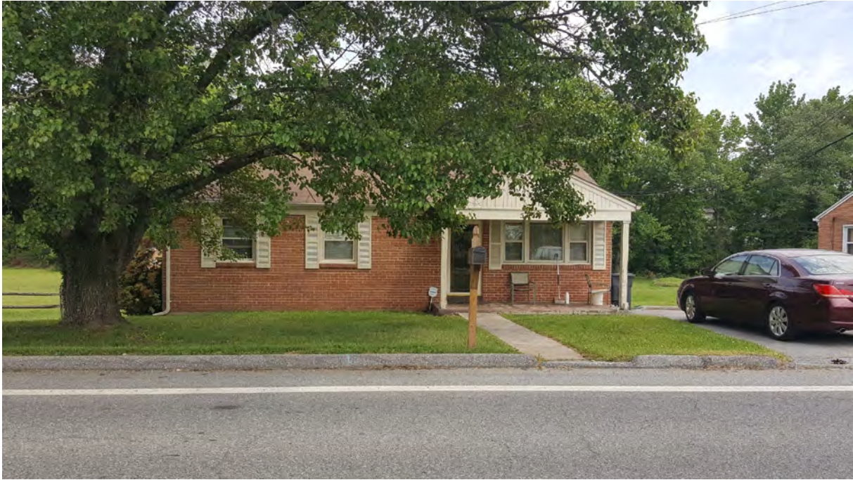
Photo 1 - Primary (south) elevation, 5434 Odell Road, Looking North
