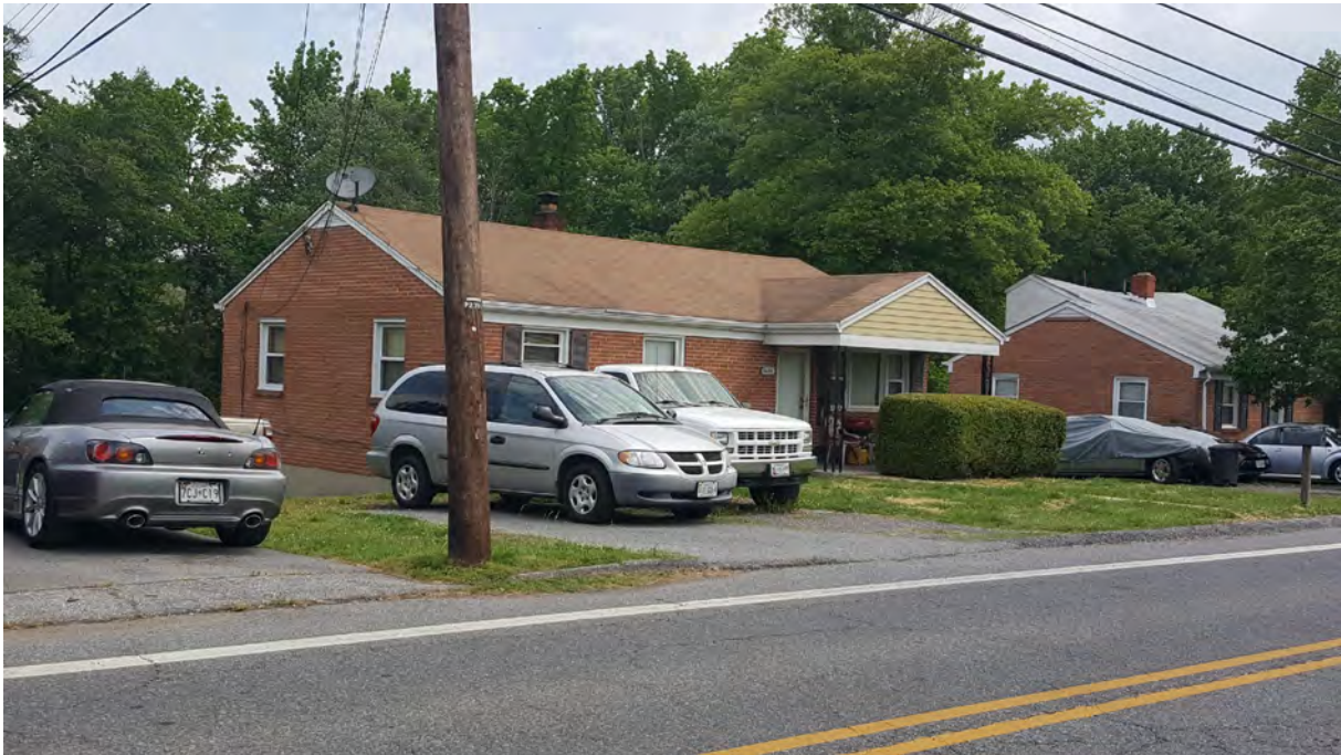
Photo 2 - Oblique view of primary elevation, 5436 Odell Road, Looking Northeast
