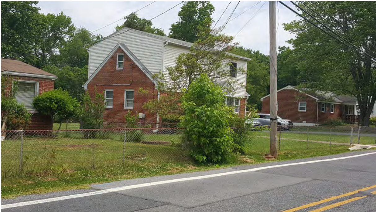
Photo 2 - Oblique view of primary elevation, 5510 Odell Road, Looking Northeast
