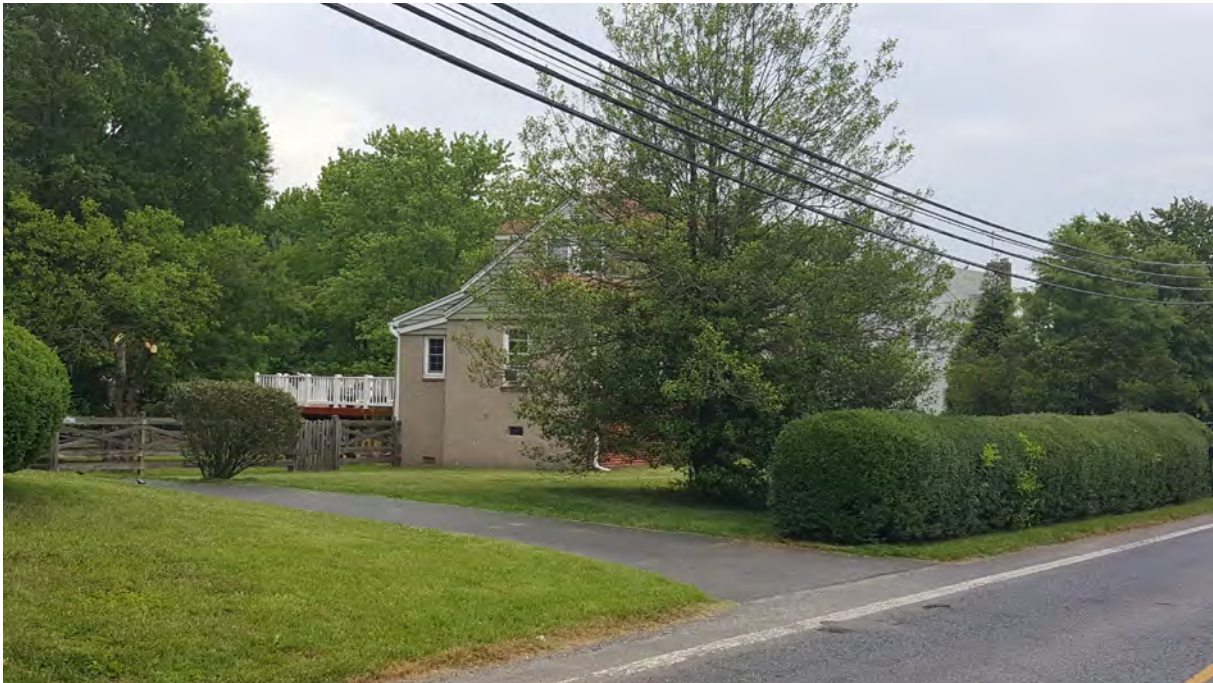
Photo 2 - Oblique view of primary elevation, 5420 Odell Road, Looking Northeast
