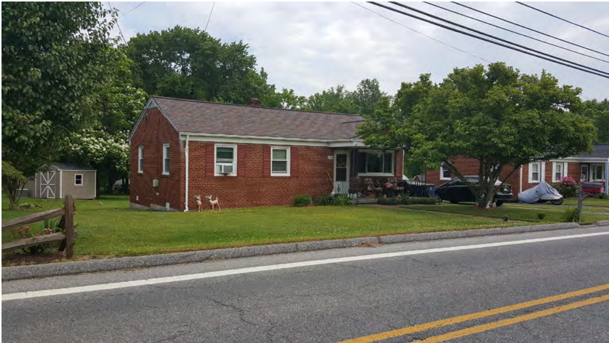
Photo 2 - Oblique view of primary elevation, 5428 Odell Road, Looking Northeast
