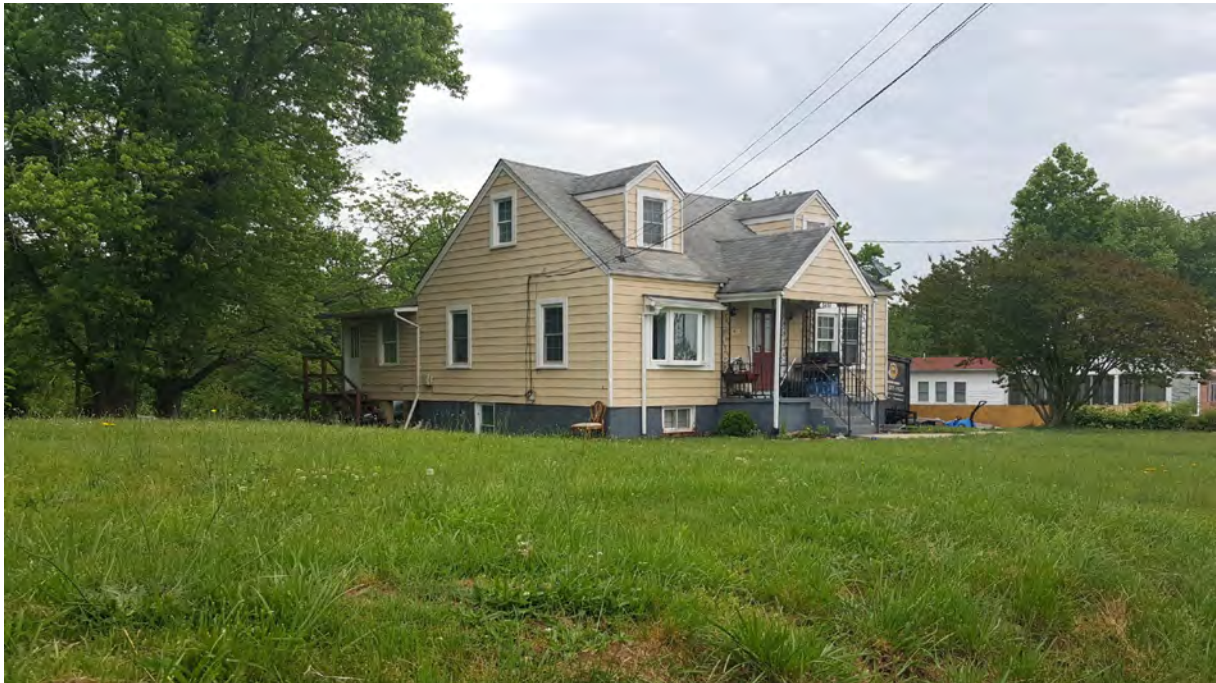
Photo 2 - Oblique view of primary elevation, 5414 Odell Road, Looking Northeast
