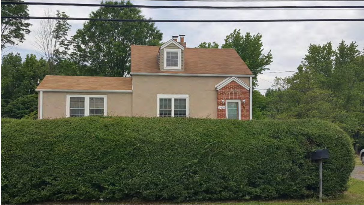
Photo 1 - Primary (south) elevation, 5420 Odell Road, Looking North
