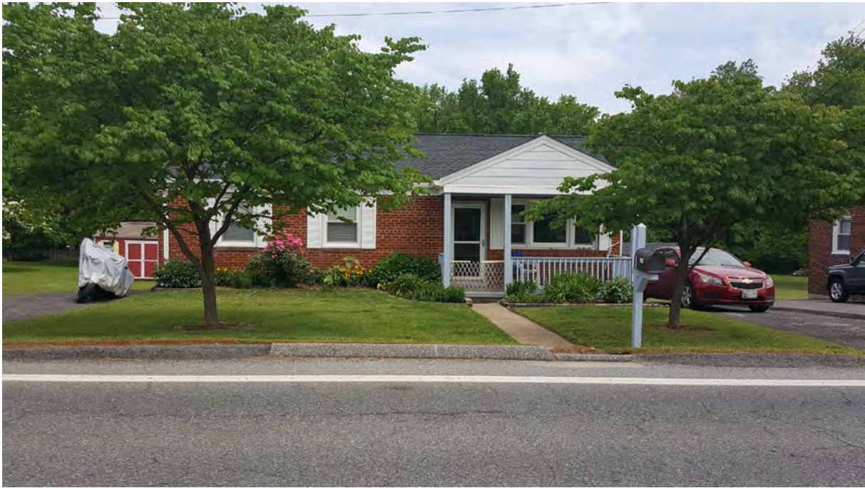
Photo 1 - Primary (south) elevation, 5430 Odell Road, Looking North
