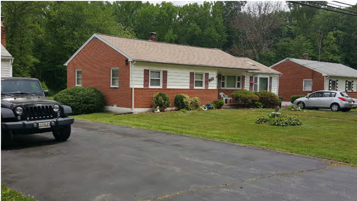
Photo 2 - Oblique view of primary elevation, 5606 Odell Road, Looking Northeast
