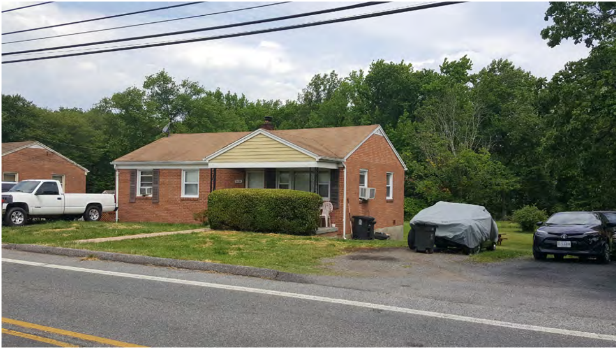
Photo 3 - Oblique view of primary elevation, 5436 Odell Road, Looking Northwest
