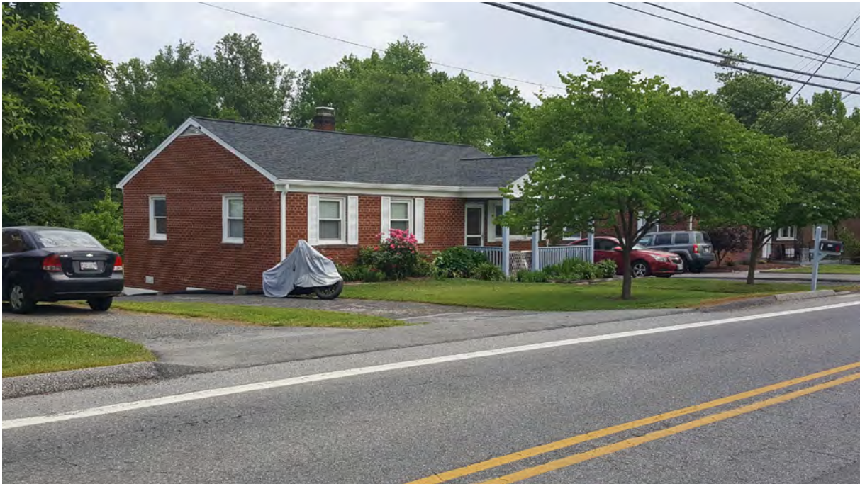
Photo 2 - Oblique view of primary elevation, 5430 Odell Road, Looking Northeast
