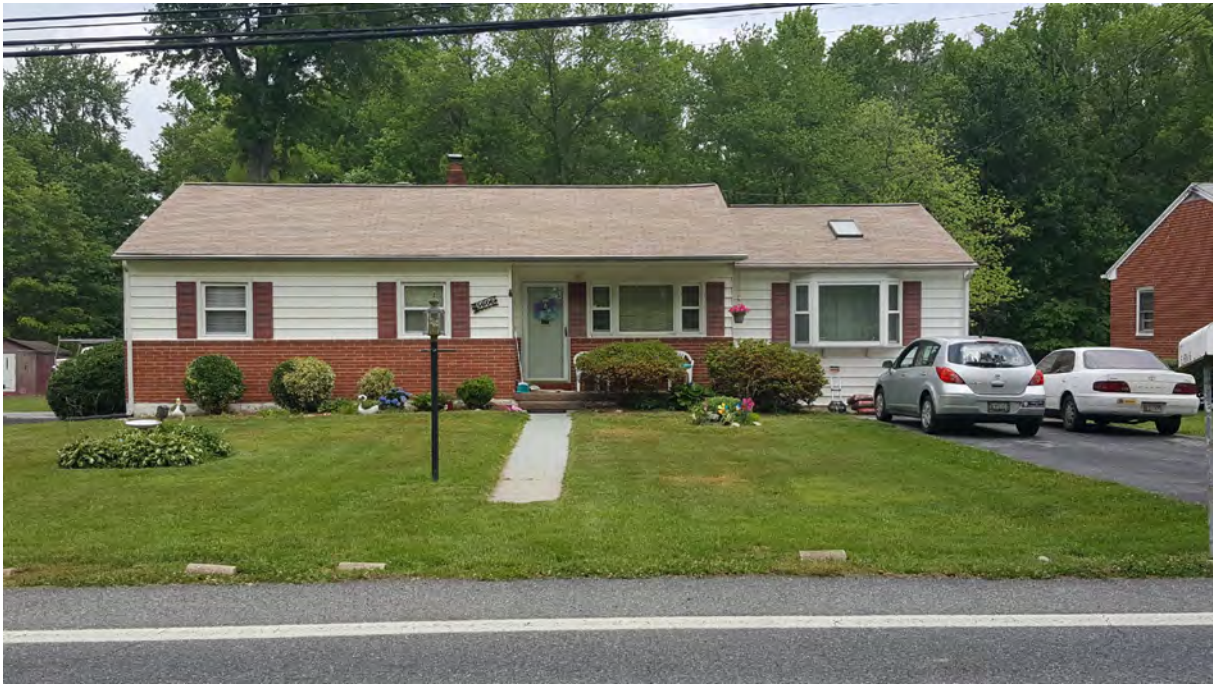
Photo 1 - Primary (south) elevation, 5606 Odell Road, Looking North
