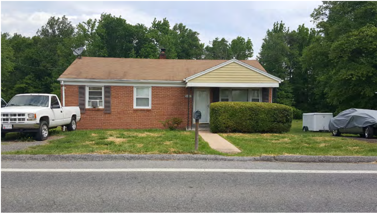
Photo 1 - Primary (south) elevation, 5436 Odell Road, Looking North
