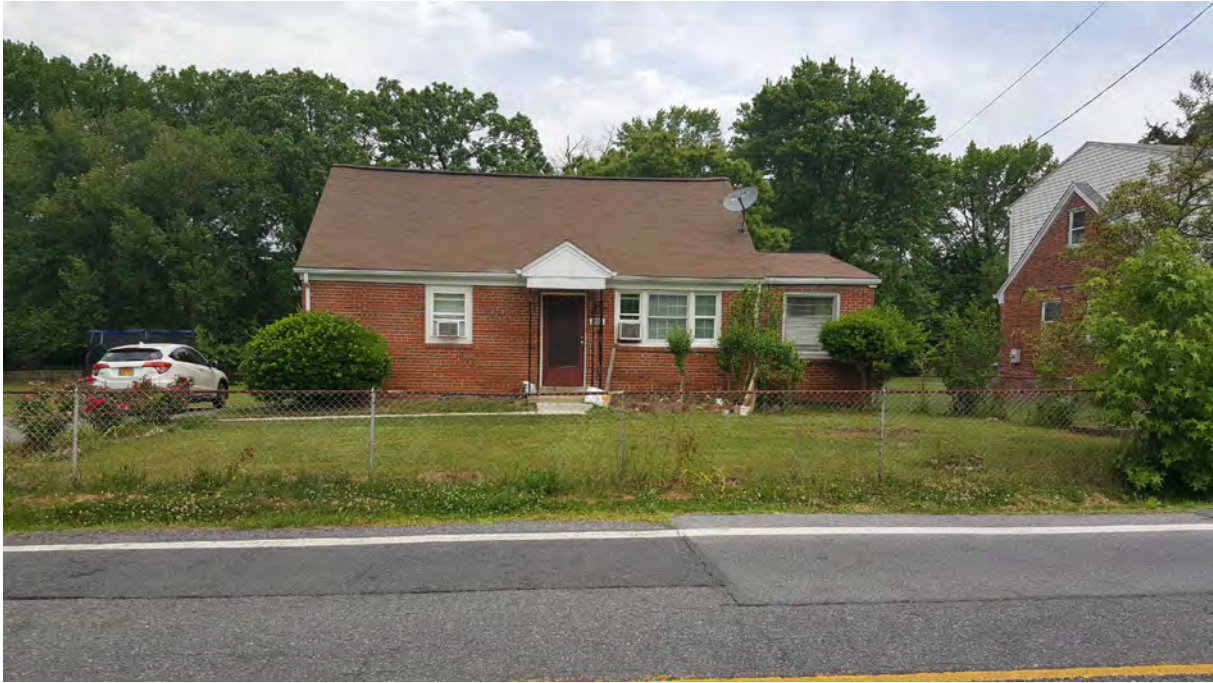
Photo 1 - Primary (south) elevation, 5508 Odell Road, Looking North
