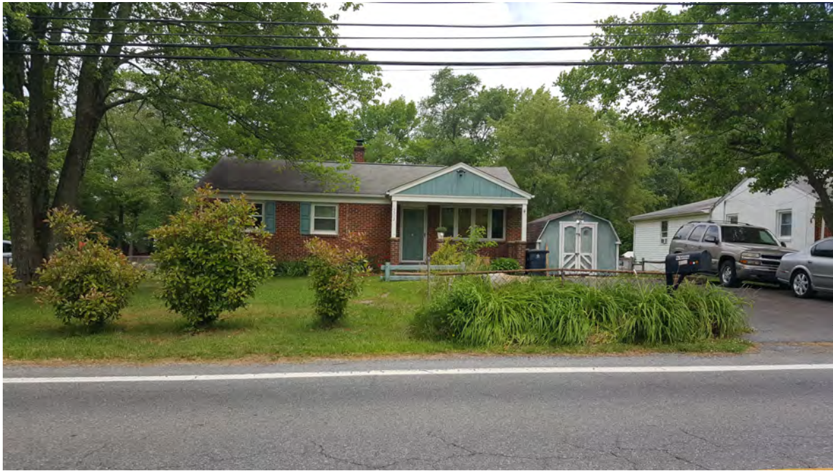
Photo 1 - Primary (south) elevation, 5512 Odell Road, Looking North
