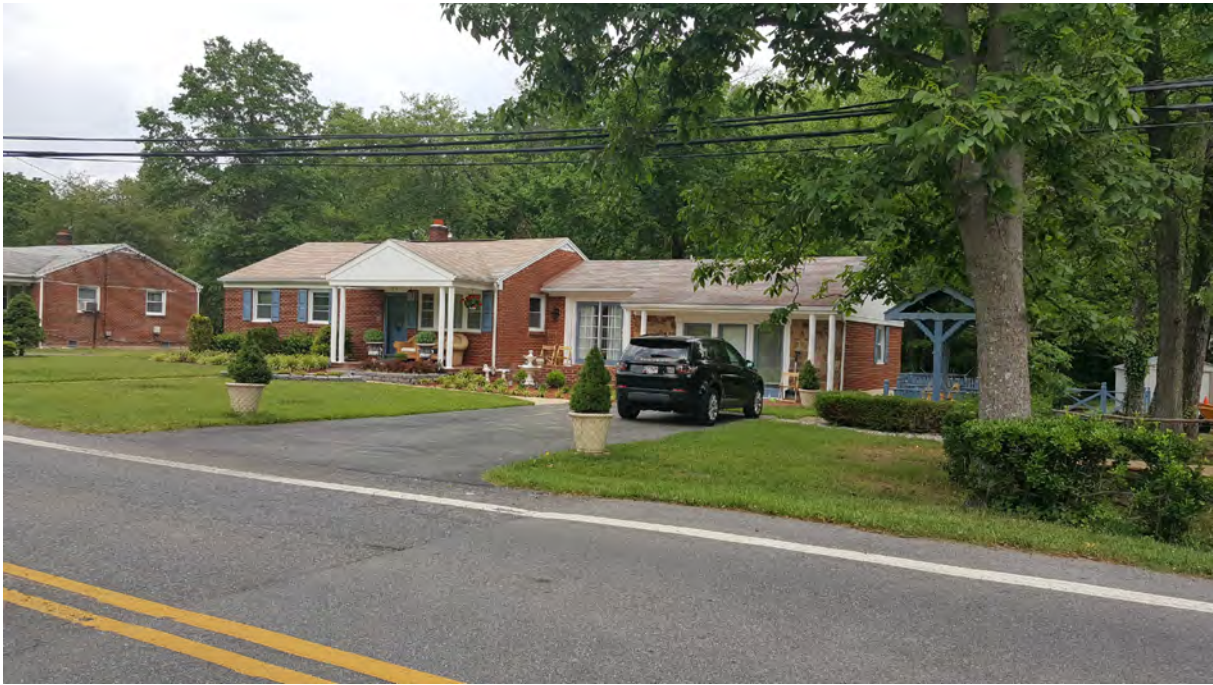
Photo 3 - Oblique view of primary elevation, 5518 Odell Road, Looking Northwest
