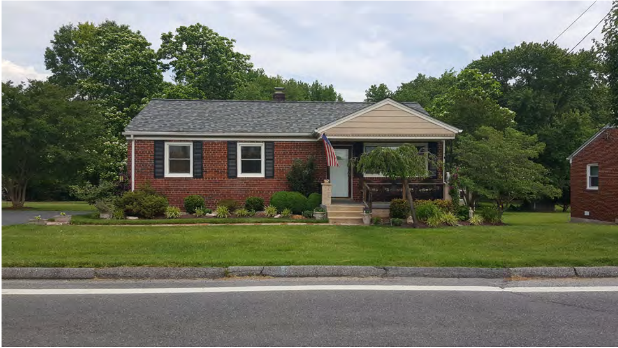
Photo 1 - Primary (south) elevation, 5426 Odell Road, Looking North
