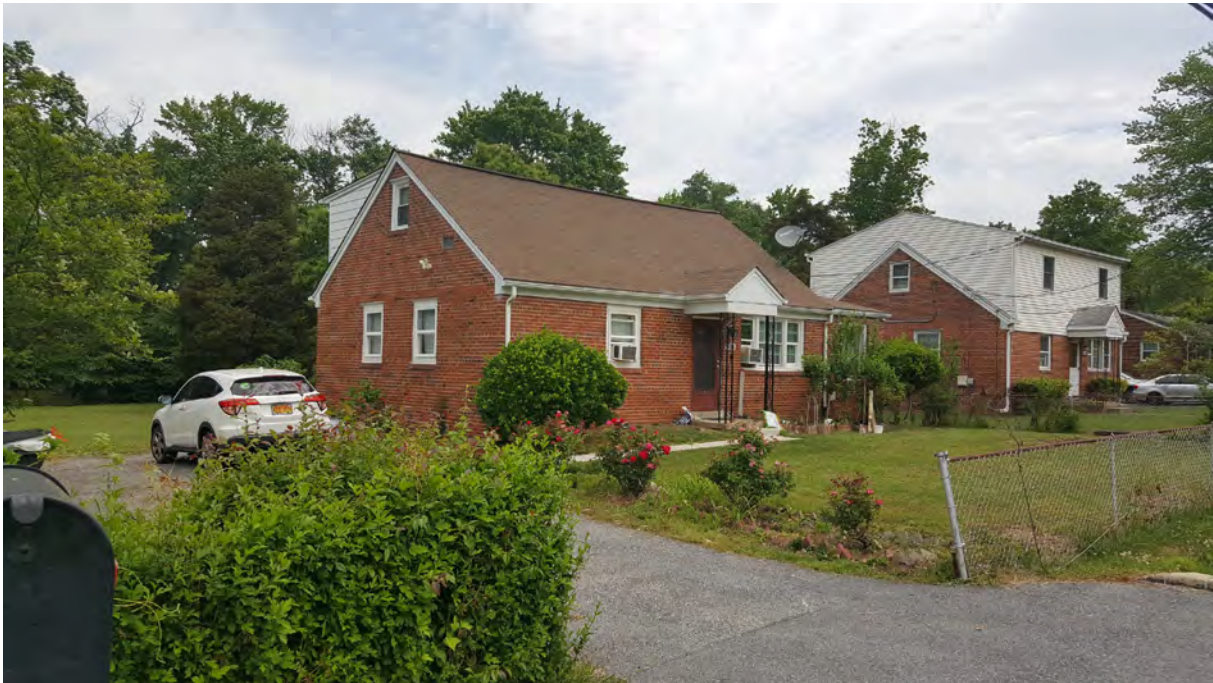
Photo 2 - Oblique view of primary elevation, 5508 Odell Road, Looking Northeast
