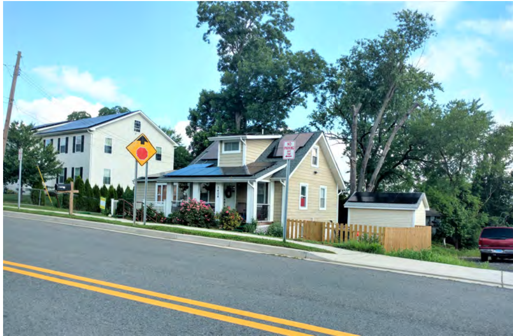
Photo 3 - Oblique view of primary elevation, 5404 Odell Road, Looking Northwest
