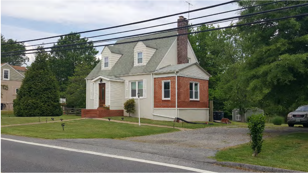
Photo 3 - Oblique view of primary elevation, 5422 Odell Road, Looking Northwest
