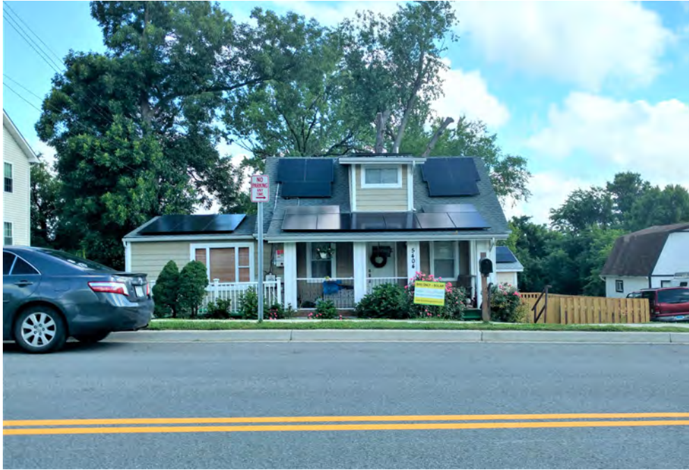
Photo 1 - Primary (south) elevation, 5404 Odell Road, Looking North
