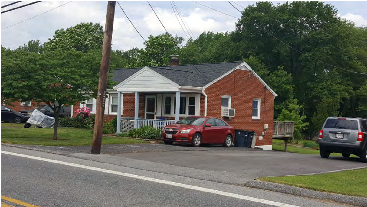
Photo 3 - Oblique view of primary elevation, 5430 Odell Road, Looking Northwest
