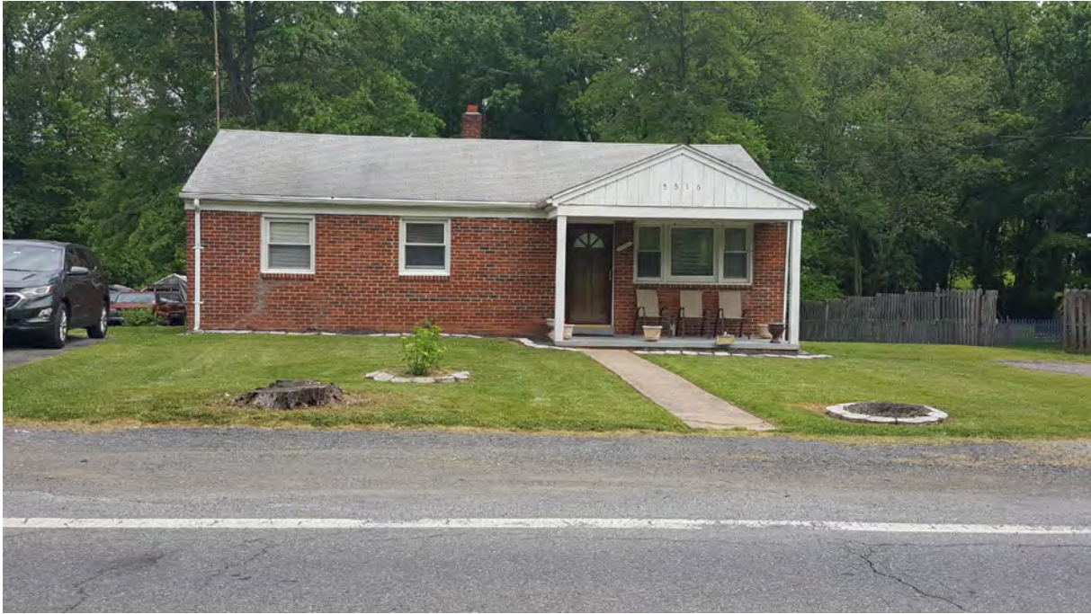
Photo 1 - Primary (south) elevation, 5516 Odell Road, Looking North
