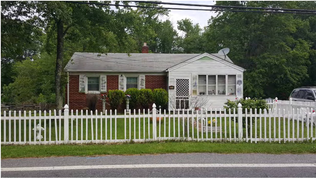
Photo 1 - Primary (south) elevation, 5514 Odell Road, Looking North
