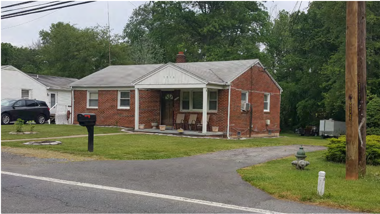
Photo 3 - Oblique view of primary elevation, 5516 Odell Road, Looking Northwest
