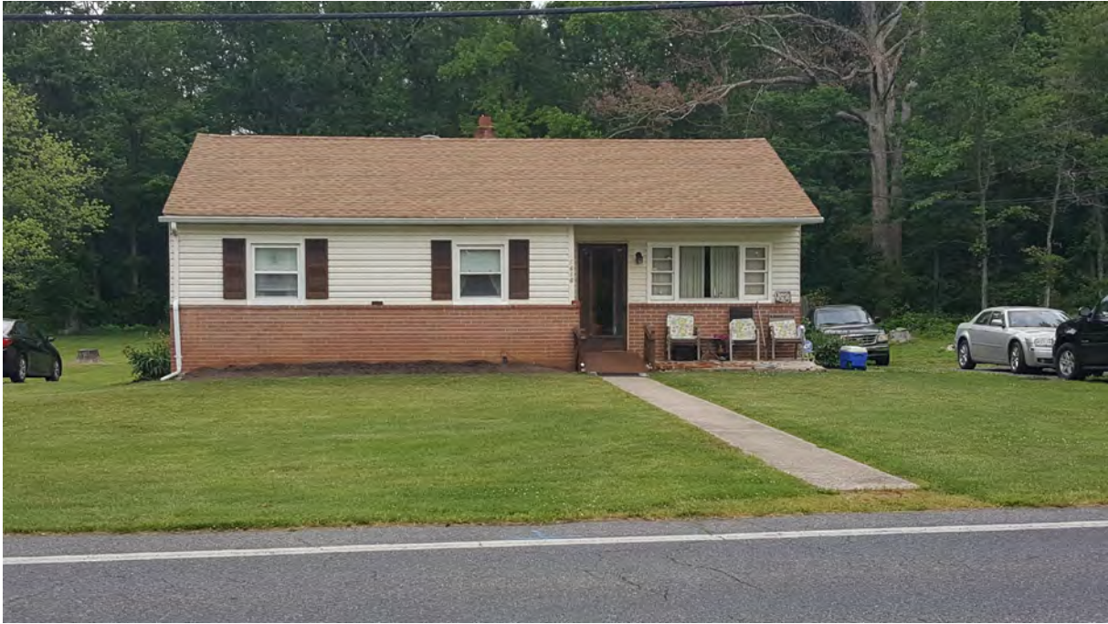
Photo 1 - Primary (south) elevation, 5610 Odell Road, Looking North
