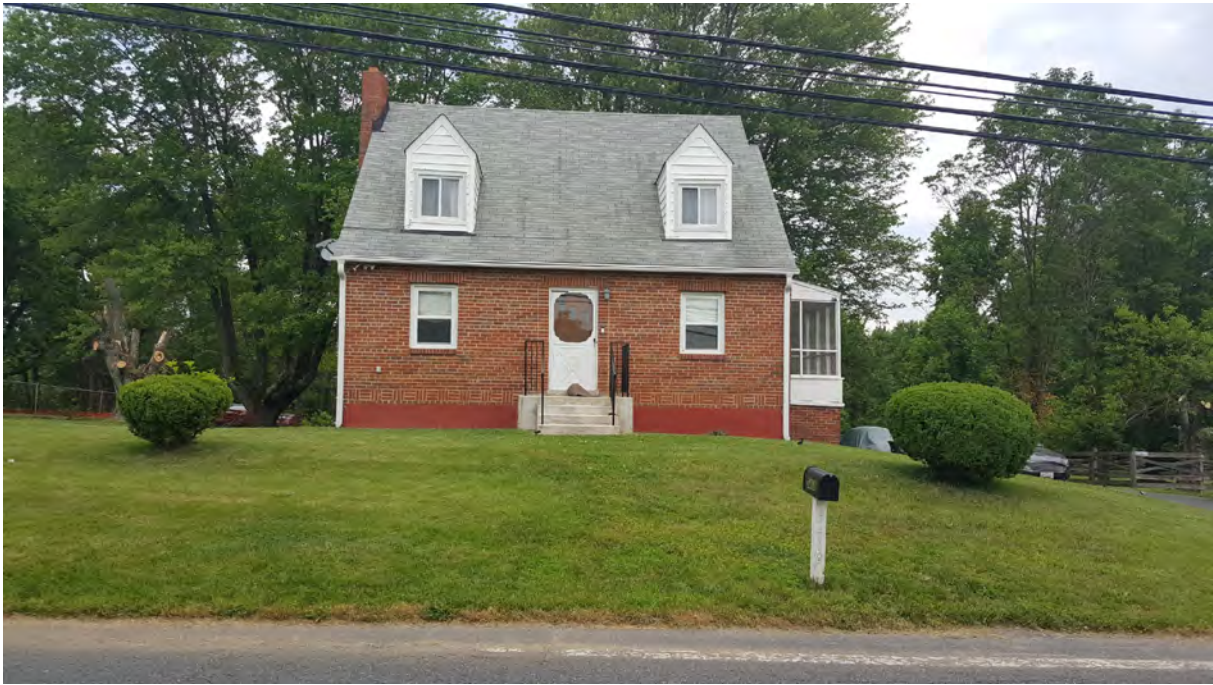
Photo 1 - Primary (south) elevation, 5418 Odell Road, Looking North
