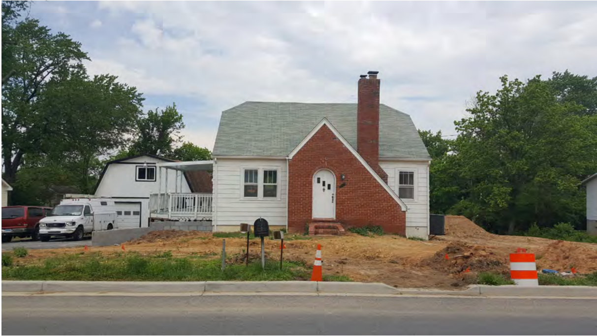
Photo 1 - Primary (south) elevation, 5406 Odell Road, Looking North
