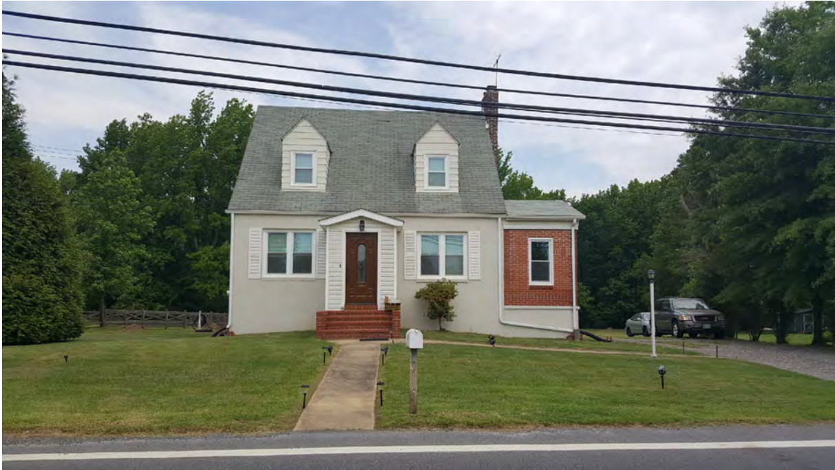
Photo 1 - Primary (south) elevation, 5422 Odell Road, Looking North
