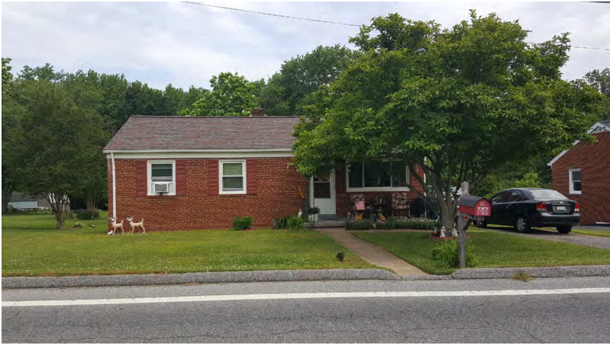
Photo 1 - Primary (south) elevation, 5428 Odell Road, Looking North
