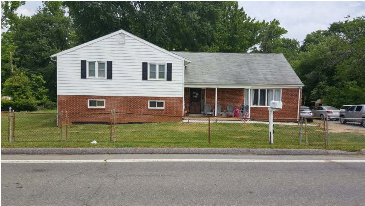
Photo 1 - Primary (south) elevation, 5440 Odell Road, Looking North
