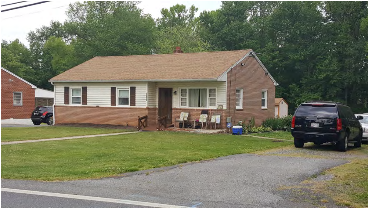
Photo 3 - Oblique view of primary elevation, 5610 Odell Road, Looking Northwest
