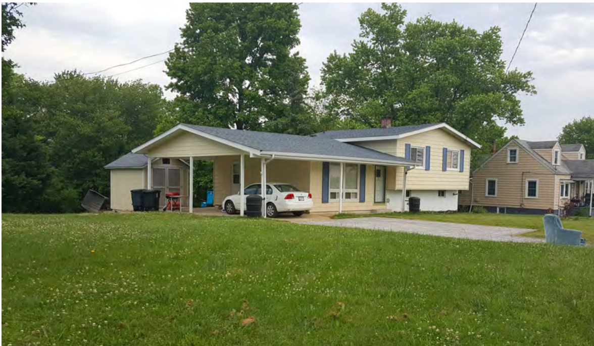
Photo 2 - Oblique view of primary elevation, 5412 Odell Road, Looking Northeast
