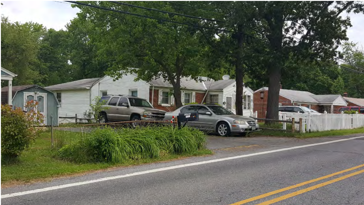
Photo 2 - Oblique view of primary elevation, 5514 Odell Road, Looking Northeast
