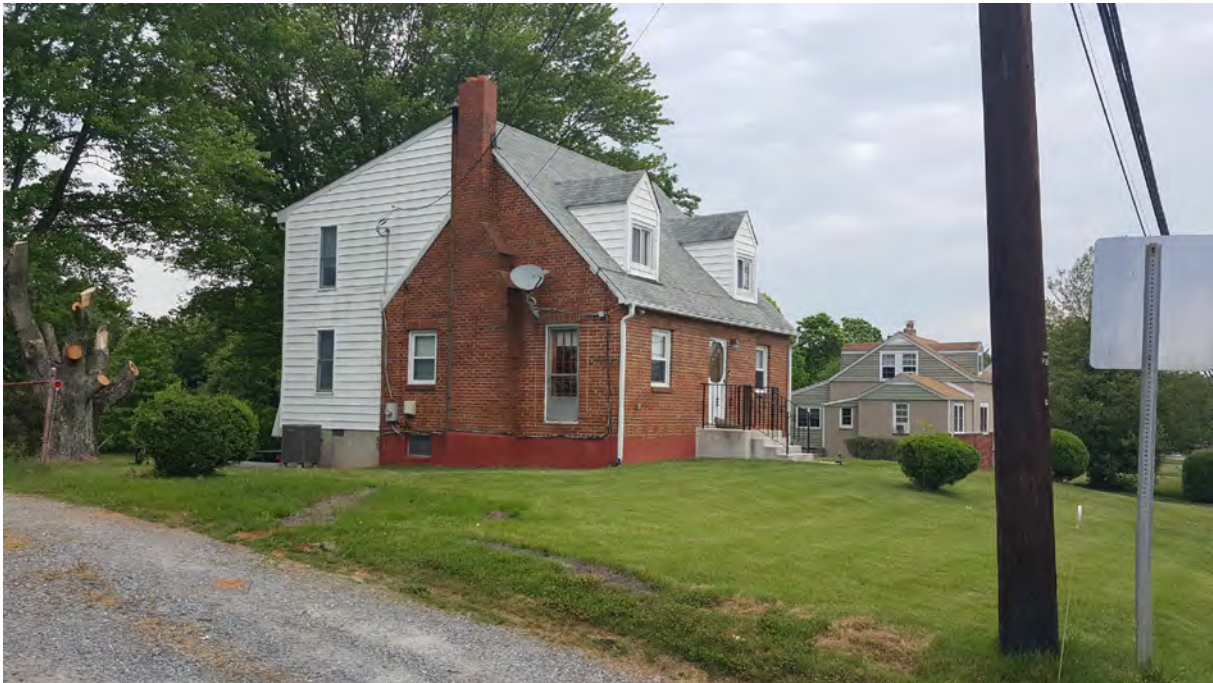
Photo 2 - Oblique view of primary elevation, 5418 Odell Road, Looking Northeast
