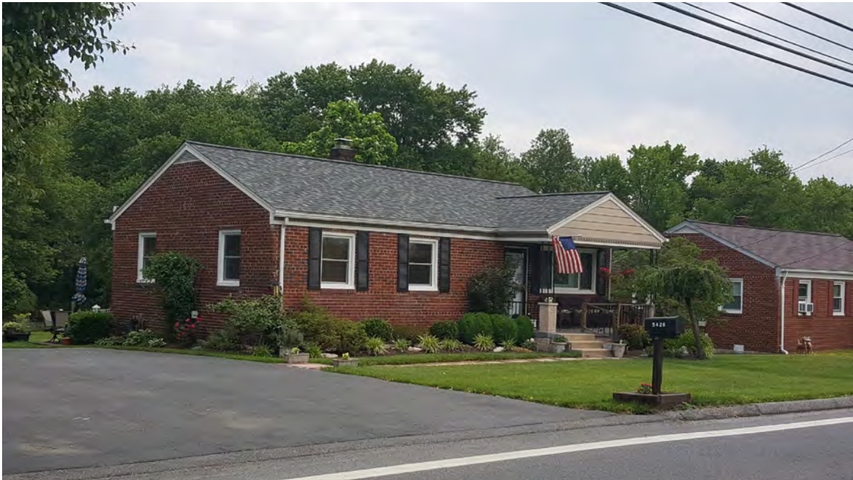
Photo 2 - Oblique view of primary elevation, 5426 Odell Road, Looking Northeast
