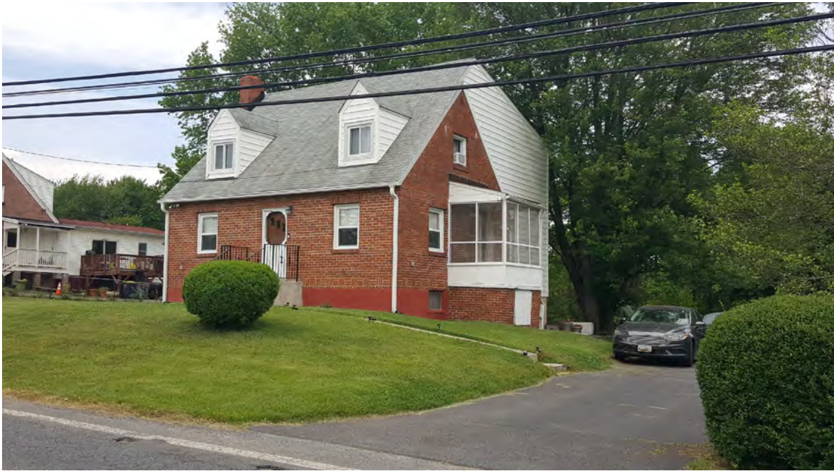
Photo 3 - Oblique view of primary elevation, 5418 Odell Road, Looking Northwest
