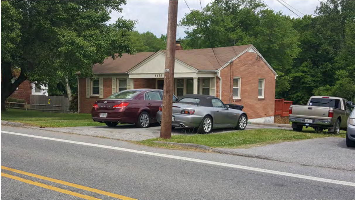
Photo 3 - Oblique view of primary elevation, 5434 Odell Road, Looking Northwest
