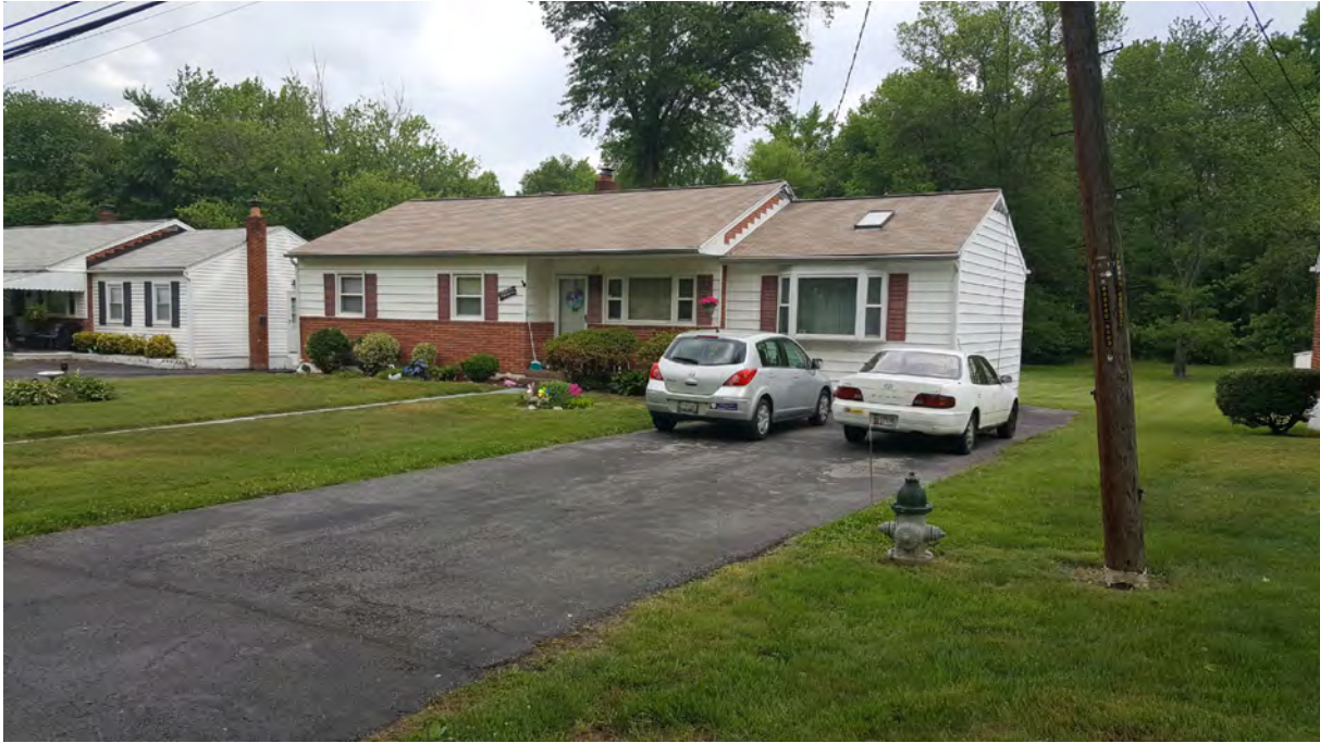
Photo 3 - Oblique view of primary elevation, 5606 Odell Road, Looking Northwest
