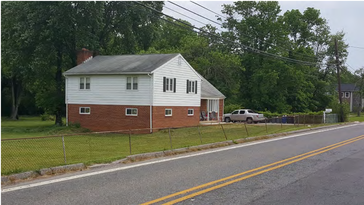
Photo 2 -Oblique view of primary elevation, 5440 Odell Road, Looking Northeast
