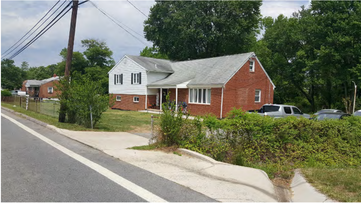
Photo 3 - Oblique view of primary elevation, 5440 Odell Road, Looking Northwest
