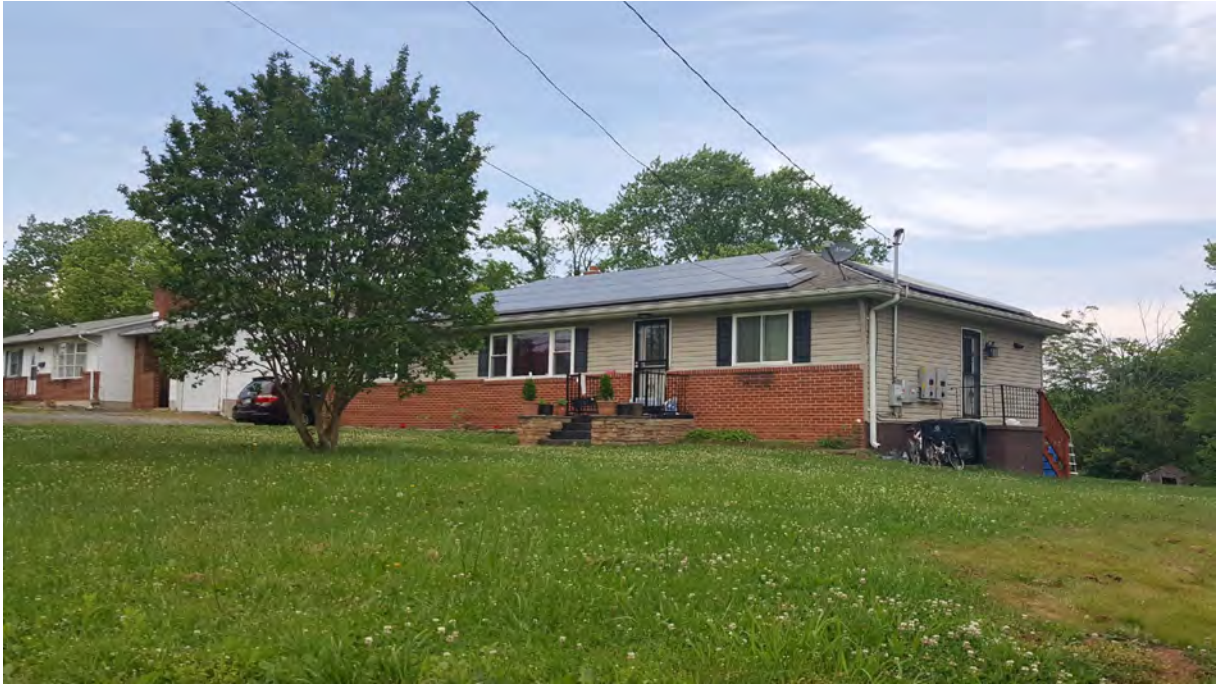
Photo 3 - Oblique view of primary elevation, 5410 Odell Road, Looking Northwest
