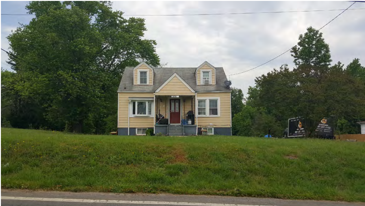
Photo 1 - Primary (south) elevation, 5414 Odell Road, Looking North
