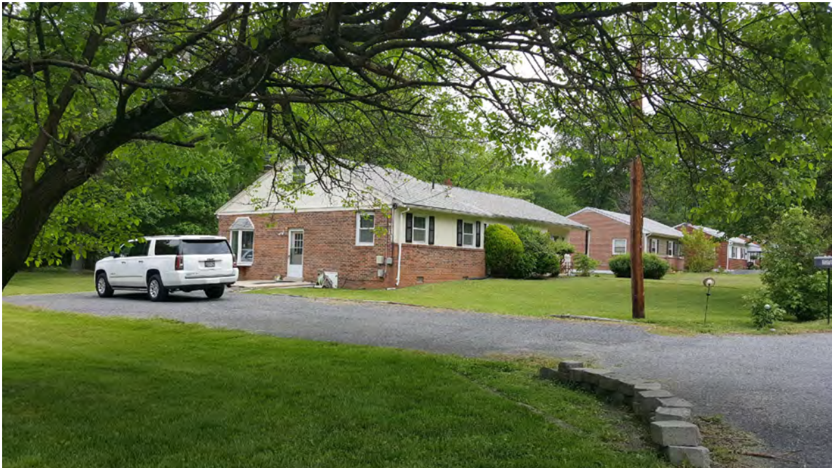
Photo 2 - Oblique view of primary elevation, 5600 Odell Road, Looking Northeast
