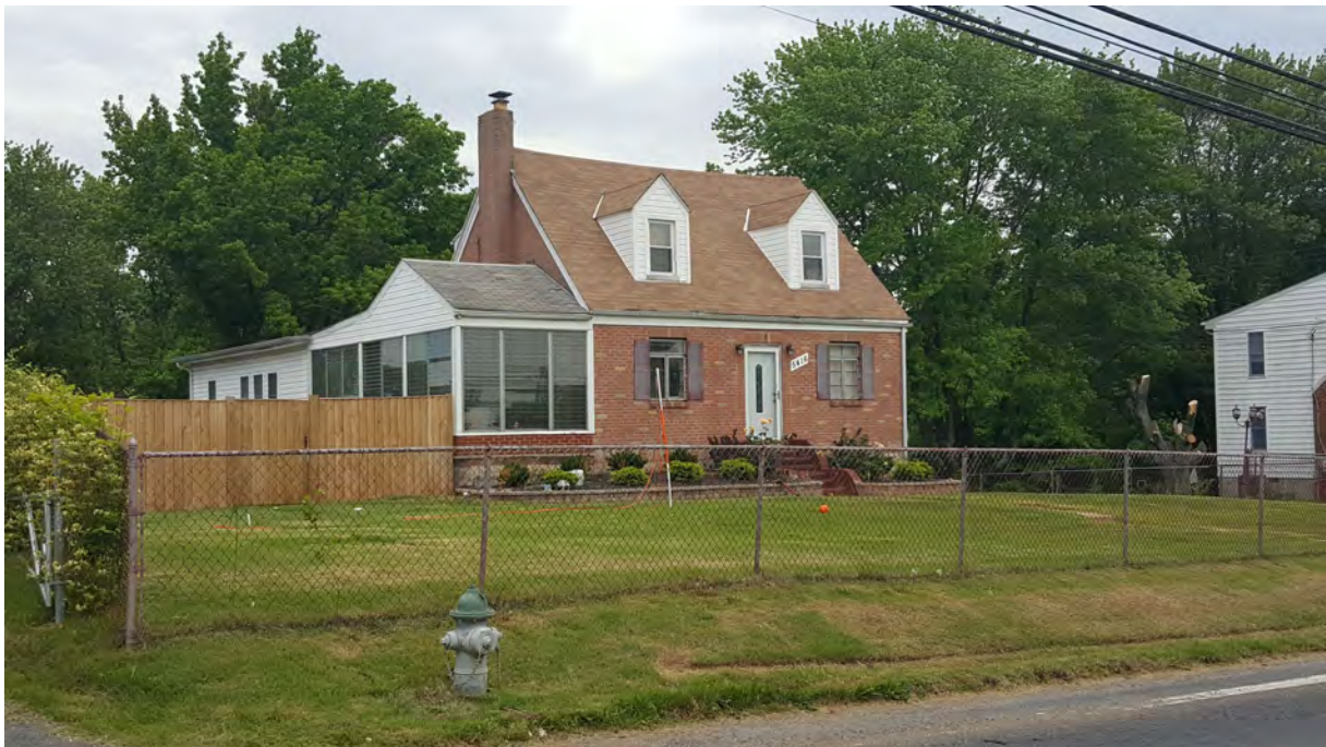
Photo 2 - Oblique view of primary elevation, 5416 Odell Road, Looking Northeast
