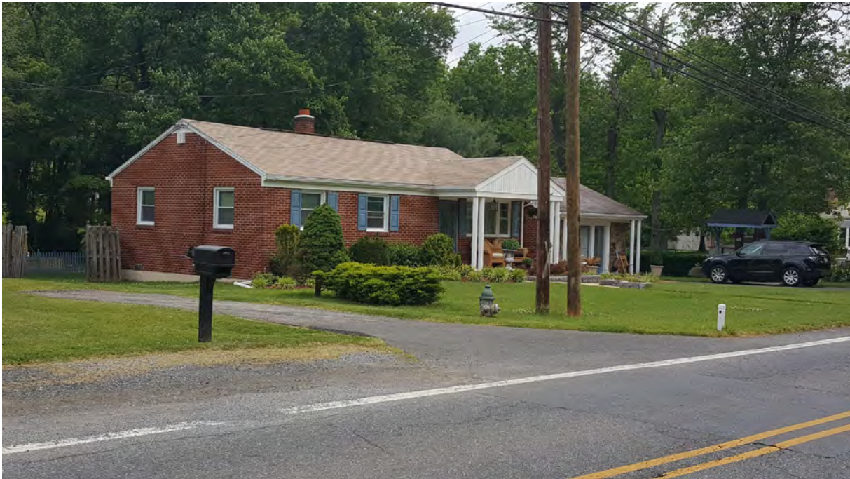
Photo 2 - Oblique view of primary elevation, 5516 Odell Road, Looking Northeast
