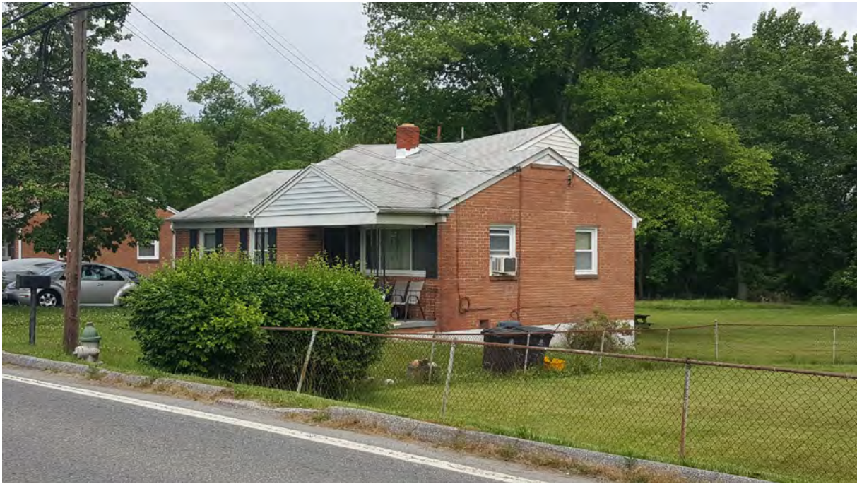
Photo 3 - Oblique view of primary elevation, 5438 Odell Road, Looking Northwest
