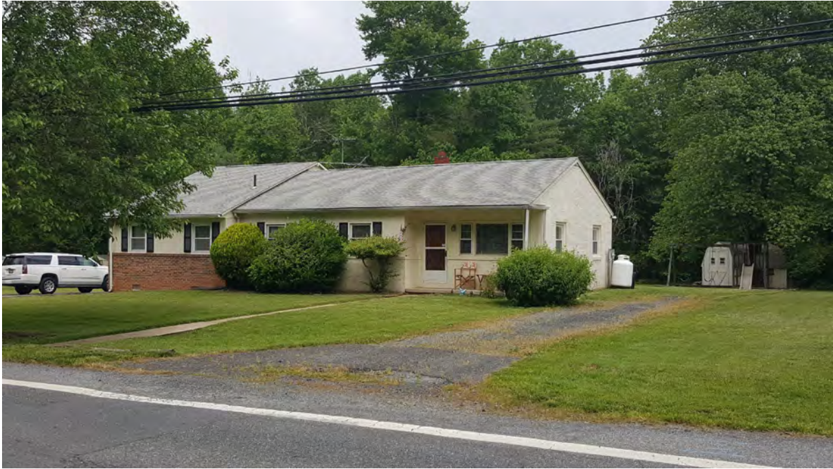
Photo 3 - Oblique view of primary elevation, 5600 Odell Road, Looking Northwest
