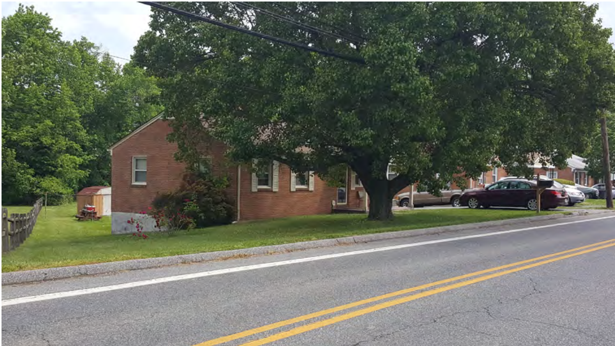
Photo 2 - Oblique view of primary elevation, 5434 Odell Road, Looking Northeast
