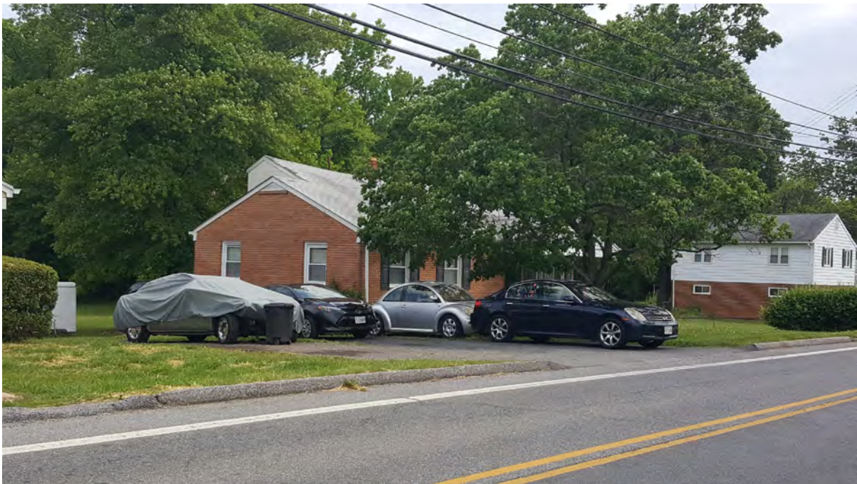
Photo 2 - Oblique view of primary elevation, 5438 Odell Road, Looking Northeast
