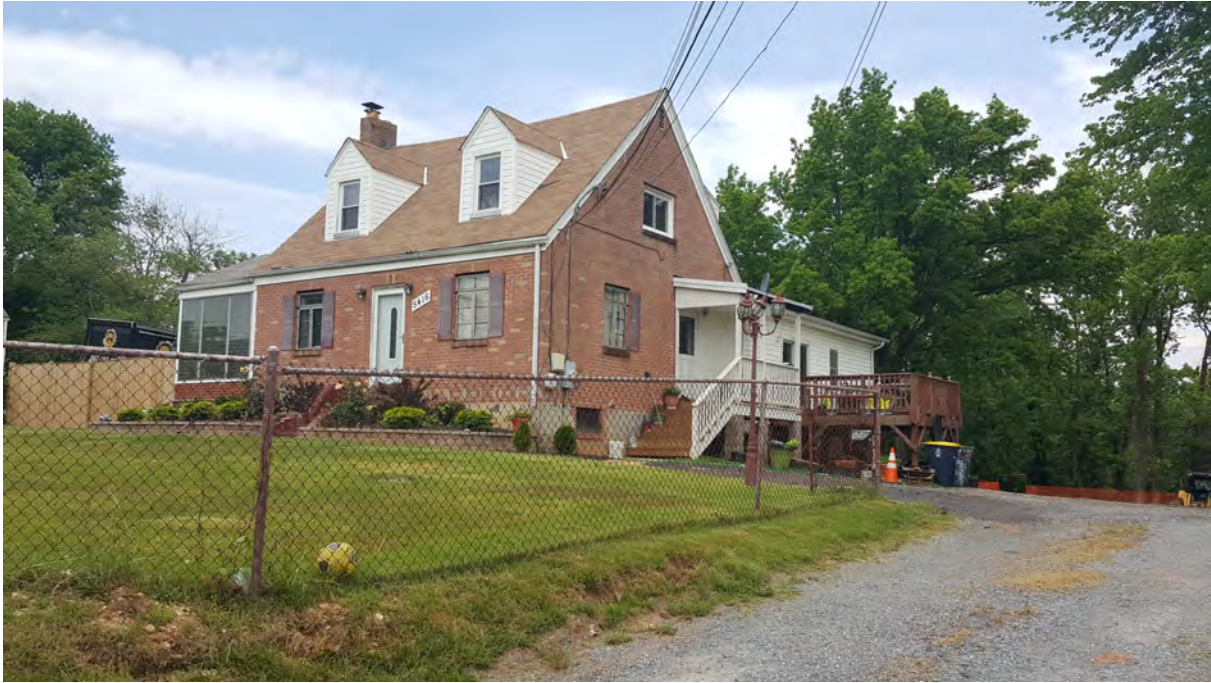
Photo 3 - Oblique view of primary elevation, 5416 Odell Road, Looking Northwest
