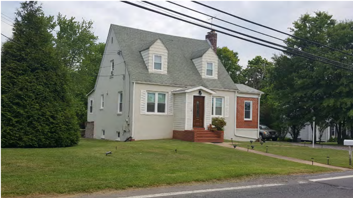
Photo 2 - Oblique view of primary elevation, 5422 Odell Road, Looking Northeast
