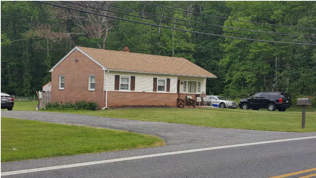
Photo 2 - Oblique view of primary elevation, 5610 Odell Road, Looking Northeast
