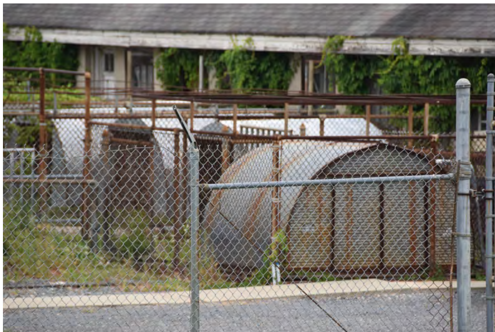
Photo 1 - Pig Shelters, Central Farm, General View of Pig Shelters, Looking West
