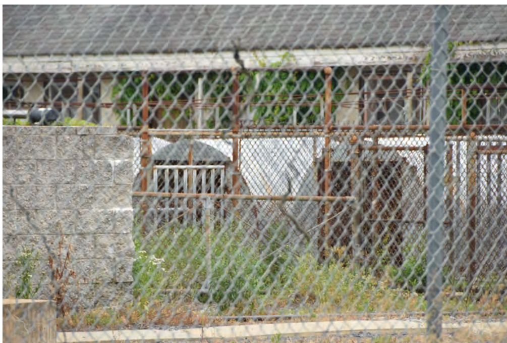
Photo 2 - Pig Shelters, Central Farm, General View of Pig Shelters, Looking West
