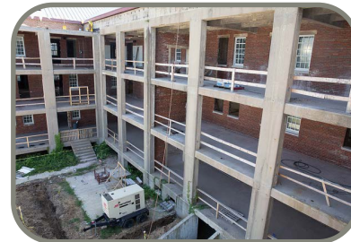
Hale Hall Renovation Fort Meade, MD
