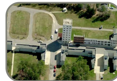
J.J. Rowley Training Center Upgrades
