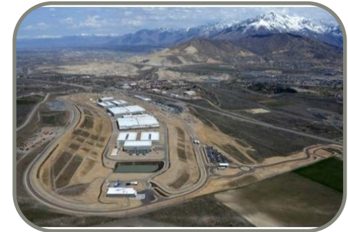
Utah Data Center
