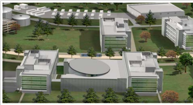
Joint Operations Center
