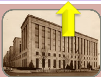
Bureau of Engraving & Printing Advise, design and construct new printing facility in Beltsville, MD
