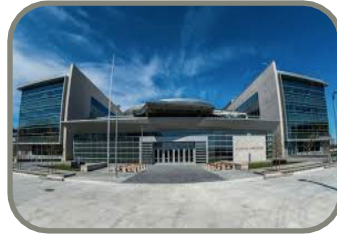
National Security Agency East Campus $7B program
