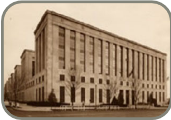
Bureau of Engraving & Printing Advise, design and construct new printing facility in Beltsville, MD
