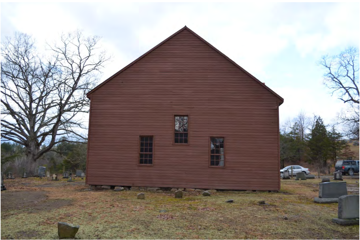
Photo 3: East Elevation of Old Pine Church, Camera Facing West
