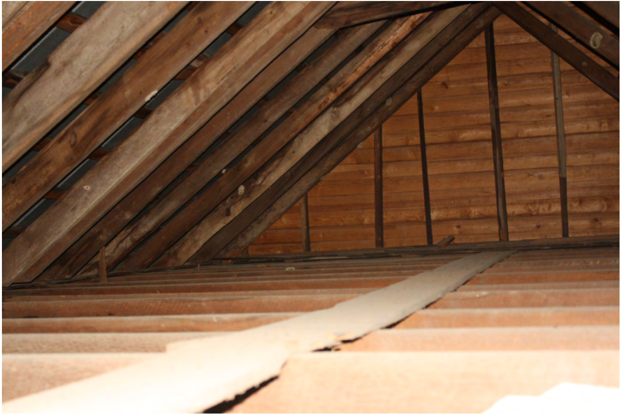
Photo 17: Interior of Attic Space, Facing East
