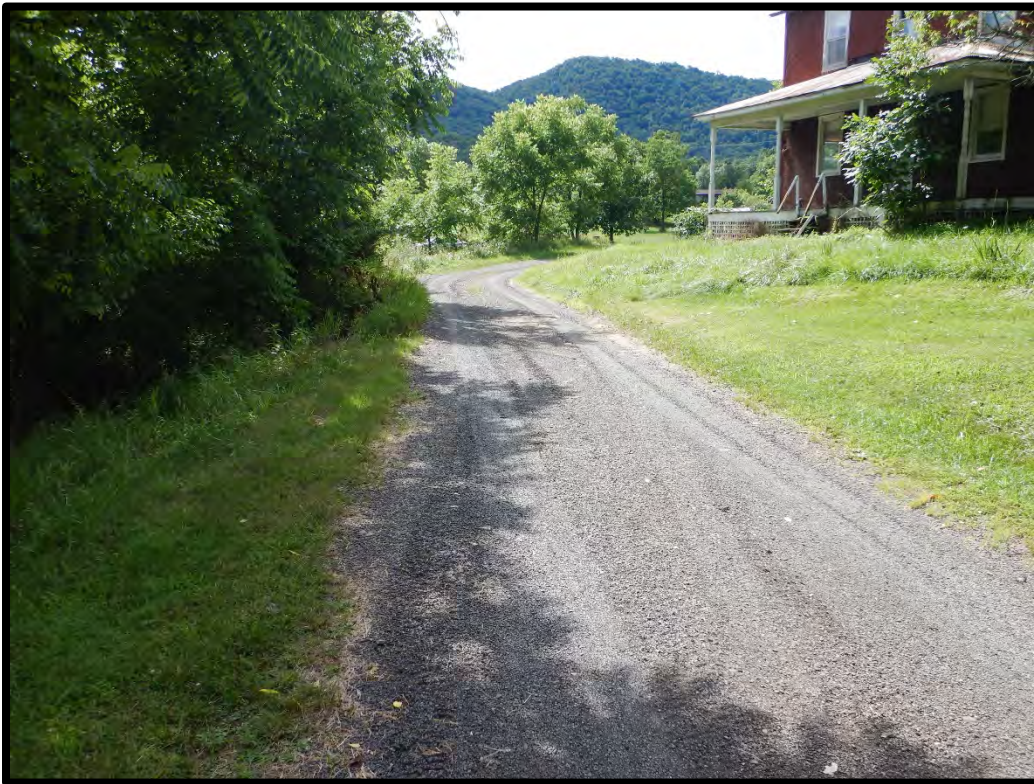
Figure 31. View of conditions within the project area looking southeast along Grove Road.
