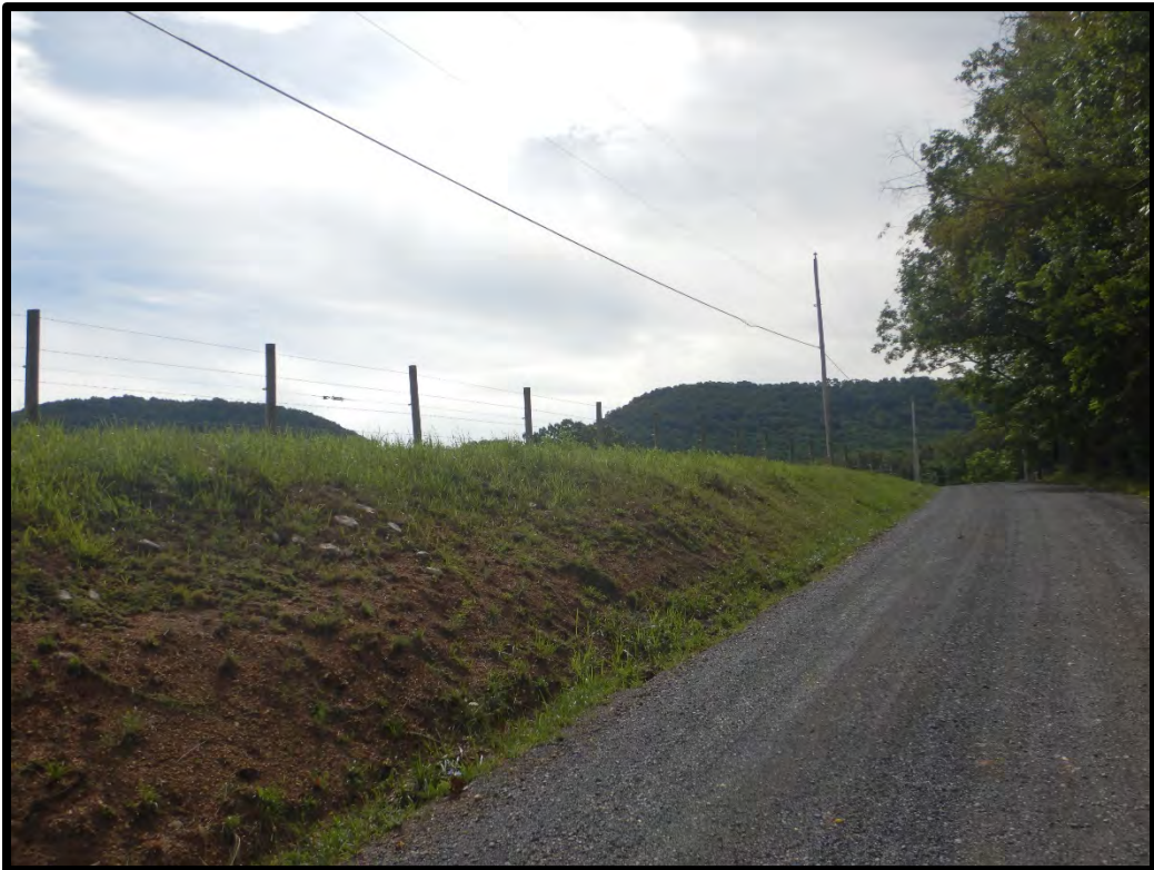
Figure 27. View of conditions within the project area looking east along Hickory Hill Road.
