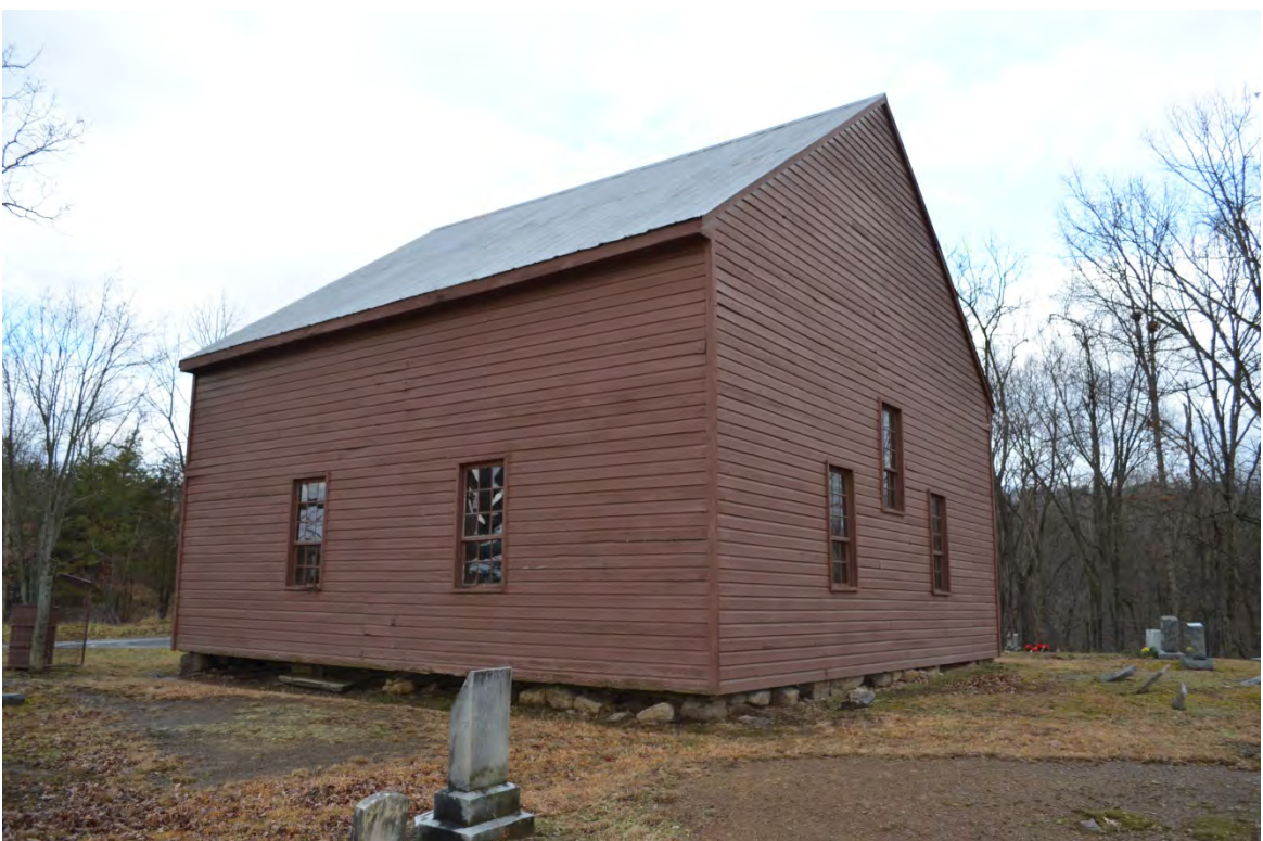
Photo 4: South and East Elevations, Camera Facing Northwest
