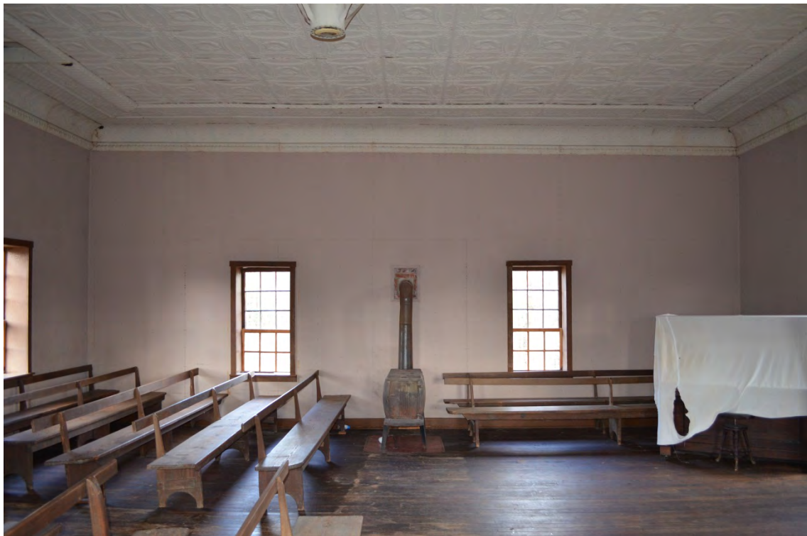
Photo 14: Interior of North Elevation, Facing North
