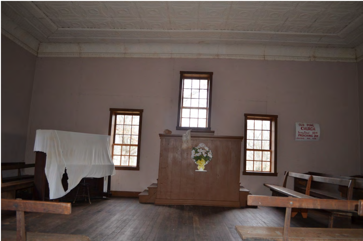
Photo 12: East Elevation, Interior, Facing East
