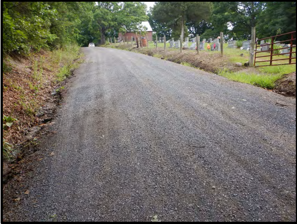
Figure 24. View of conditions looking north along Old Pine Church Road adjacent to cemetery.
