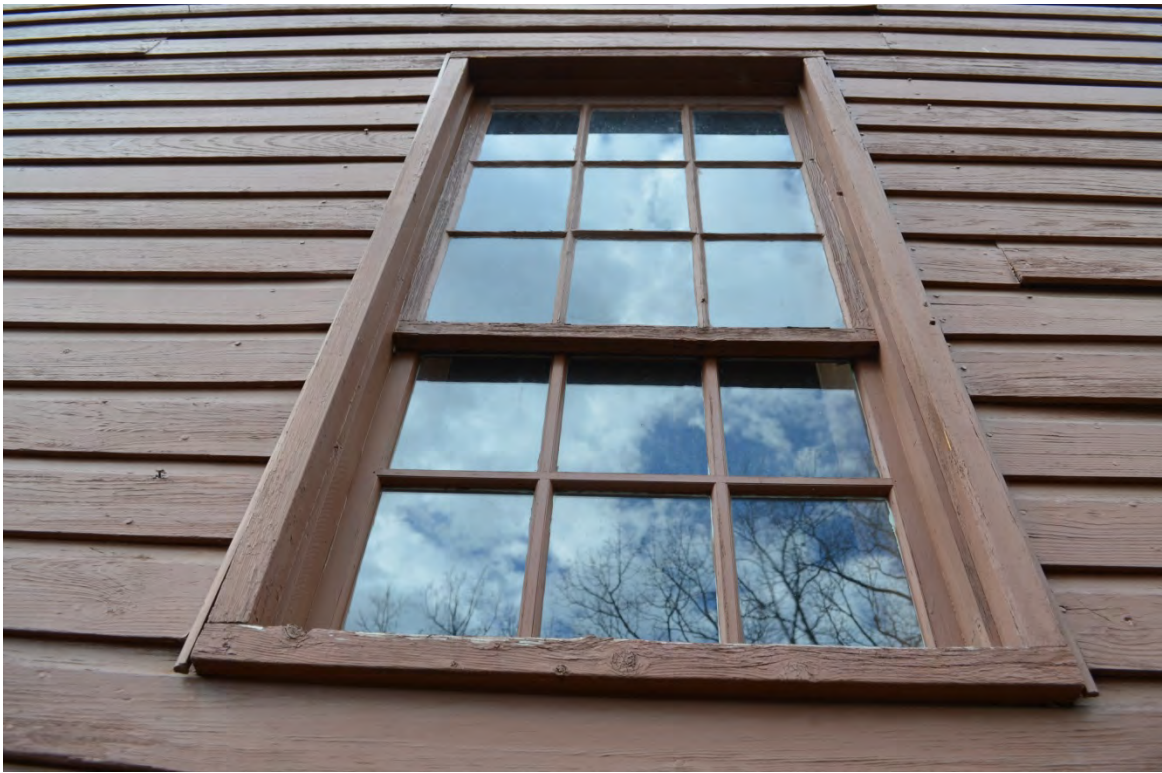
Photo 11: Detail of Window, East Elevation, Facing West
