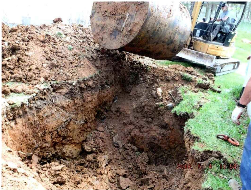
Figure 1 1,000 gallon tank removal
