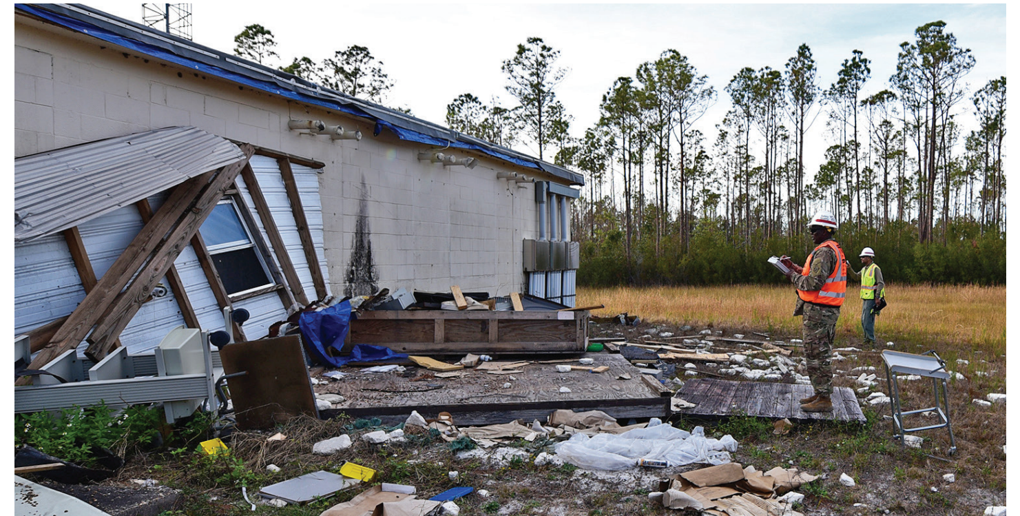
71st Detachment, Forward Engineer Support Team - Advance (FEST-A) conducts infrastructure assessments on Tyndall Air Force Base in Florida following Hurricane Michael. (Photos courtesy of Tyndall AFB)
