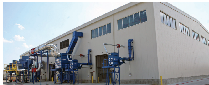
Exterior shot of the Metal Treatment Annex at the northeast corner of Building 350 that houses a wash bay, metal treatment tanks, sanding area, blast booths and surface repair areas. Sept. 7, 2018. (Photo courtesy of Pam Goodhart, Letterkenny Army Depot)
