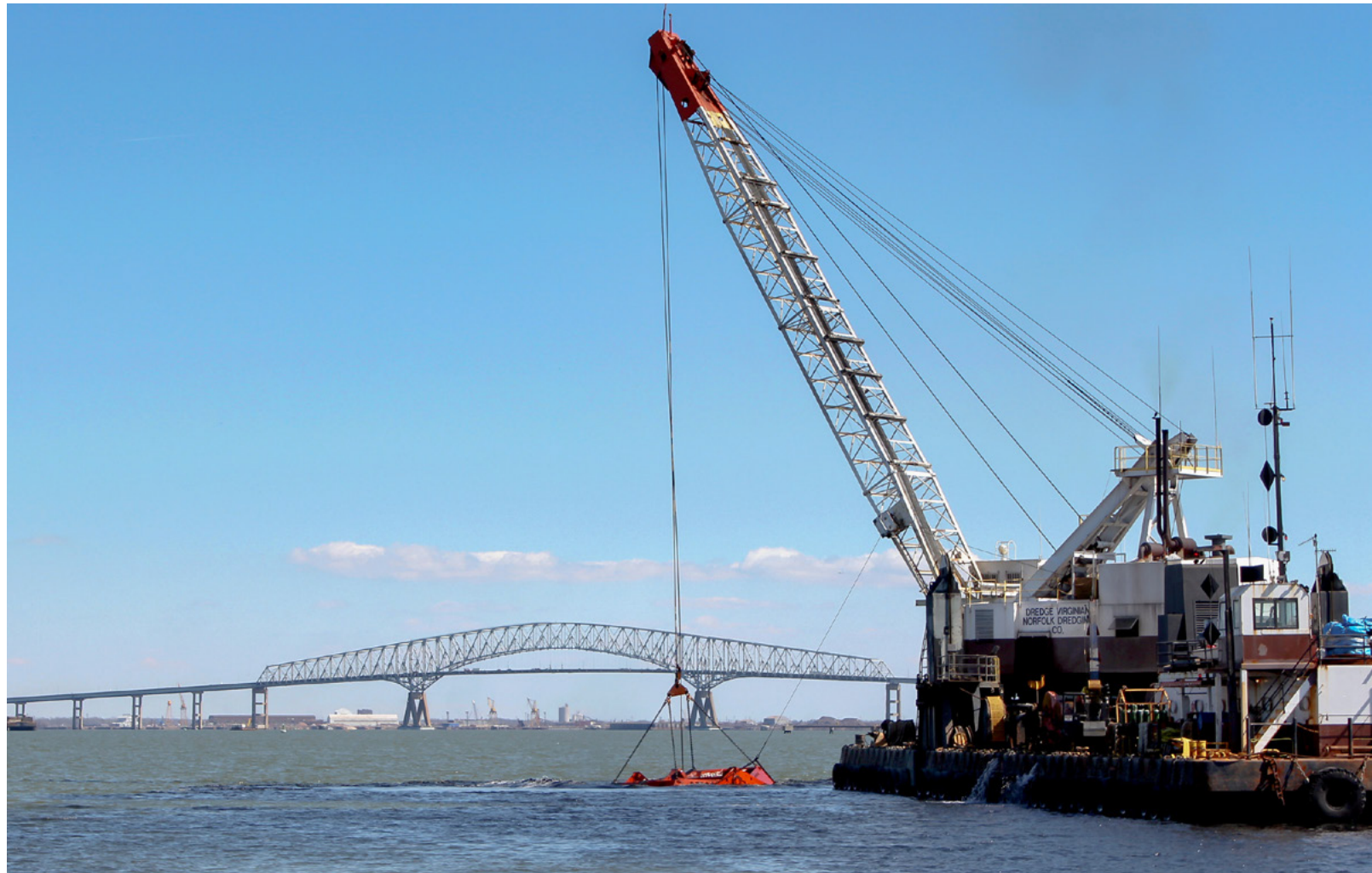
An Army Corps contracted dredge operated by Norfolk Dredging lifts material out of Curtis Bay Channel in Baltimore Harbor. (U.S. Army photo by Chris Gardner)
