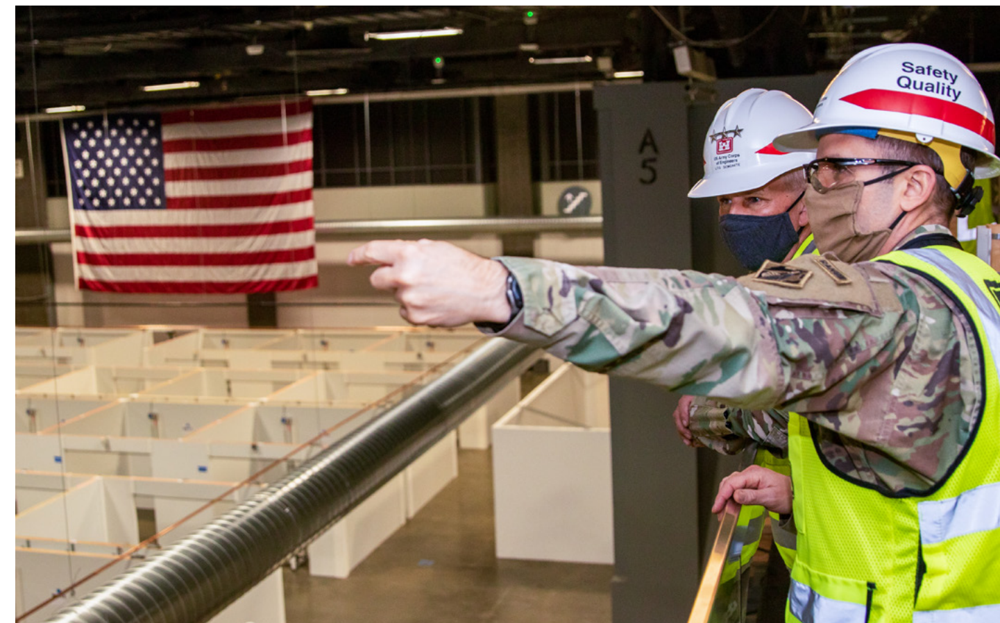
Col. John Litz, commander of the U.S. Army Corps of Engineers, Baltimore District, highlights aspects of construction of the alternate care facility in the Walter E. Washington Convention Center in Washington, D.C., to Lt. Gen. Todd T. Semonite, U.S. Army Corps of Engineers commanding general, April 30, 2020. The U.S. Army Corps of Engineers, Baltimore District, using funds through FEMA, awarded a contract on April 16, 2020, to Hensel Phelps Construction Co. out of Tyson, Virginia, and both the design and construction of the facility were completed in just 22 days. The alternate care facility was requested by D.C.'s Homeland Security and Emergency Management Agency through FEMA to address potential shortages in hospital beds in the event of a surge of patients needing care in the District of Columbia. (U.S. Army photo by Carlos J. Lazo)
