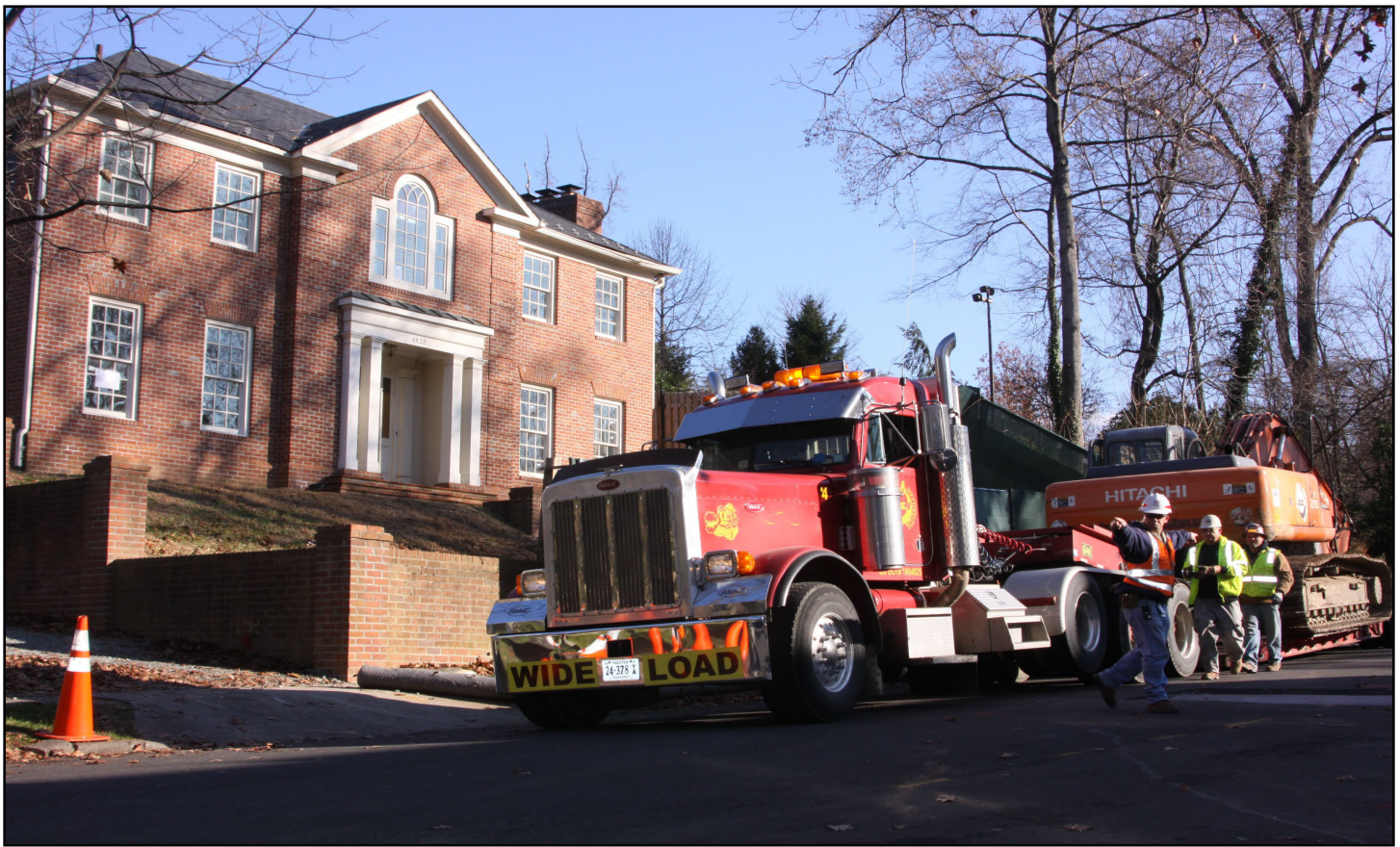
The crew arrives to prepare the 4825 Glenbrook Road property for demolition. Photo by Brittany Bangert
