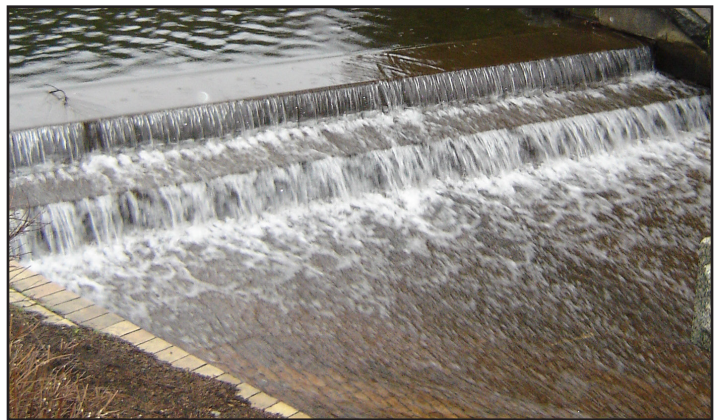
The Lusk Dam and Reservoir at the U.S. Military Academy, West Point, N.Y. Photo by Larry Mathena
