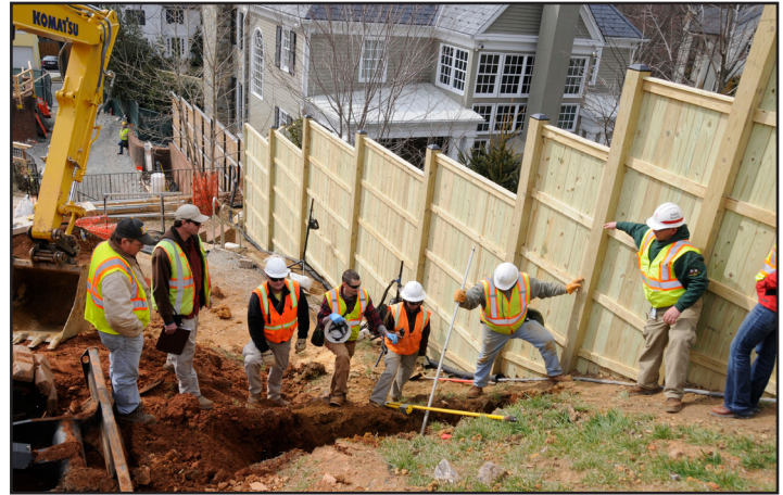
Crews excavate the last test pit as part of the initial low probability work at 4825 Glenbrook Road.
