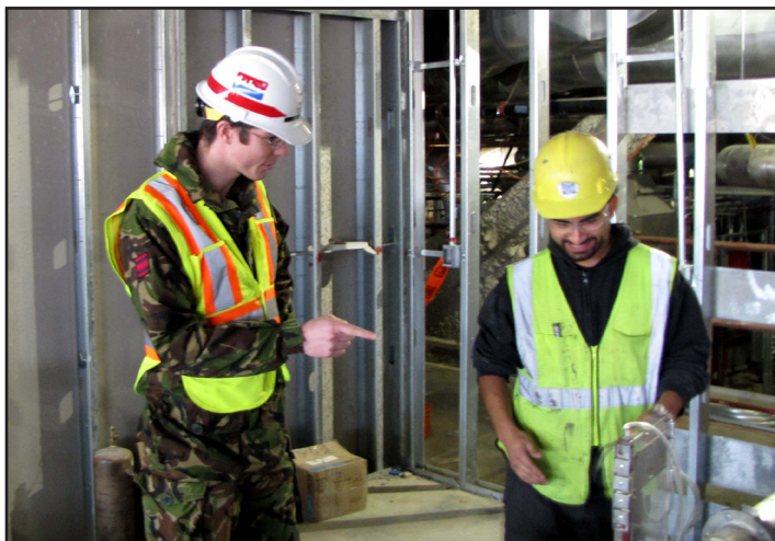
Capt. Ben Hancock (left) works with a Fort Detrick contractor to test ducts at the U.S. Army Medical Research Institute for Infectious Diseases project to ensure containment and that all specifications are met as part of the quality assurance process.
