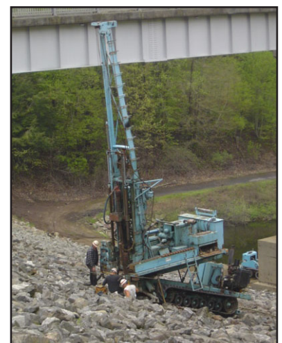
FEU technicians Albert McNamara (left), John Blackson and Doug Baughman work on the slope of the Hop Brook dam (New England District) investigating the embankment and foundation materials. Photo by Maria Orosz
