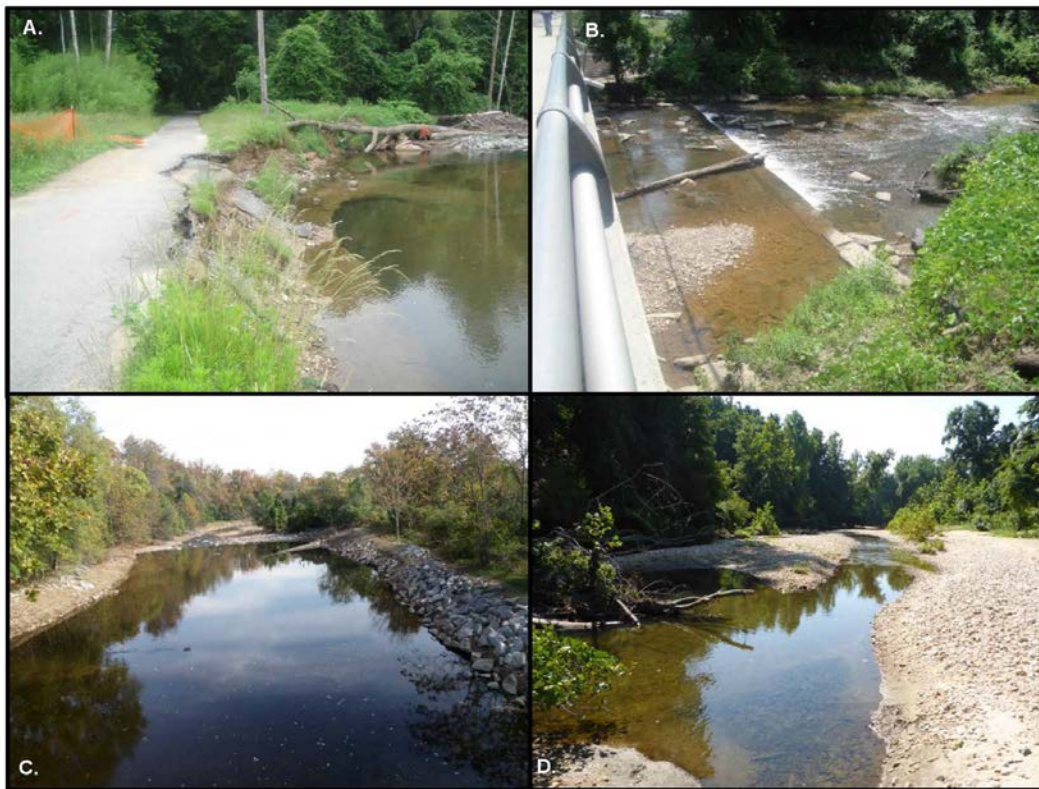
Figure 1-11. Problems in the study stream reaches. A. Erosion along study stream reach (site 13) undermining a pedestrian trail system. B. Concrete sill inhibiting fish migration upstream on Northwest Branch (site 3). C. Homogeneous habitat conditions as a result of USACE channelization (site 3). D. Excess sediment deposition and formation of large sediment bars (site 5).
