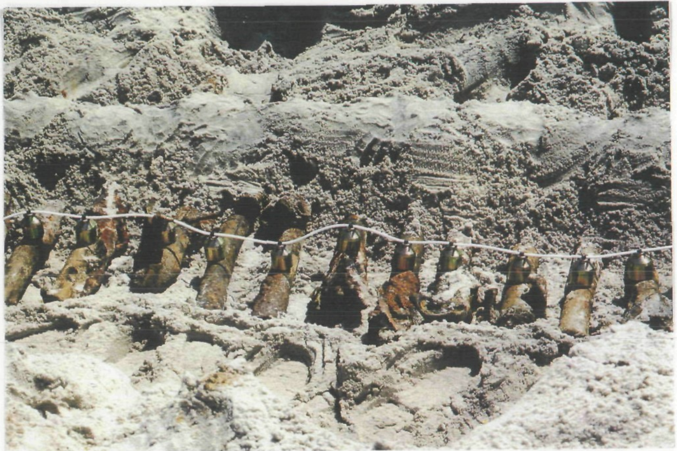
The detonating cord is strung through each perforator and then attached to a blasting cap.
