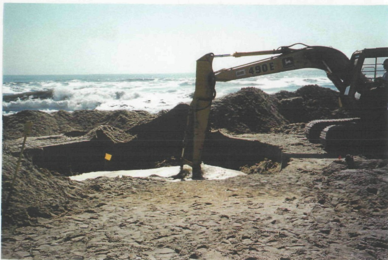
The track hoe was able to dig below the water table and remove the practice ordnance.
