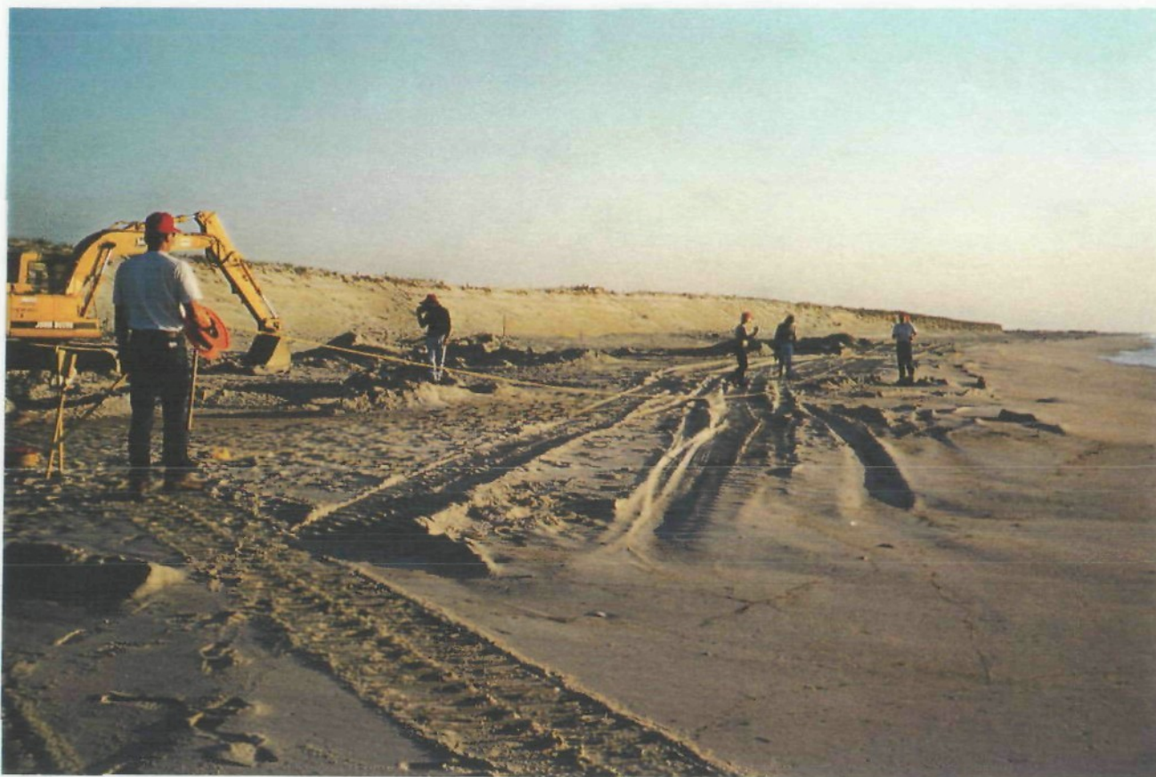
Clearance operations begin by laying out search lanes with ropes.
