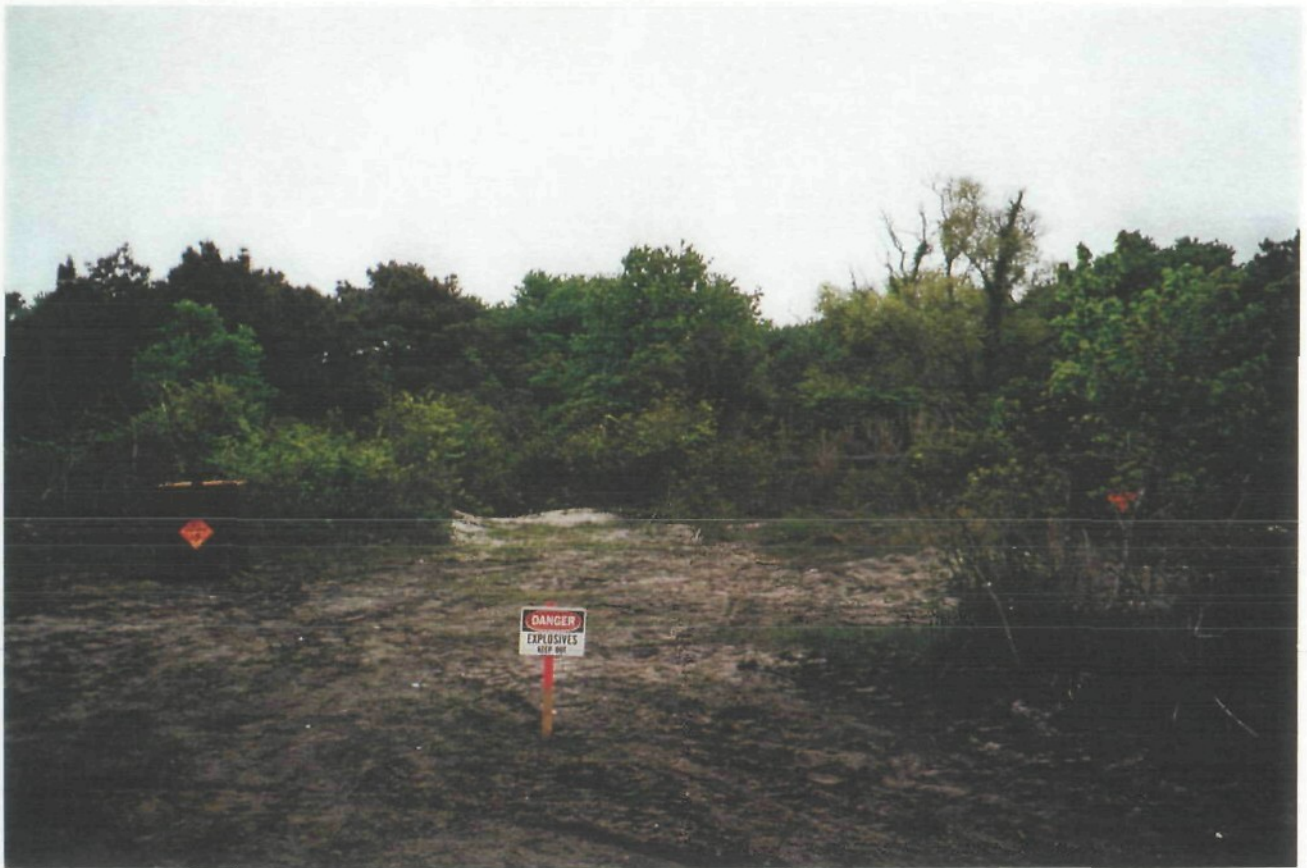
Prior to conducting any intrusive operations an explosive storage magazine was placed in a remote and secure area.
