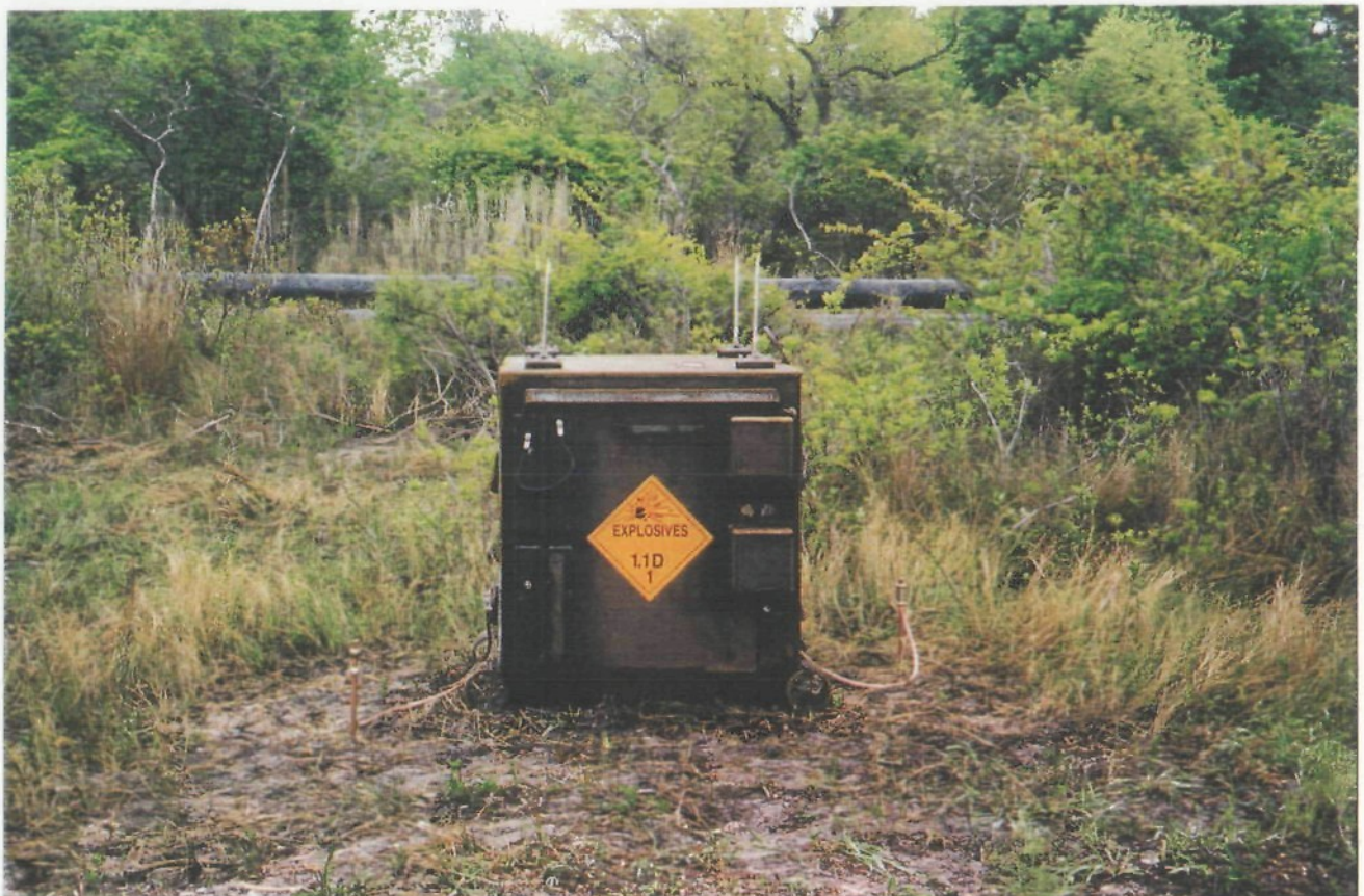
The magazine was grounded and certified by a licensed electrician. Note the four antennas on top of the magazine, and the two grounding rods in the ground.
