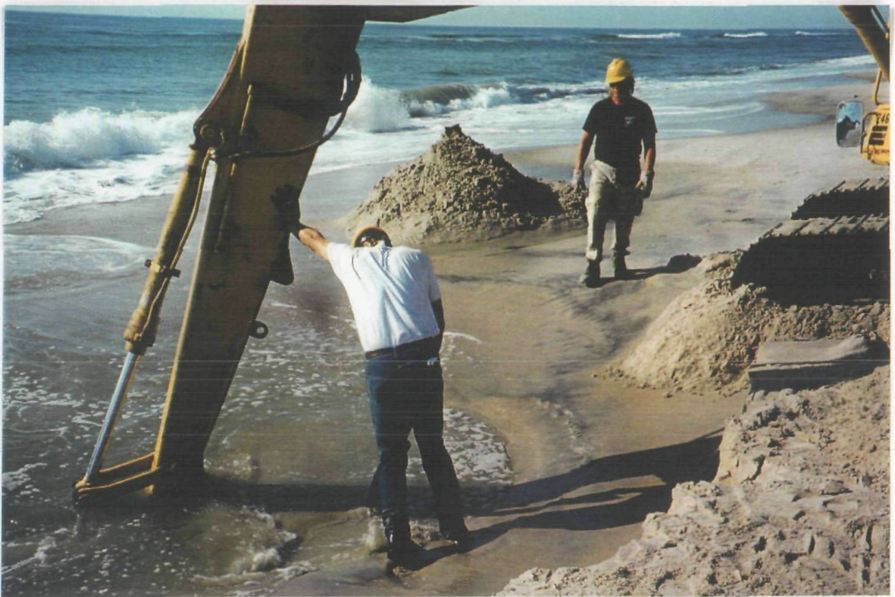
The track hoe dug up a practice 5 inch warhead and one of the UXO Specialist is removing it from the hole.
