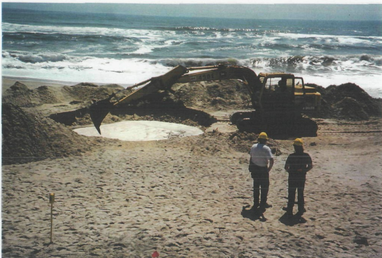
When large anomalies were discovered, a track hoe was used to investigate.
