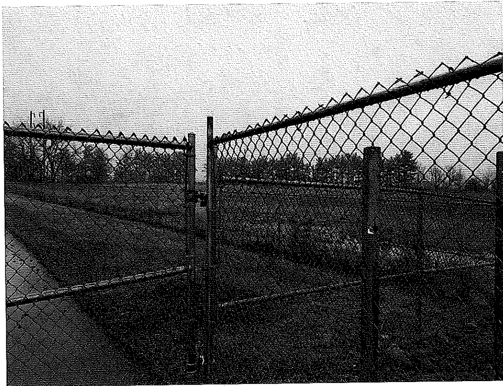
Photograph 2 – Bio retention basin on the southern portion of Area I
