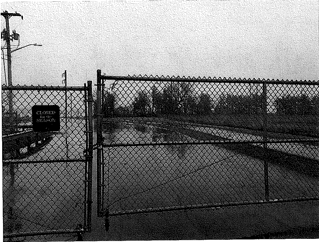
Photograph 1 – Entrance to Frankford Boat Launch
