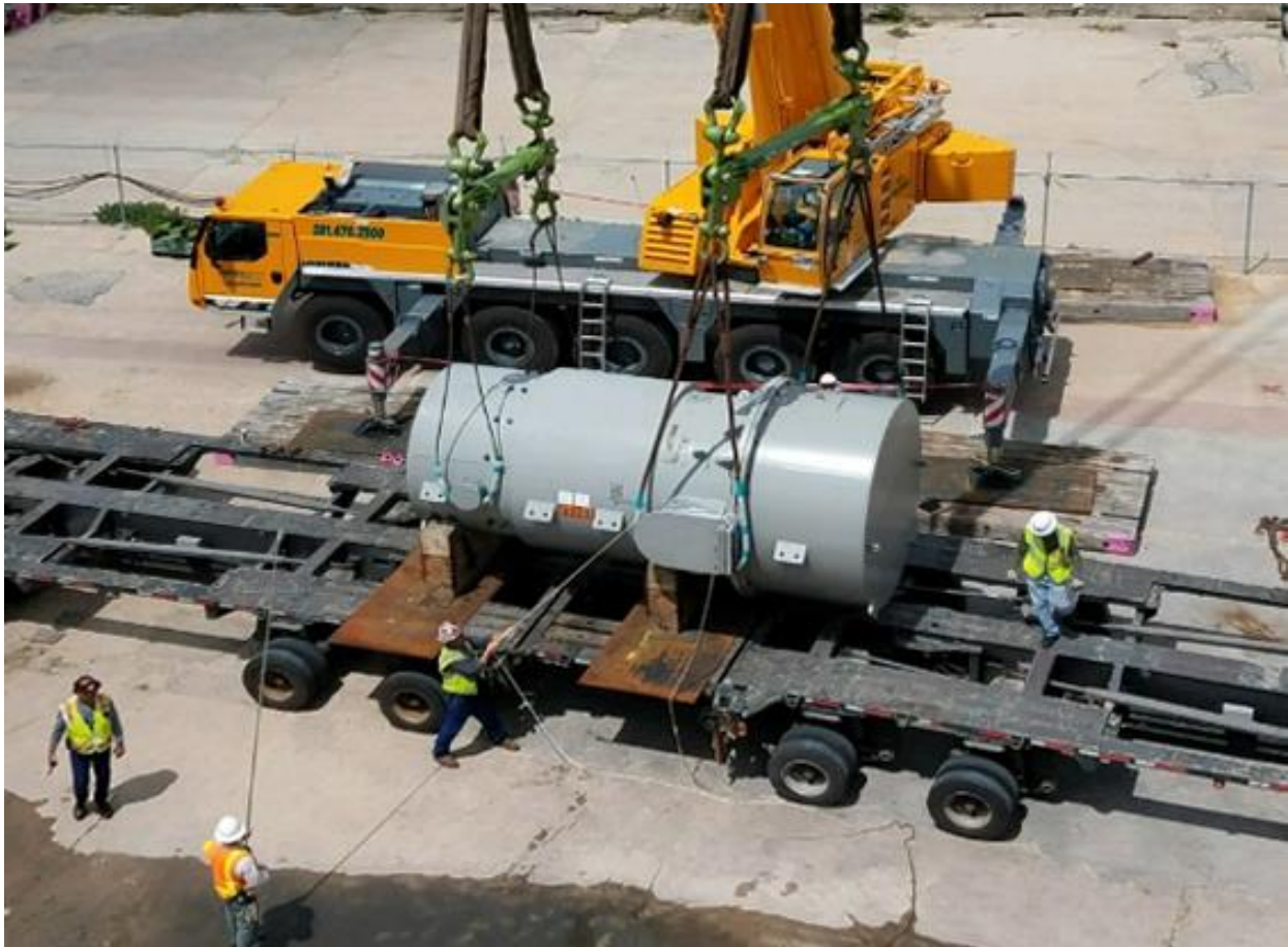
Figure 26. MH-1A Reactor Pressure Vessel being loaded for shipment at Port of Galveston, 2018.
