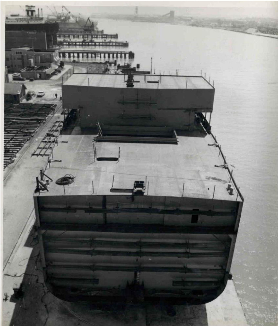
Figure 20. Completed MH-1A mid-body, ready for launching, 1 April 1964 (USACE Baltimore's MH-1A STURGIS Digitized Historical Documents Archive at http://www.nab.usace.army.mil/Missions/Environmental/Sturgis.aspx )
