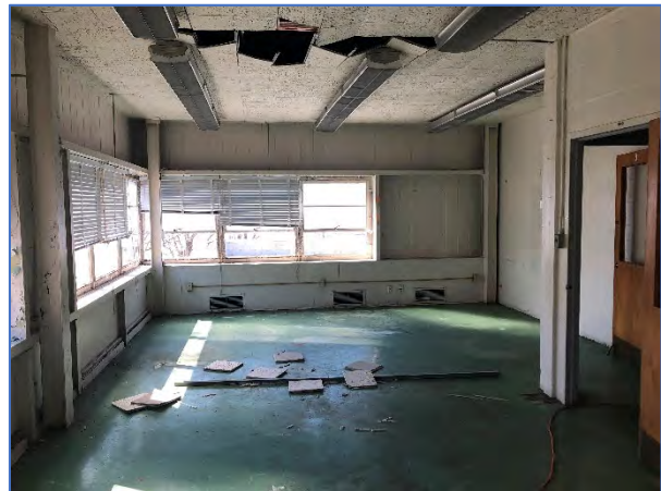
Existing interior space condition in Building 372.
