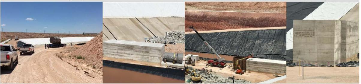
RPV and Shielded Container are Moved into the Waste Control Specialists Federal Waste Facility Disposal Cell and Encased in Concrete
