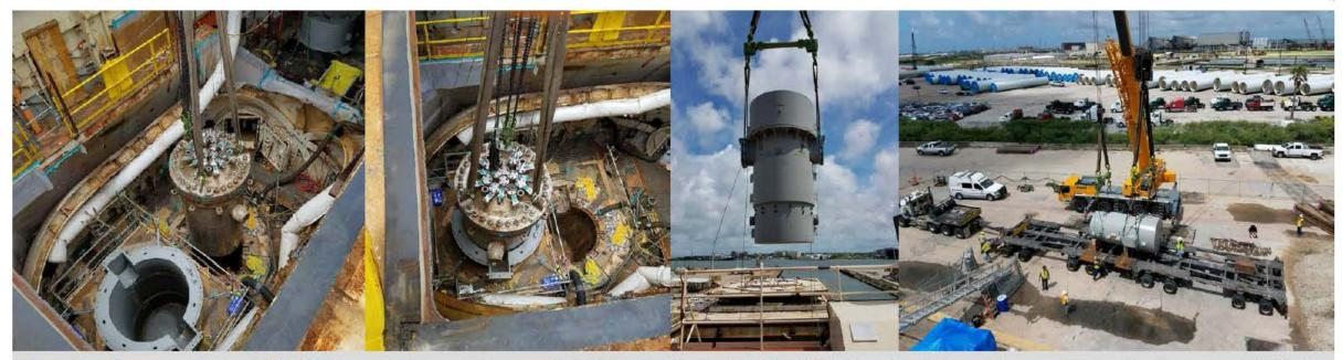
Reactor Pressure Vessel (RPV) Removed from Primary Shield Tank, Sealed in the Shielded Container, Secured onto the Transport Vehicle
