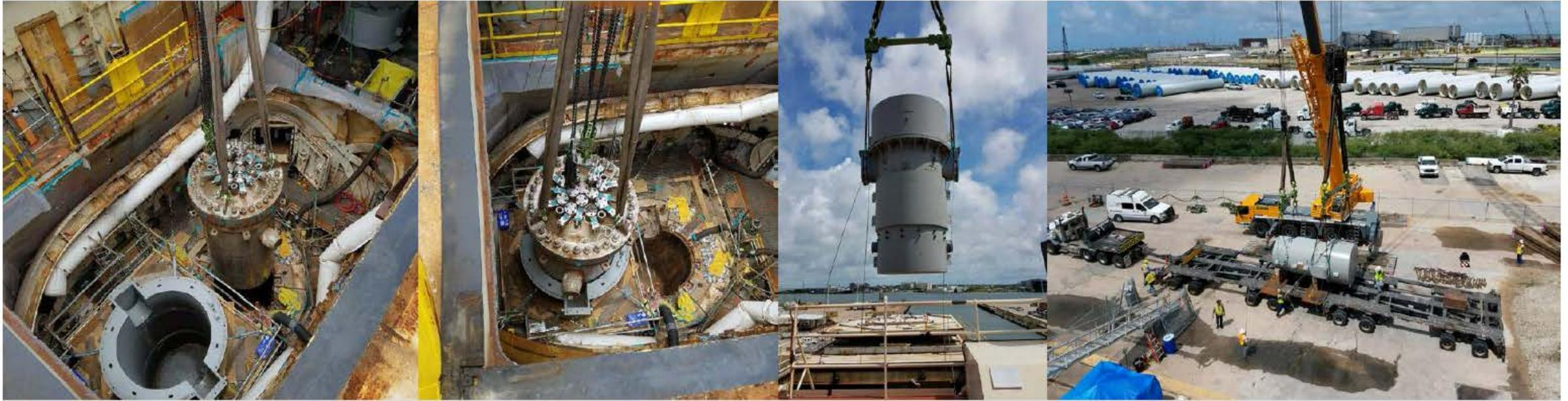
Reactor Pressure Vessel (RPV) Removed from Primary Shield Tank, Sealed in the Shielded Container, Secured onto the Transport Vehicle
