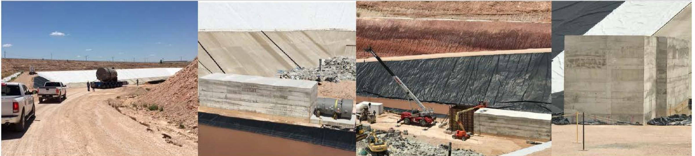
RPV and Shielded Container are Moved into the Waste Control Specialists Federal Waste Facility Disposal Cell and Encased in Concrete
