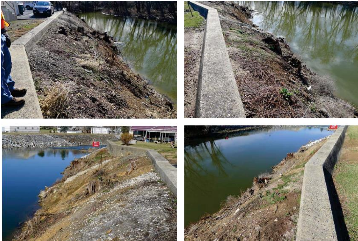
Photograph 3. Site of Alternative 2.C: Riprap Installation near South Richland Avenue Bridge
