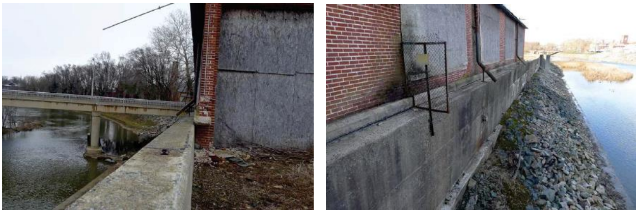
Photograph 1. Site of Alternative 2.A: Floodwall Replacement near Penn Street Bridge
