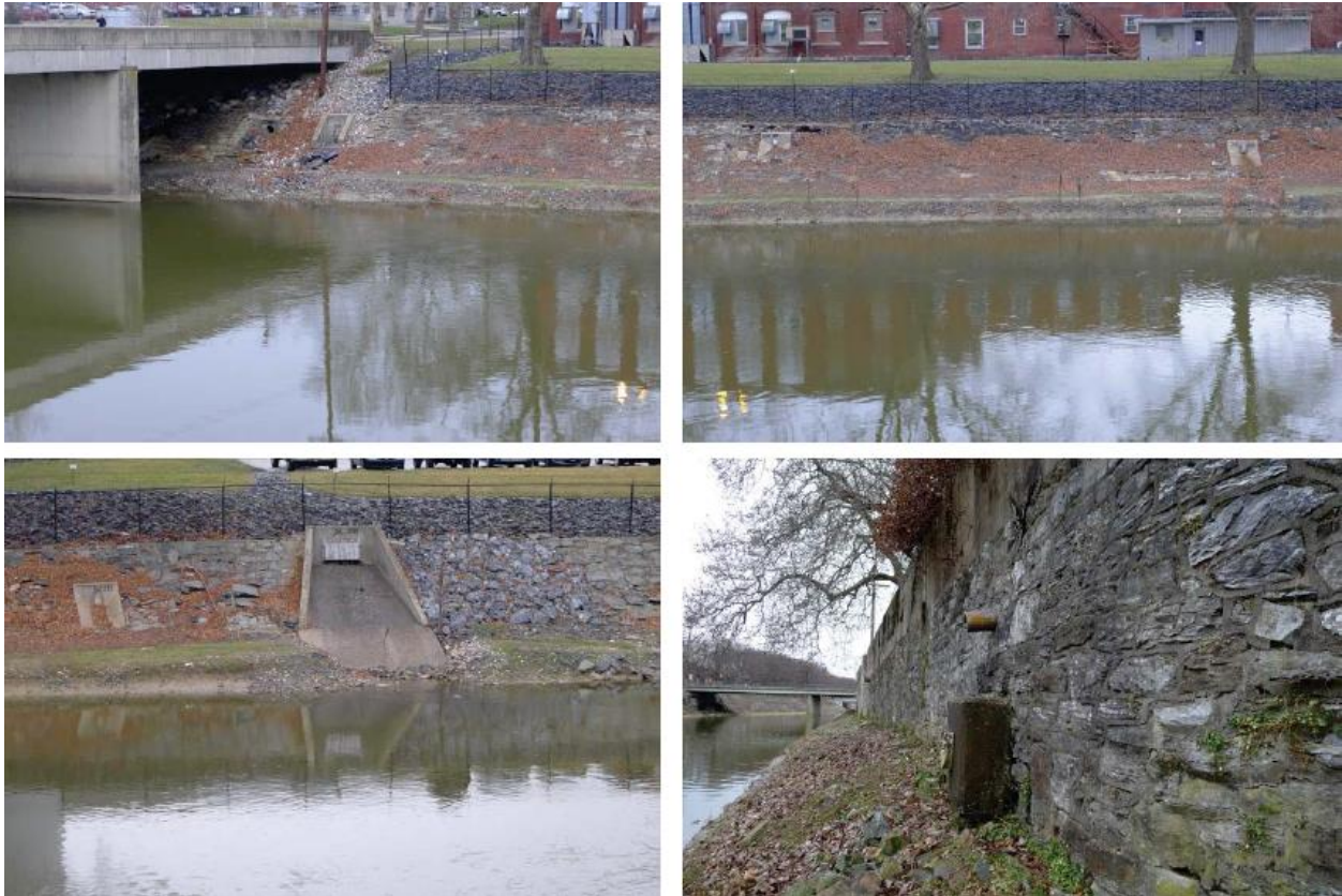
Photograph 4. Examples of Alternative 2.D: Drainage Conduit Maintenance
