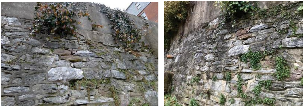
Photograph 2. Site of Alternative 2.B: Bulge Repairs near Market Street Bridge
