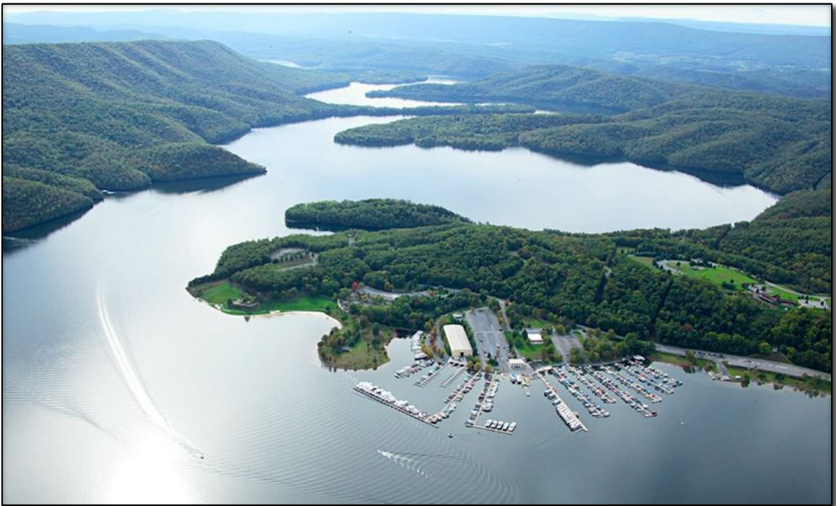
Figure 5.2 The Seven Points Marina, a leased facility (USACE Photo).
