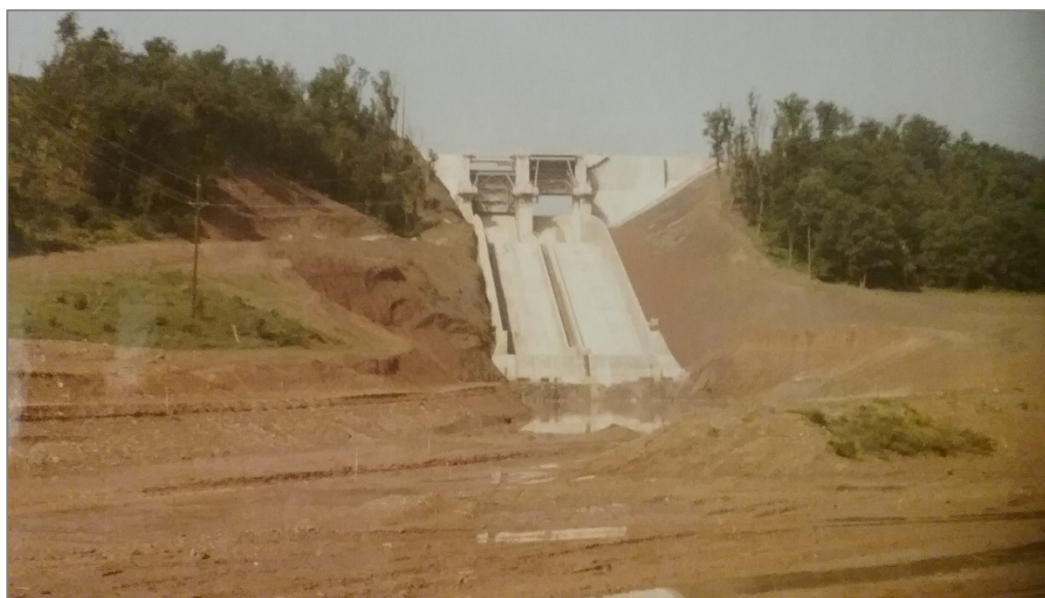
Figure 5.1 Construction of Raystown Lake Spillway, early 1970s (USACE Photo).
