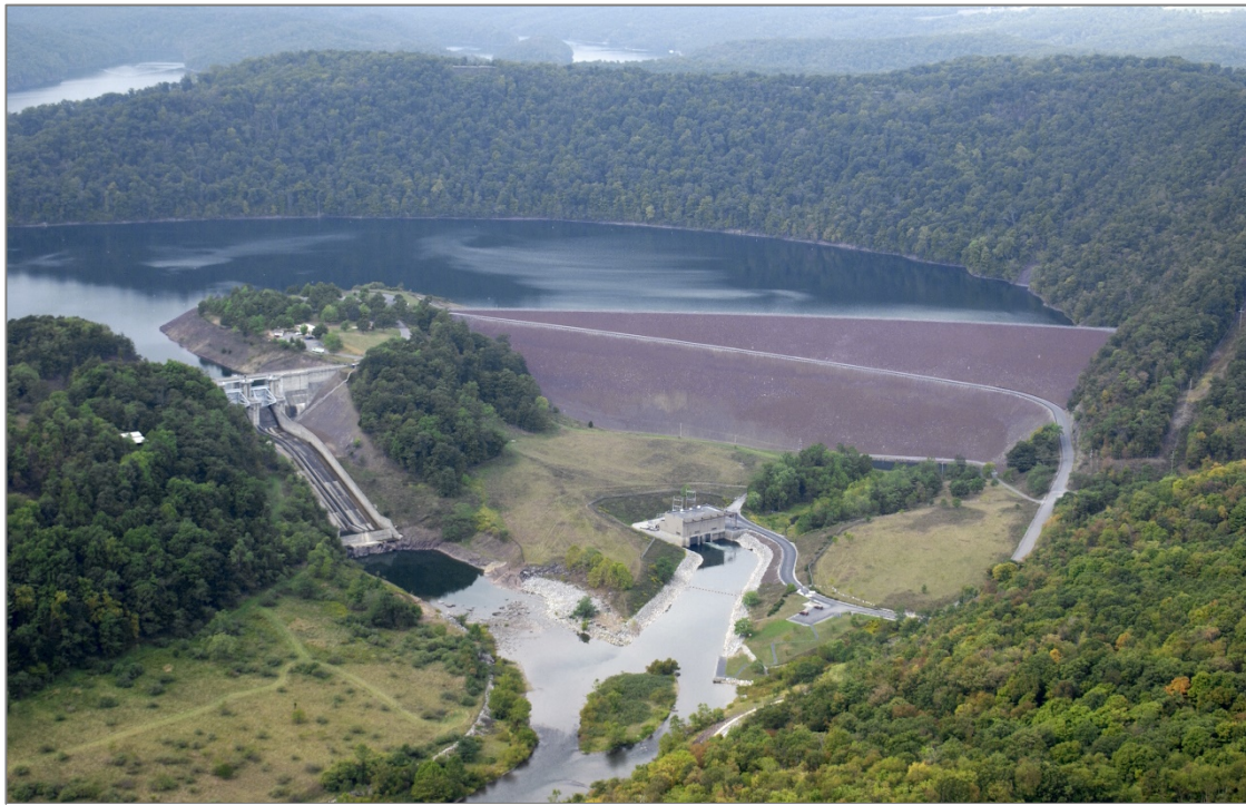
Figure 1.1 View of the Ravstown Dam and Outlet Works.
