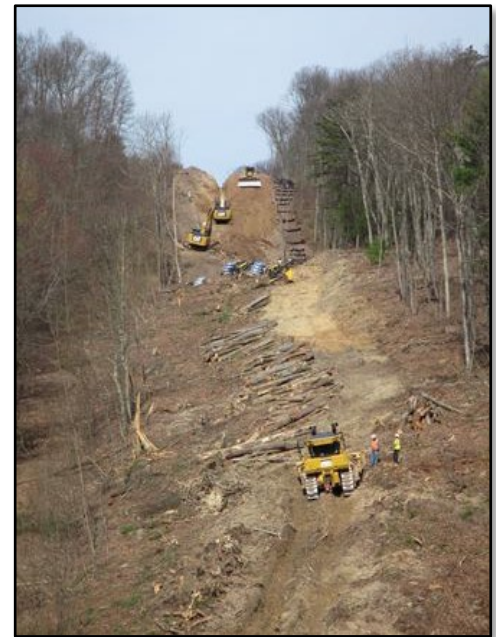
Figure 2.10 Construction of the Mariner 2 Pipeline on the Raystown Lake Project.
