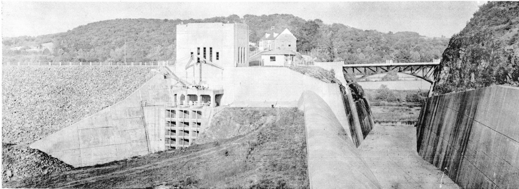
INDIAN ROCK DAM AND SPILLWAY. A portion of the rock-faced dam can be seen at the left. The control house is shown at the center. Flow in the creek normally enters the three gated openings under the control house and is carried through a 15-foot tunnel to the creek channel downstream. The operator's residence appears just to the right of the control house. The concrete spillway (foreground) would be used only in the event of a flood that exceeds the reservoir capacity. Note 3-hinged steel arch bridge which carries road across spillway channel.
