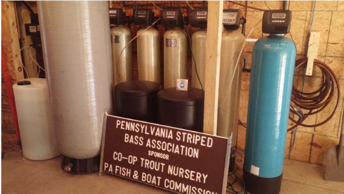
Water Purification Tanks to Condition Artesian Well Water for Hatchery
