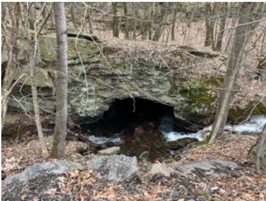
Exhibit 2- Photo from site visit on 3 April 2026 of Trib 28570 disappearing into an underground mine.
