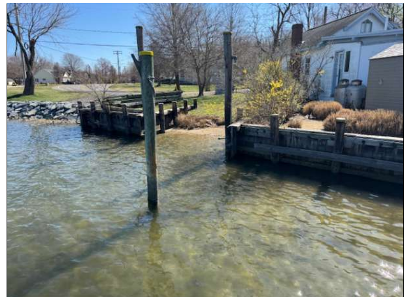
EXISTING BOAT RAMP PHOTO
