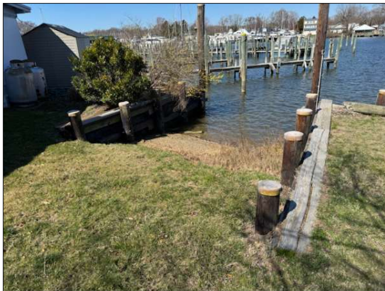
EXISTING BOAT RAMP PHOTO
