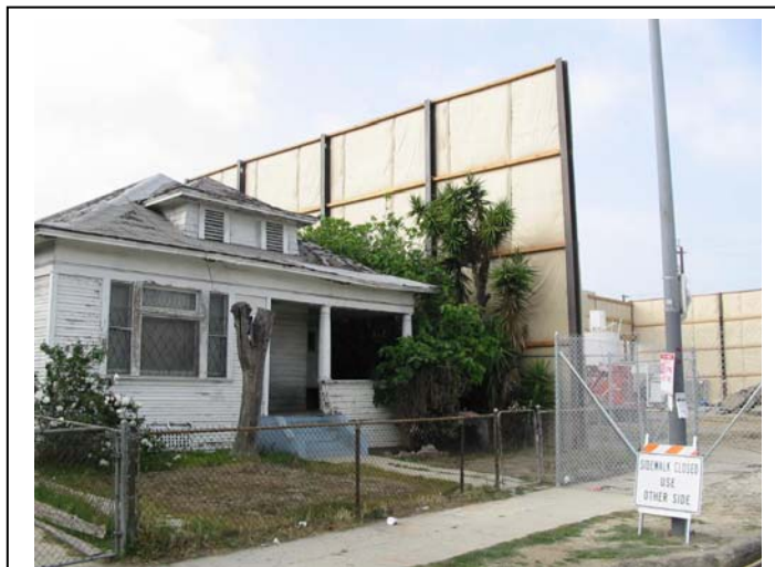
Figure 5 – Soundwall Made of Acoustical Curtain
