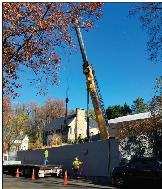
Crews utilize the crane on its first day at the Glenbrook Road project site to lift some of the crane's own equipment and extension parts that arrived by flatbed truck. The small crane is essential for lifting and relocating the ECS and heavy support equipment, in preparation for the third and final phase of high-probability removal operations.
