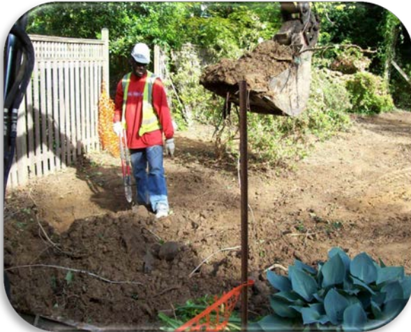
Exhibit 4-4. During Grid Excavation
