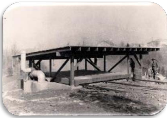
Exhibit 1-4. Bunker with Roof on Rollers
