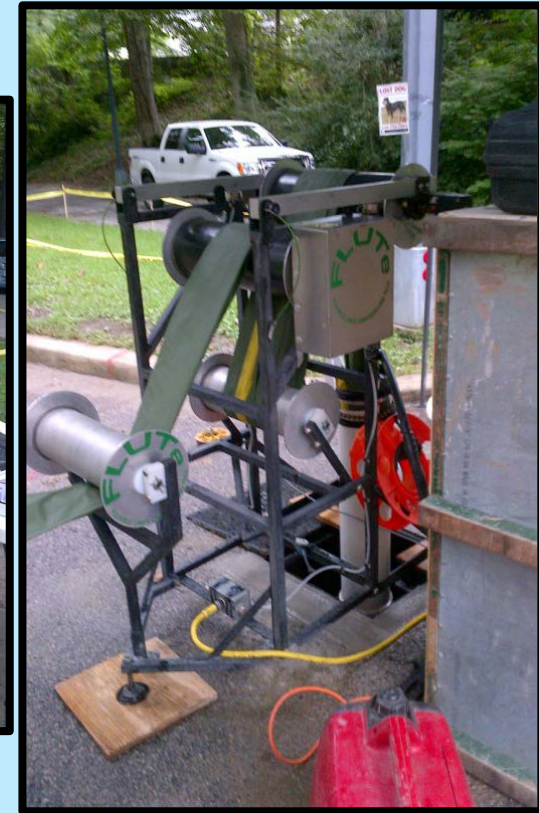
Installing the liner to seal bore hole wall
