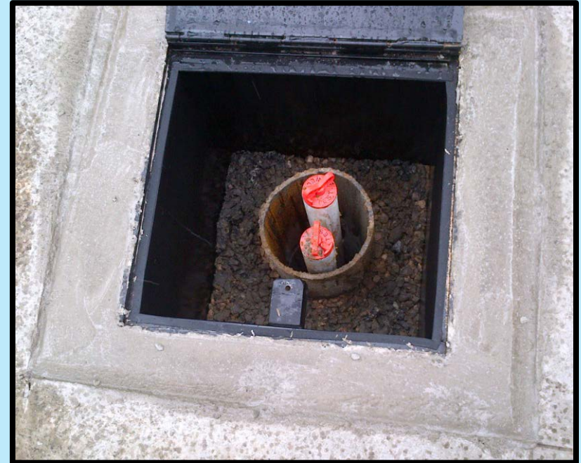
Completed Well at Sibley Hospital (MW-46 S&D)
