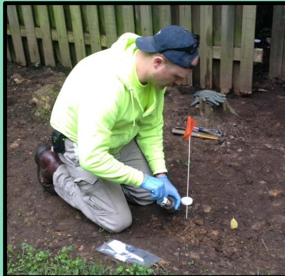
Using a Schoenstat to clear the area for anomalies
