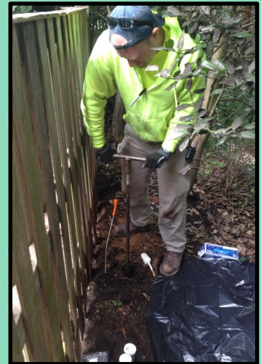
Hand augering for subsurface sampling
