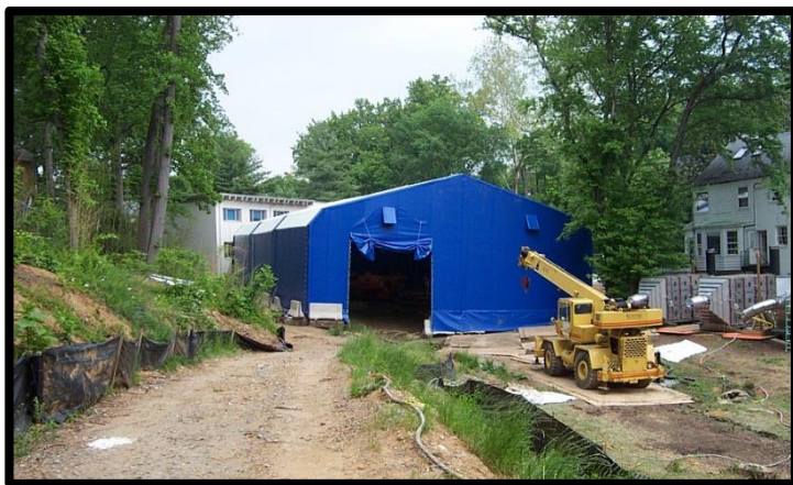
Engineering Control Structure Tent at Lot 18
