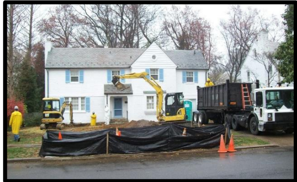
Arsenic Contaminated Soil Excavation
