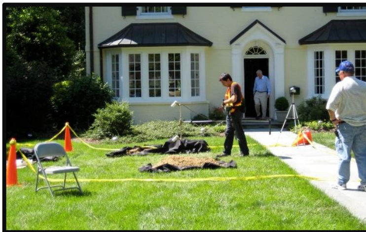
Intrusive Investigation of Anomalies
