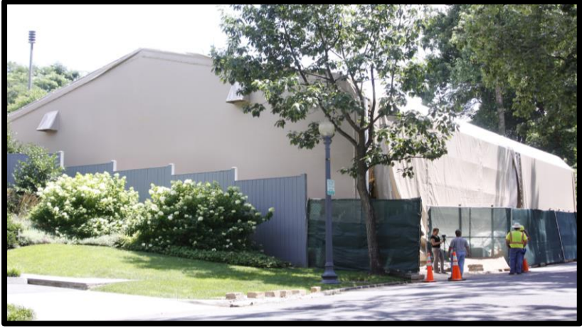
Engineering Control Structure over Excavation Site at 4825 Glenbrook Road NW
