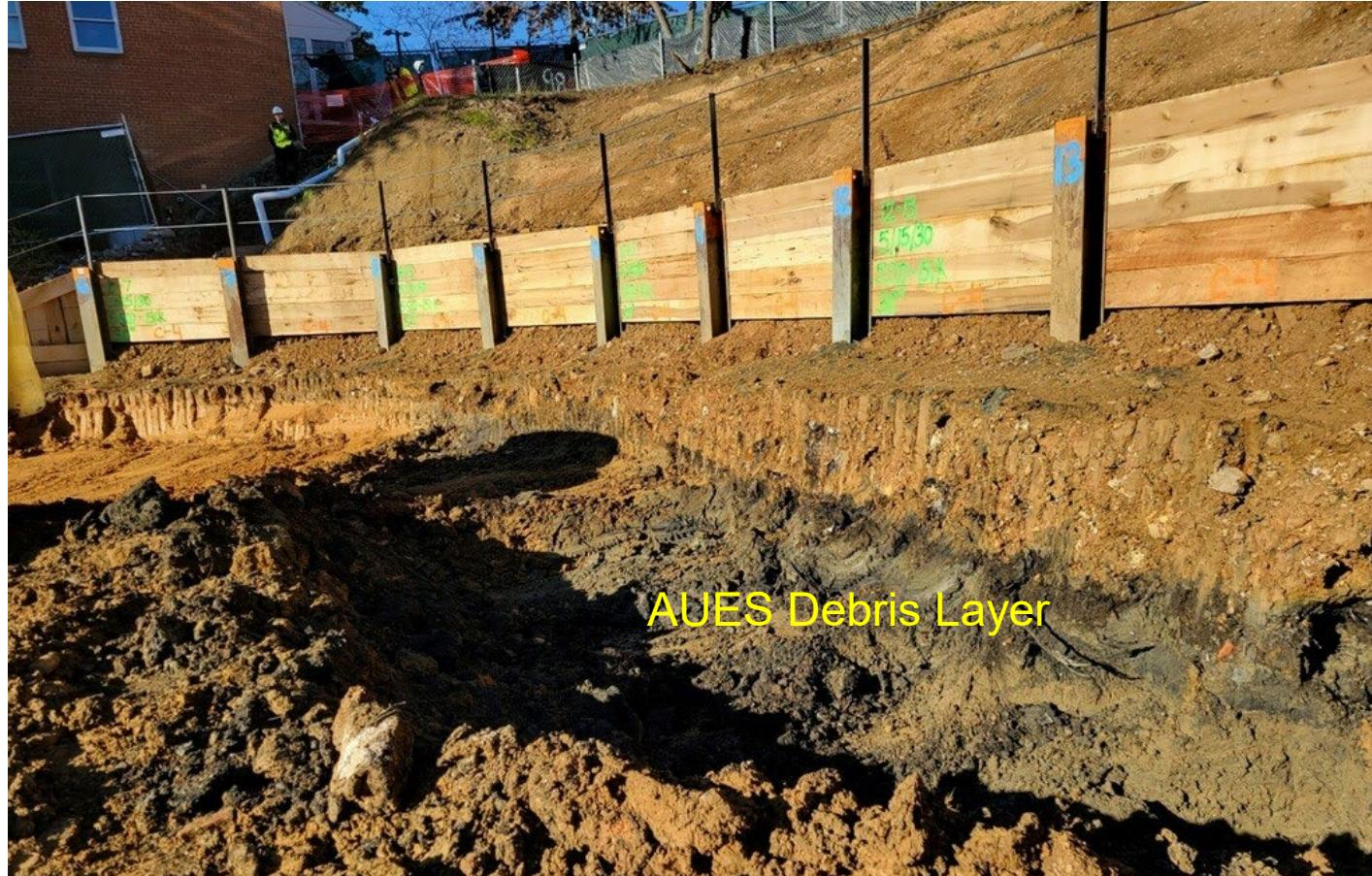
Dark Stained Soil and Glassware (see adjacent photo) Indicative of AUES Debris was First Encountered Excavating Soil at Elevation 355 ft, approximately 7 ft below the top of the Retaining Wall and extended down to Elevation 347 ft. The AUES layer was 7-8 ft thick between Piles 14 and 15.
