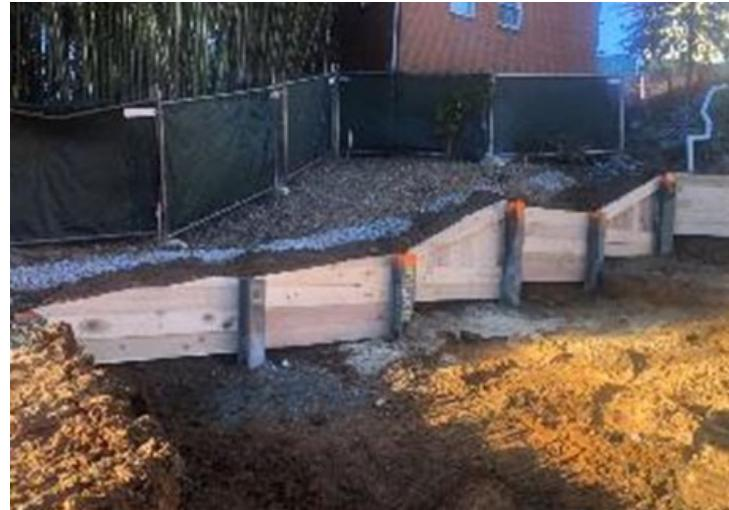
Wood Lagging Installed between the H Piles on the Western wing of Wall
