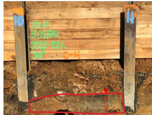
Sidewall at Piles 10 & 11. Dark AUES layer at wall, 1 ft 7 in thick
