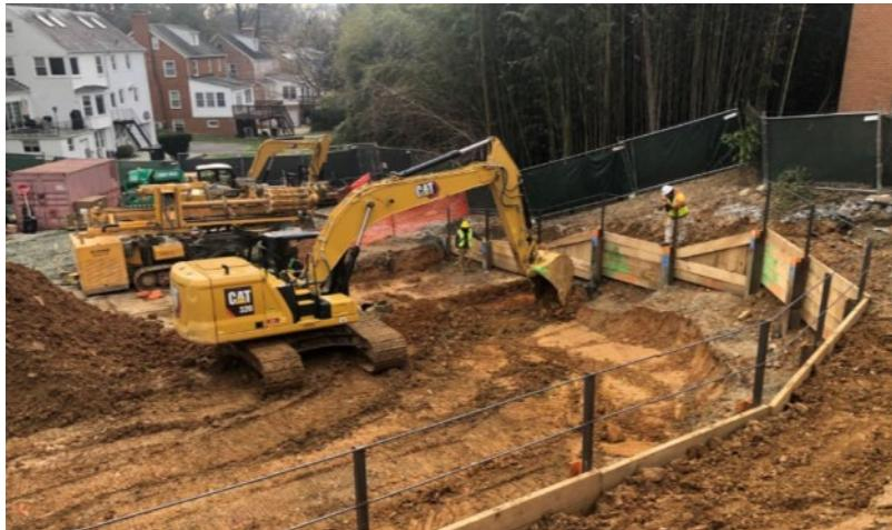
Excavation in progress along the west end of the retaining wall for the second tier of lagging
