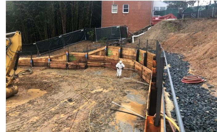
Berkel pumping grout into tieback between H piles 8 and 9.
