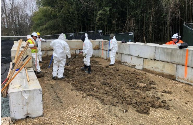
UXO Team screening soil on AUES Debris sorting pad with a metal detector
