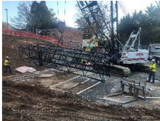
Breaking down the Crane and Auger components for Demobilization
