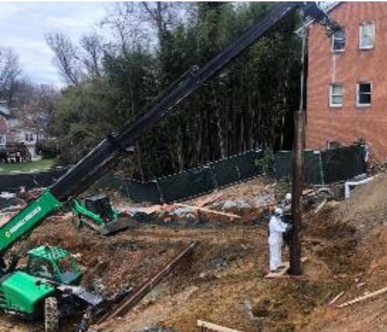
Lifting & Setting H Pile #14 in the Auger hole
