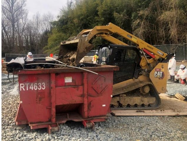
Skid steer dumping processed AUES soil into roll-off container.
