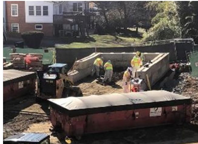
UXO Team screening soil on AUES Debris sorting pad with rakes/hoes
