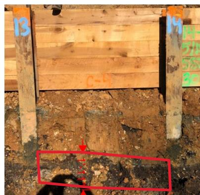
Sidewall at Piles 13 & 14. Dark AUES layer at wall, 1 ft 11 in thick
