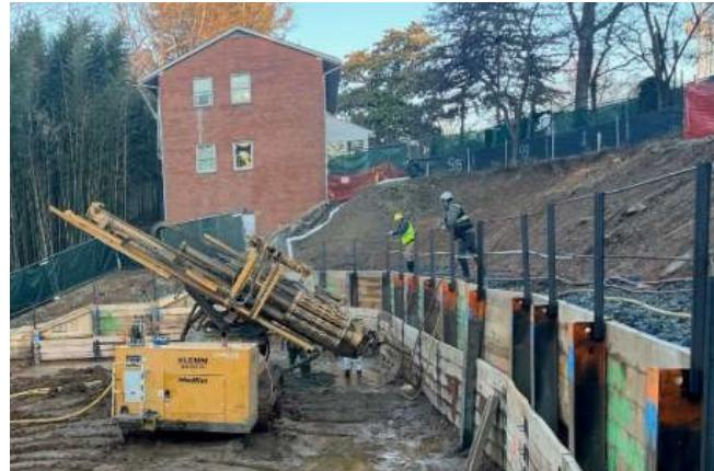
Berkel starting initial tieback installation at location between H piles 12 and 13.
