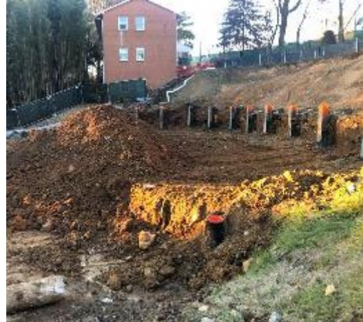
First soil bench completed on the north wall – ready for Laging
