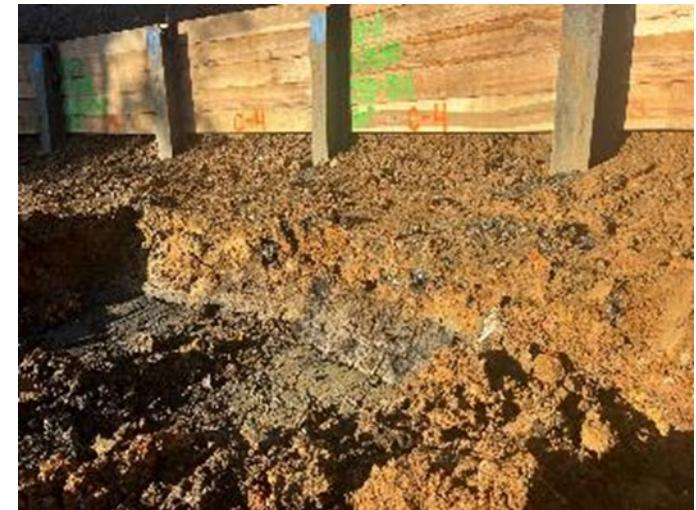
First Encounter of dark AUES Debris layer in second cut at H Piles #9 and #10
