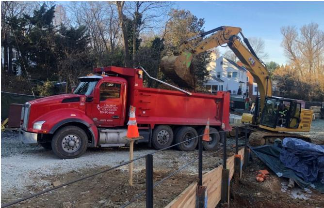
Clean overburden material being loaded into dump truck for transport to the soil storage area at the Federal Compound.
