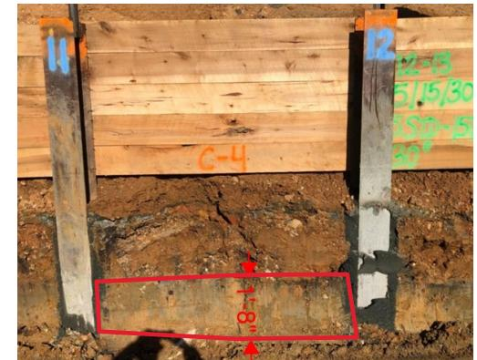
Sidewall at Piles 11 & 12. Dark AUES layer at wall, 1 ft 8 in thick
