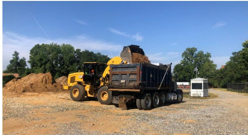
Loader placing clean overburden fill material into dump truck for transportation to PSB.
