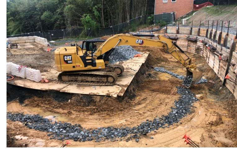
Excavator placing stone at the start of excavation backfill operations.
