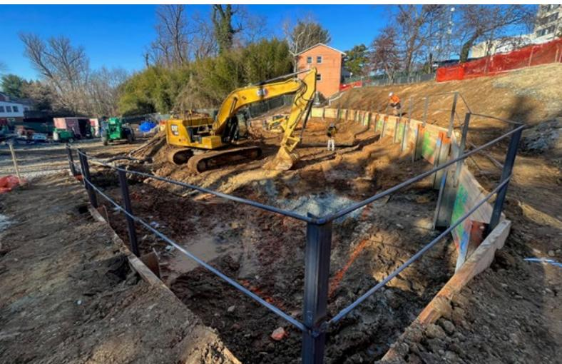
Overview of the First 5 Feet of Completed Retaining Wall
