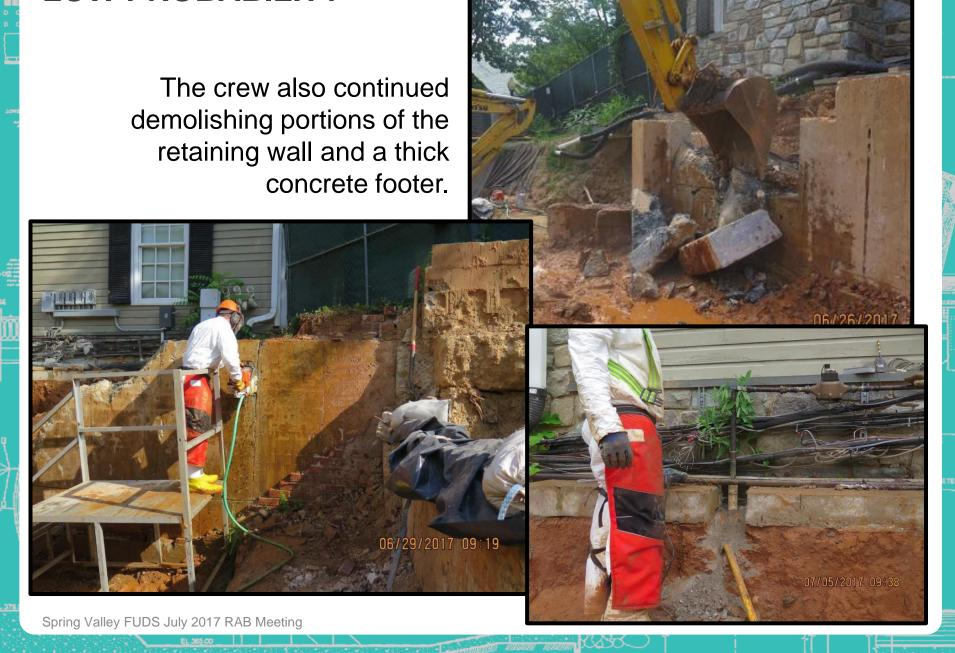
Rubble from the demolished retaining wall where CACM or AUES debris was recovered, is broken into small pieces so it can also be placed into drums for disposal.
