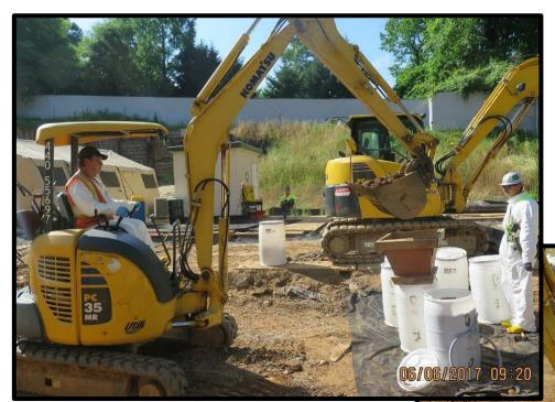
Potentially contaminated soil continues to be sifted and placed into drums for disposal.
