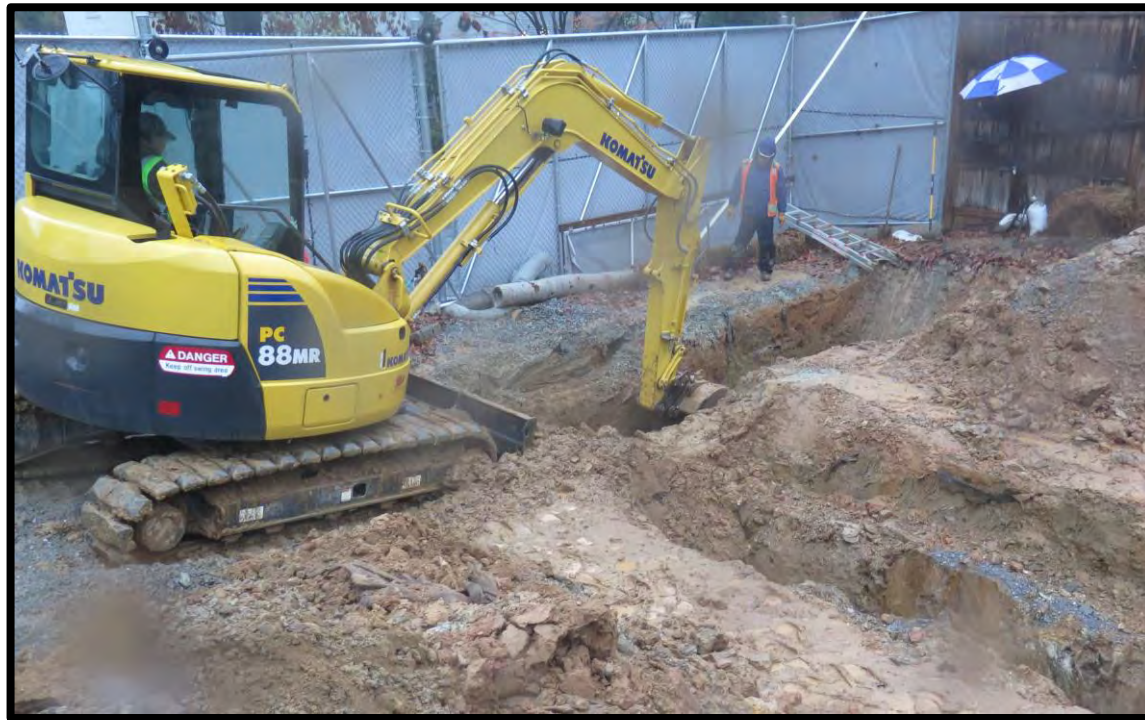
Digging sewer line trenches
