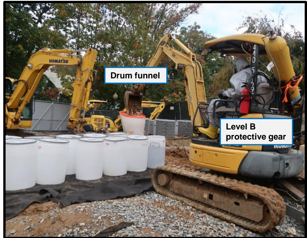
Crew working in Level B gear using a mini-excavator to load soil into drums with a drum funnel
