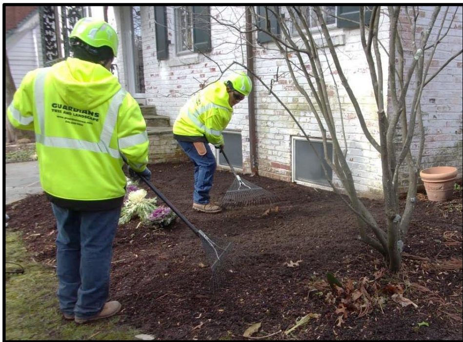
Landscape removal team leveling area where vegetation was removed.
