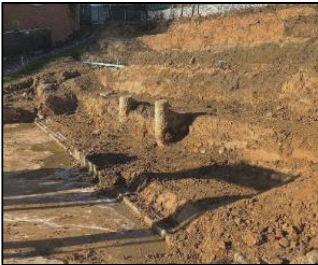
Completed upslope stabilization benches
