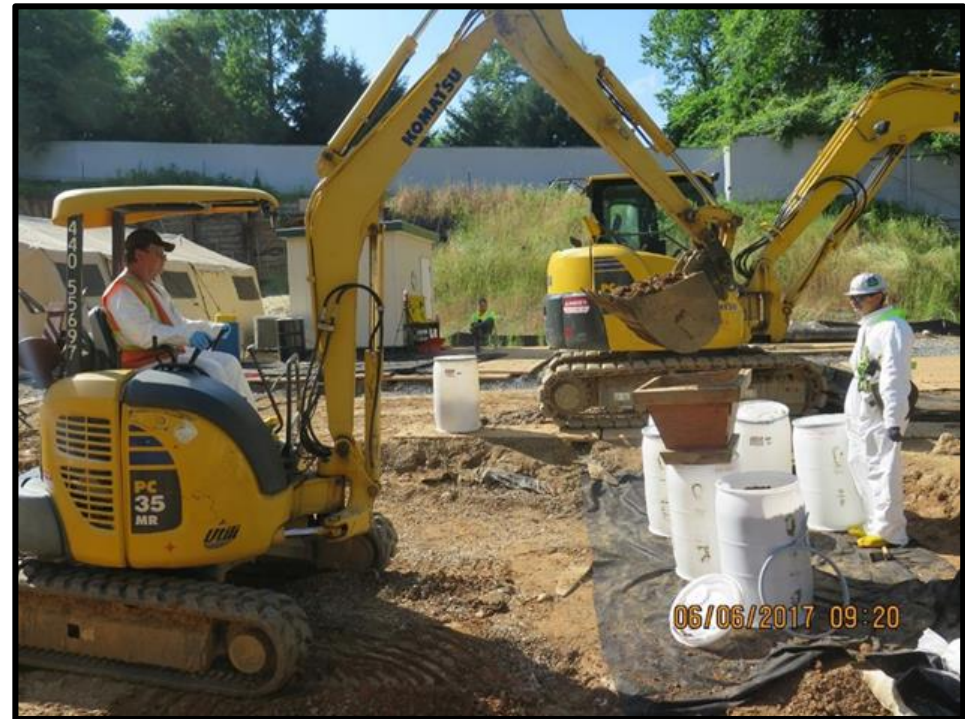
Mini-excavator placing soil into poly drums
