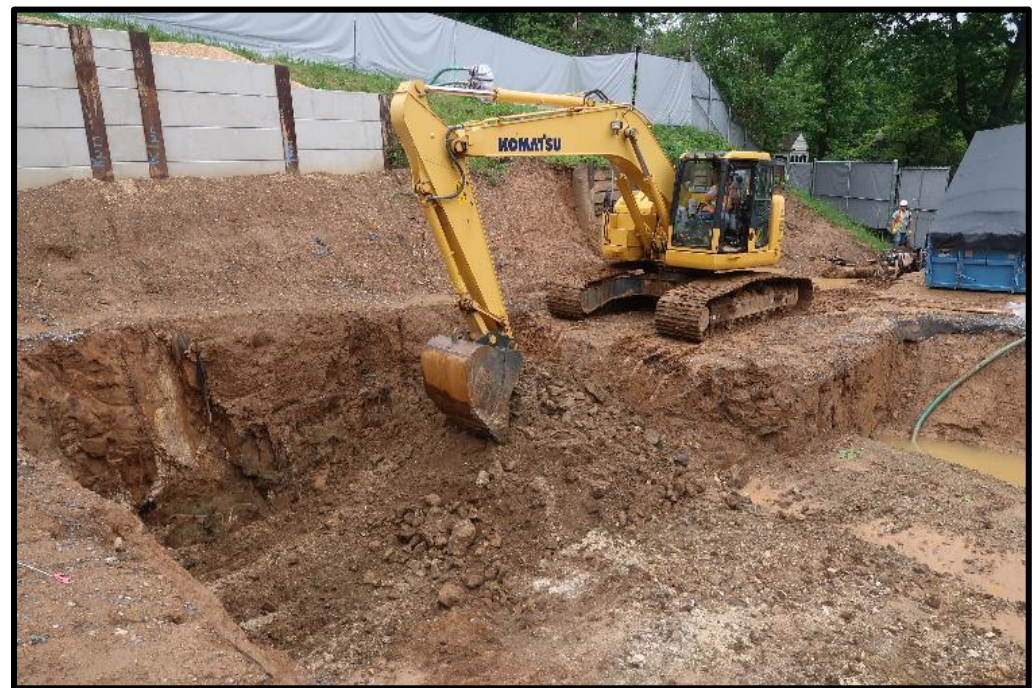
Backfilling grids with clean soil
