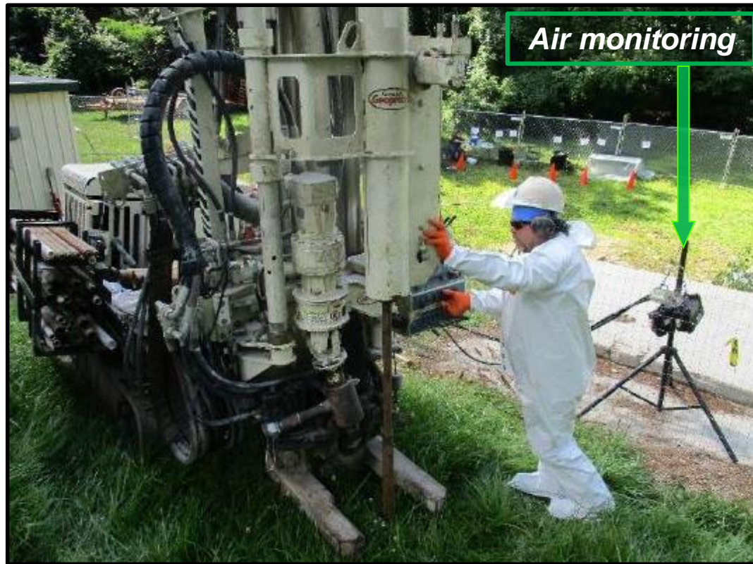
Geoprobe with auto-hammer operating geotechnical boring at AU's former Public Safety Building
