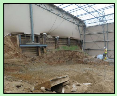
In mid-April, the crews began the final scraping away of the existing soil, and thereby exposing the saprolite or bedrock in the excavation area where the former basement floor was removed.
