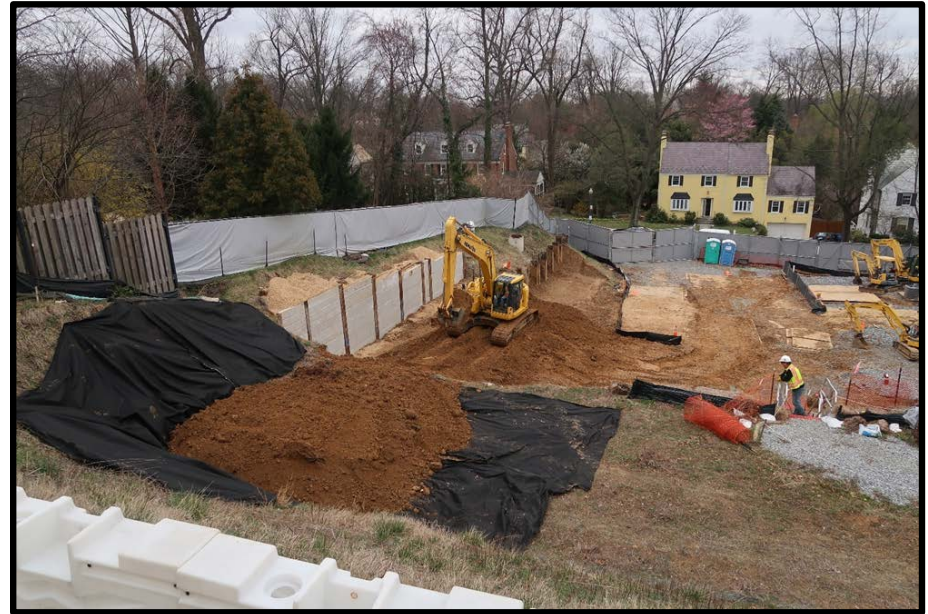
Removing clean top soil, to access some contamination noted at the saprolite level.
