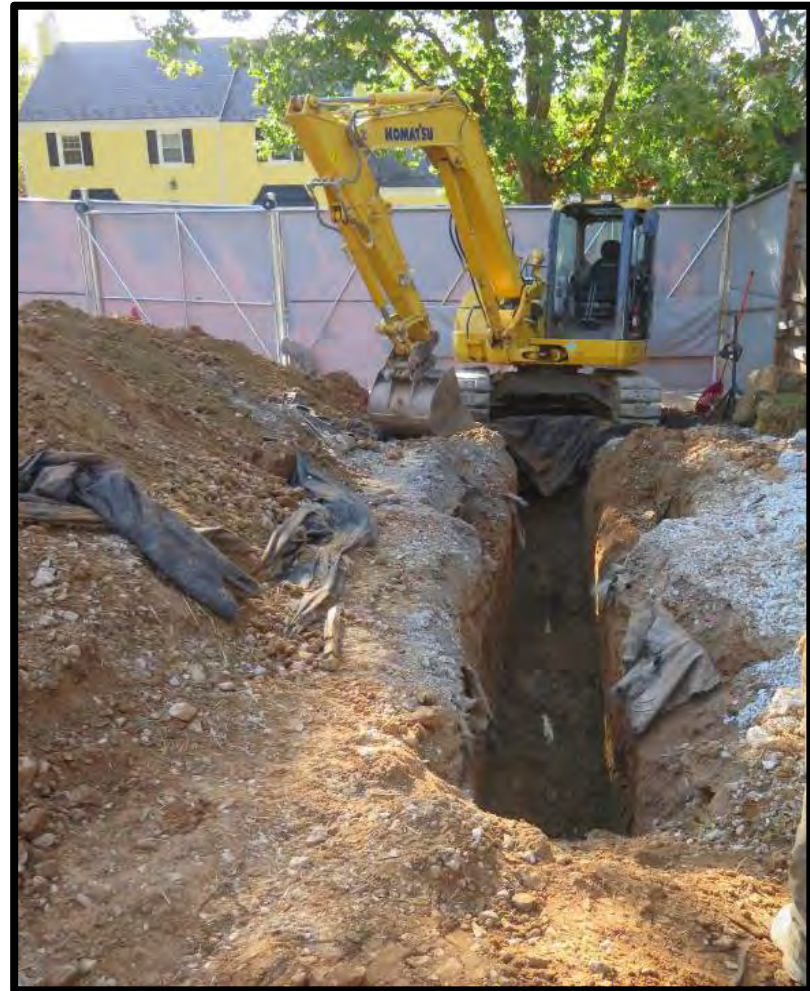
Trench to characterize existing sewer line
